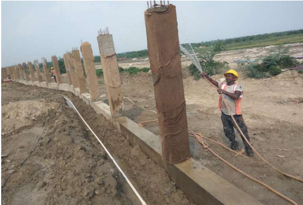
Funny bag wrapping and Curing of BW columns
