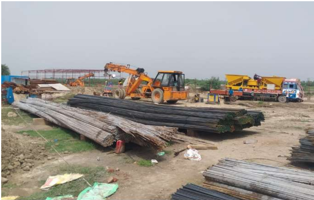
Unloading of steel
