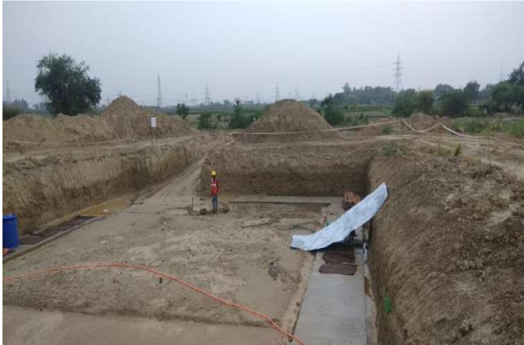
Ongoing Excavation work
