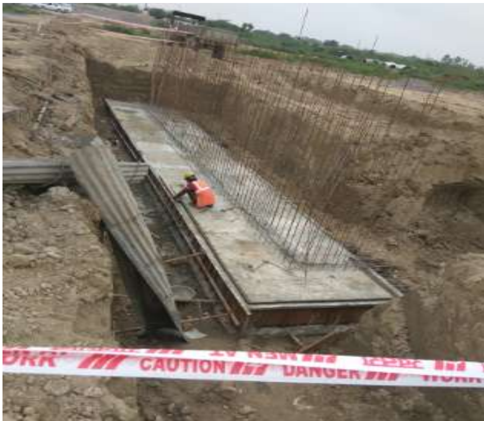
CCT Raft work
