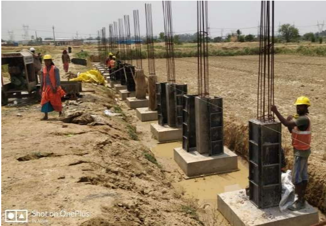
Boundary Wall work
