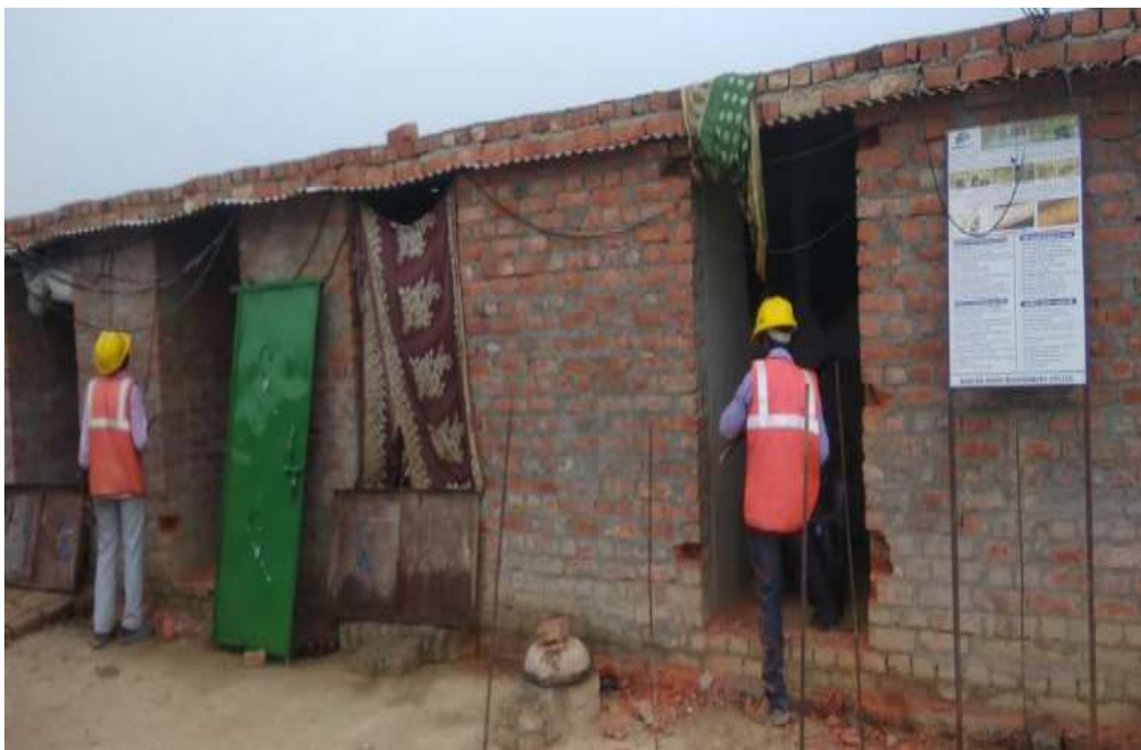
Ongoing work of Labour Kitchen
