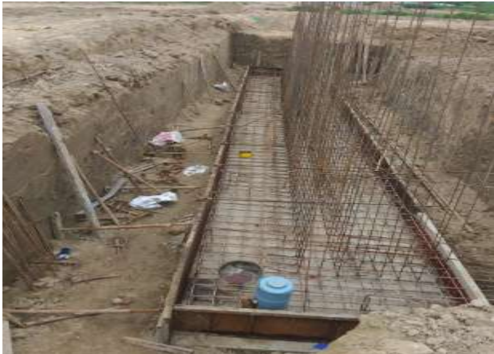
CCT wall foundation
