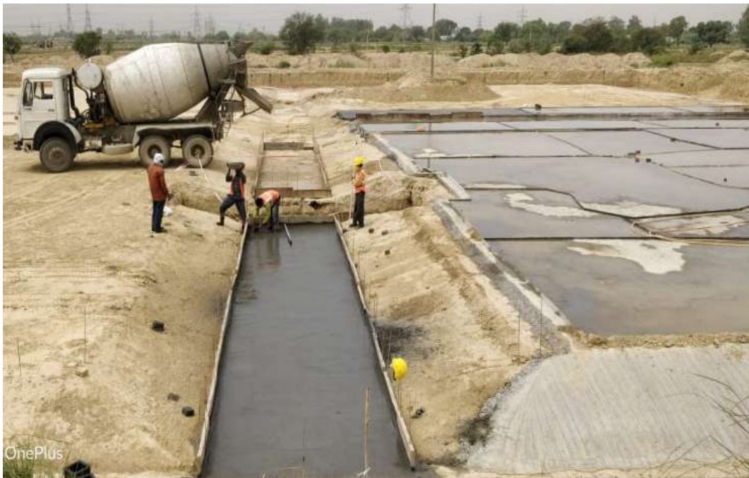
PCC work of SBR
