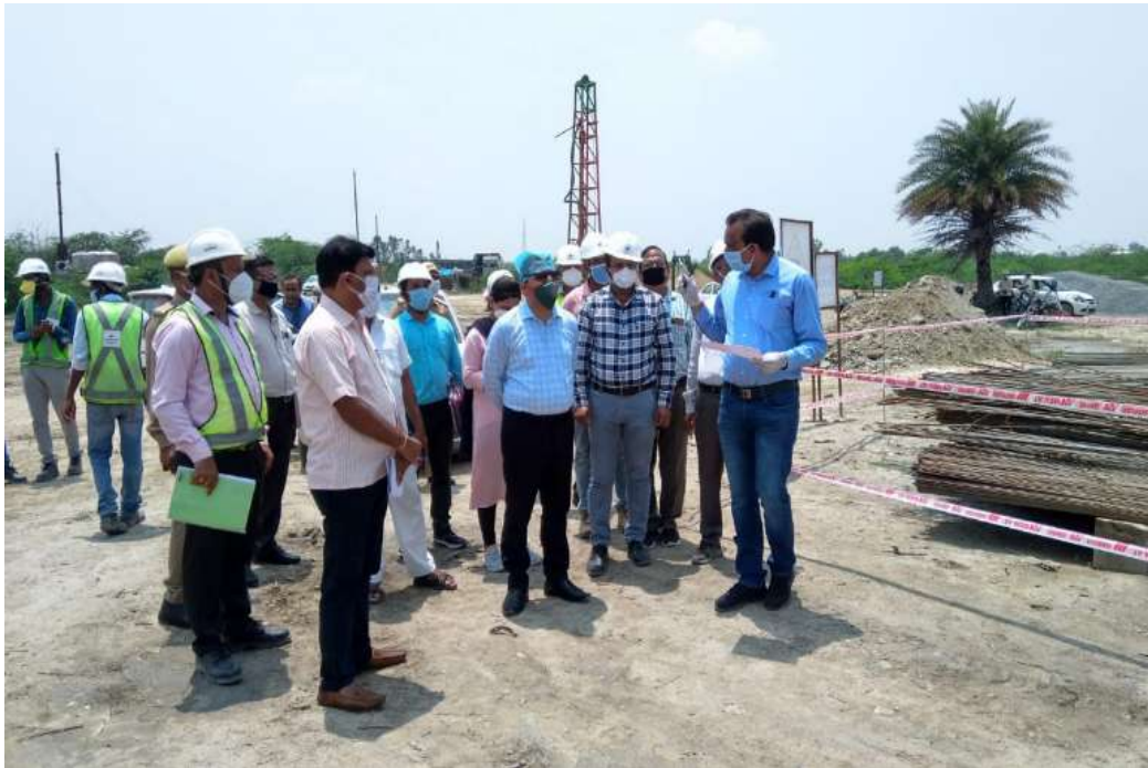
Site inspection by DM
