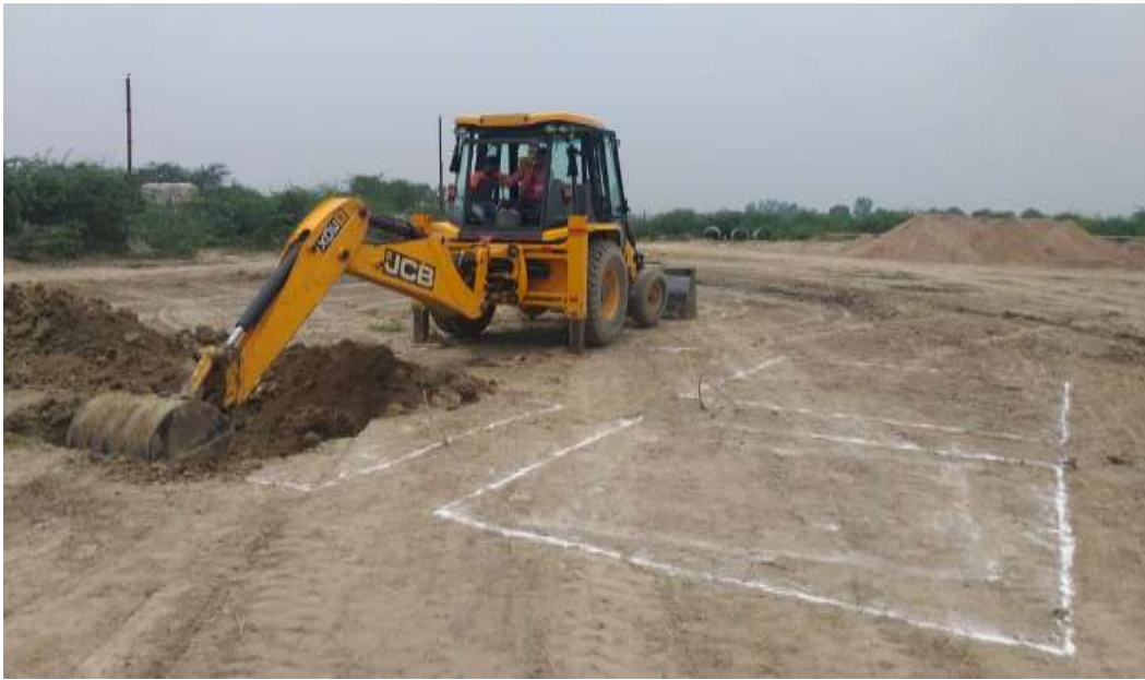
Guard Room excavation
