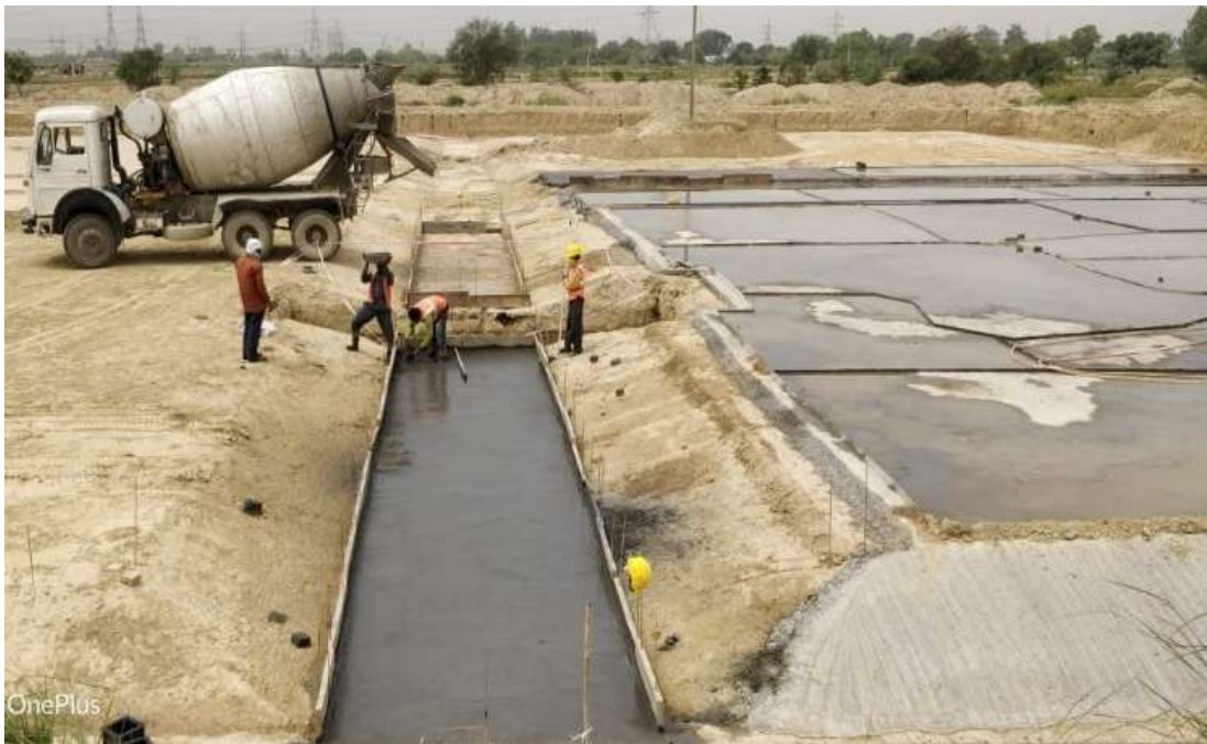
PCC work of SBR
