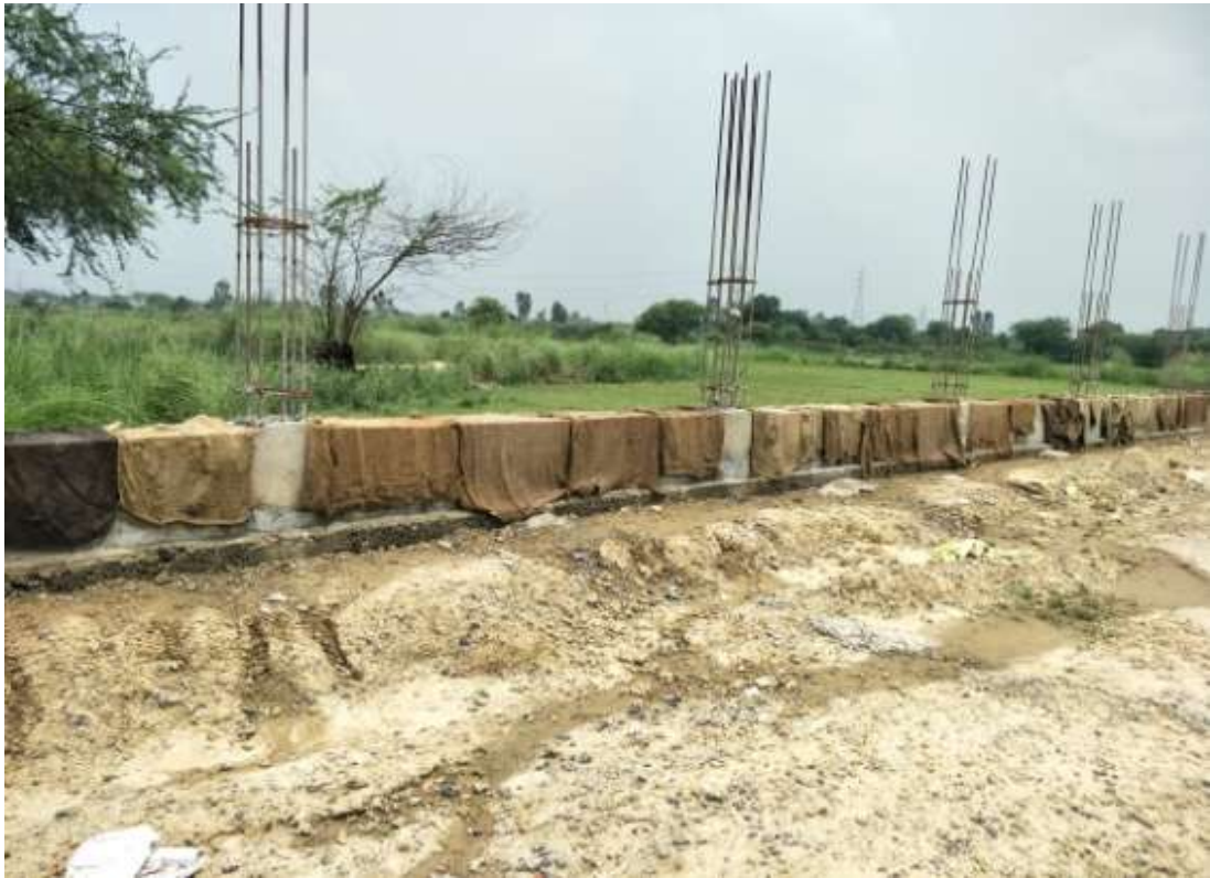
Plinth Beam Boundary Wall work
