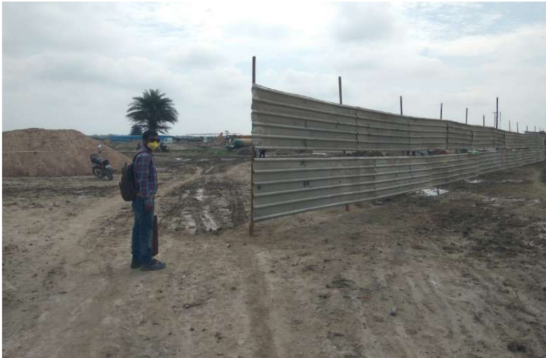
Hard Barricading in progress
