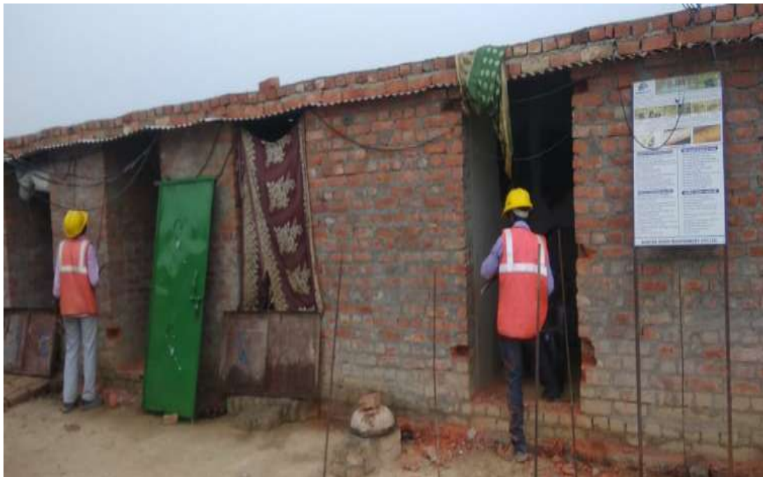
Ongoing work of Labour Kitchen
