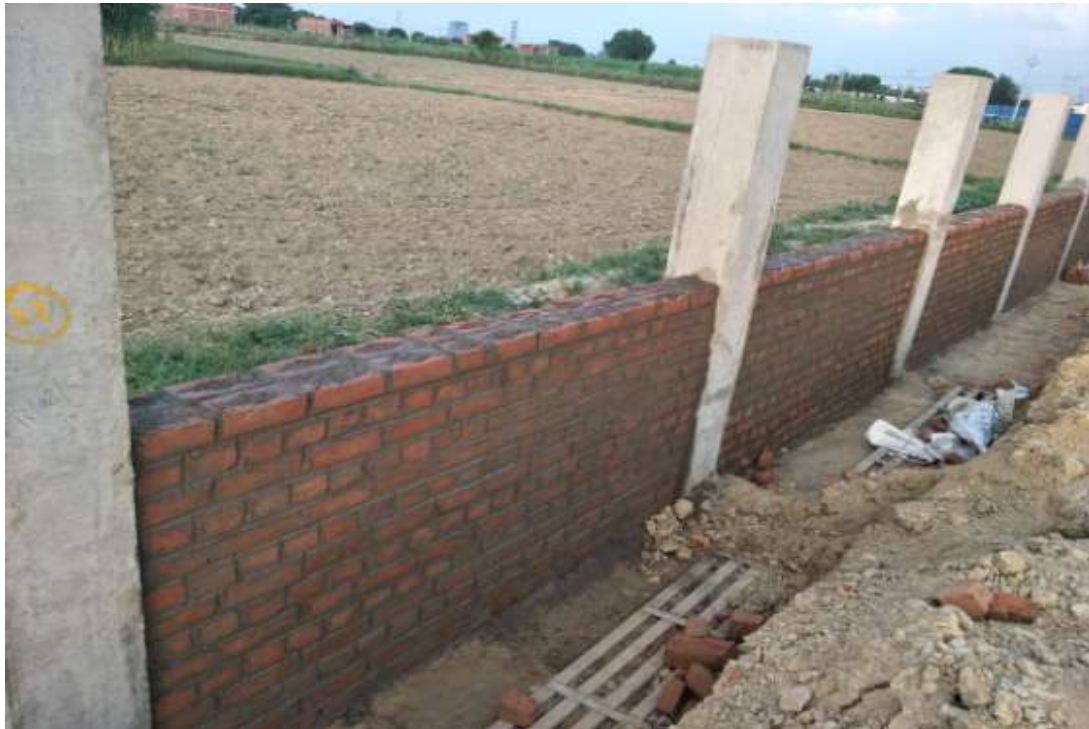
Boundary Wall Brick Work
