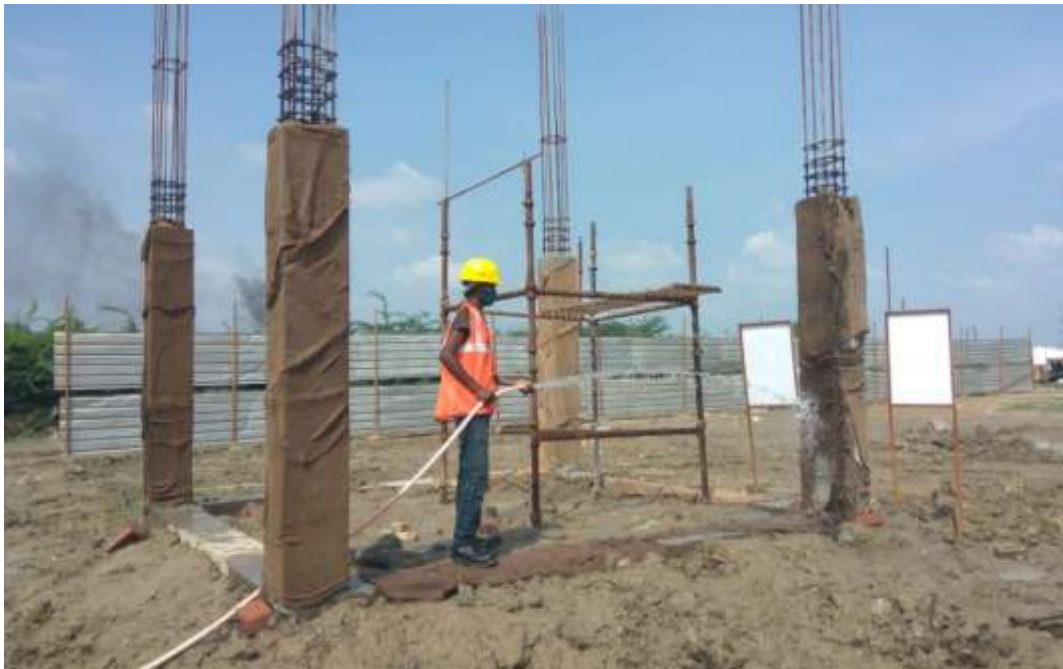
Curing at site
