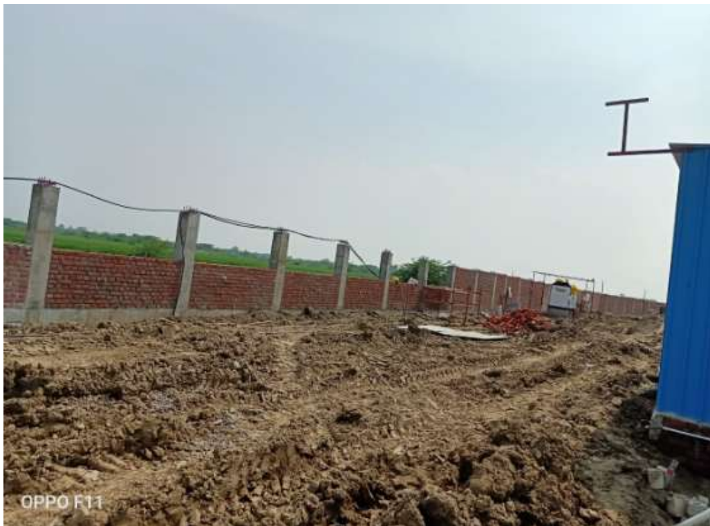
Brickwork of Boundary Wall
