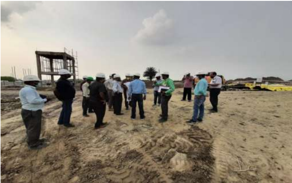
Site inspection by SMCG & SMEC
