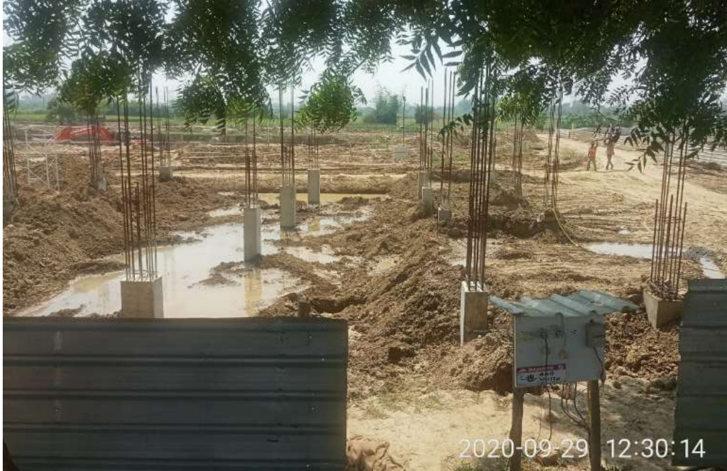
Admin building Excavation work
