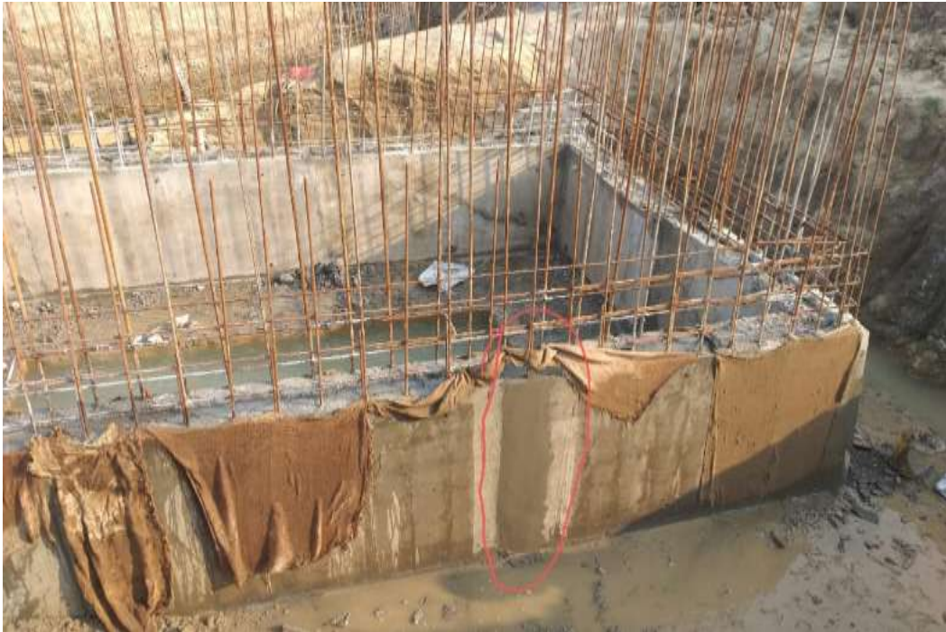
Supernatant sump wall correction & Funny bag wrapping and Curing
