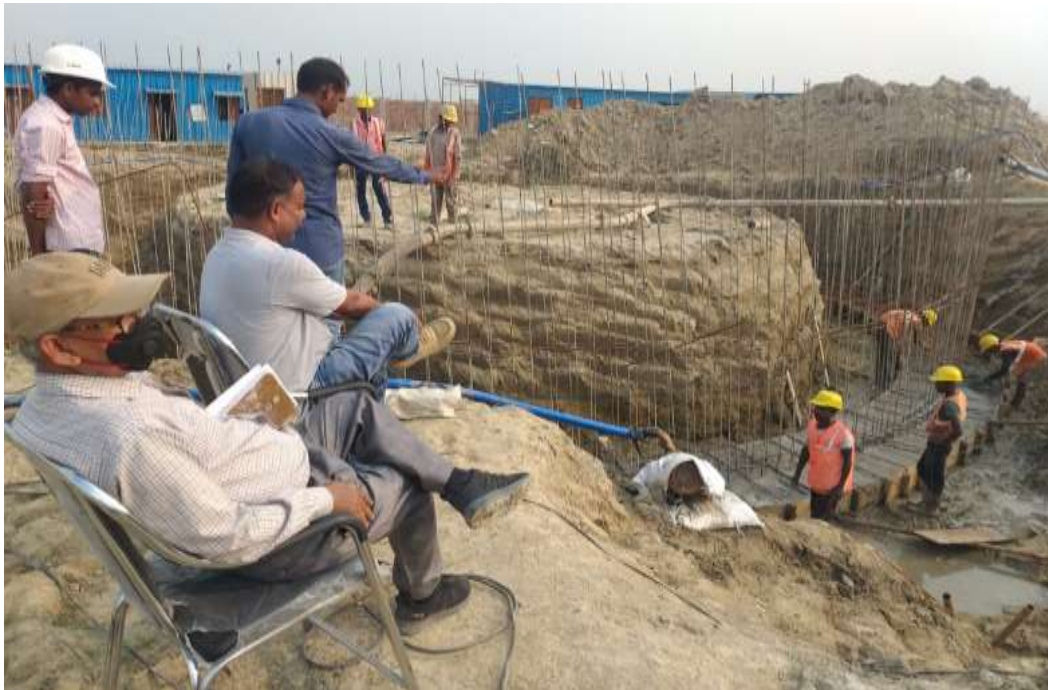
Concrete work of sludge thickener
