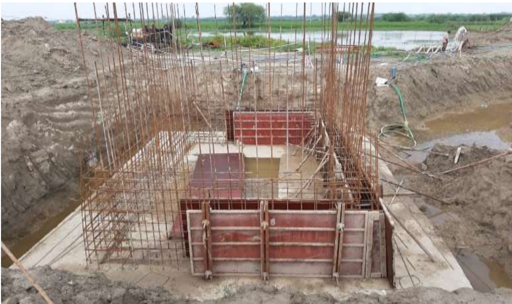
Concrete work of CCT
