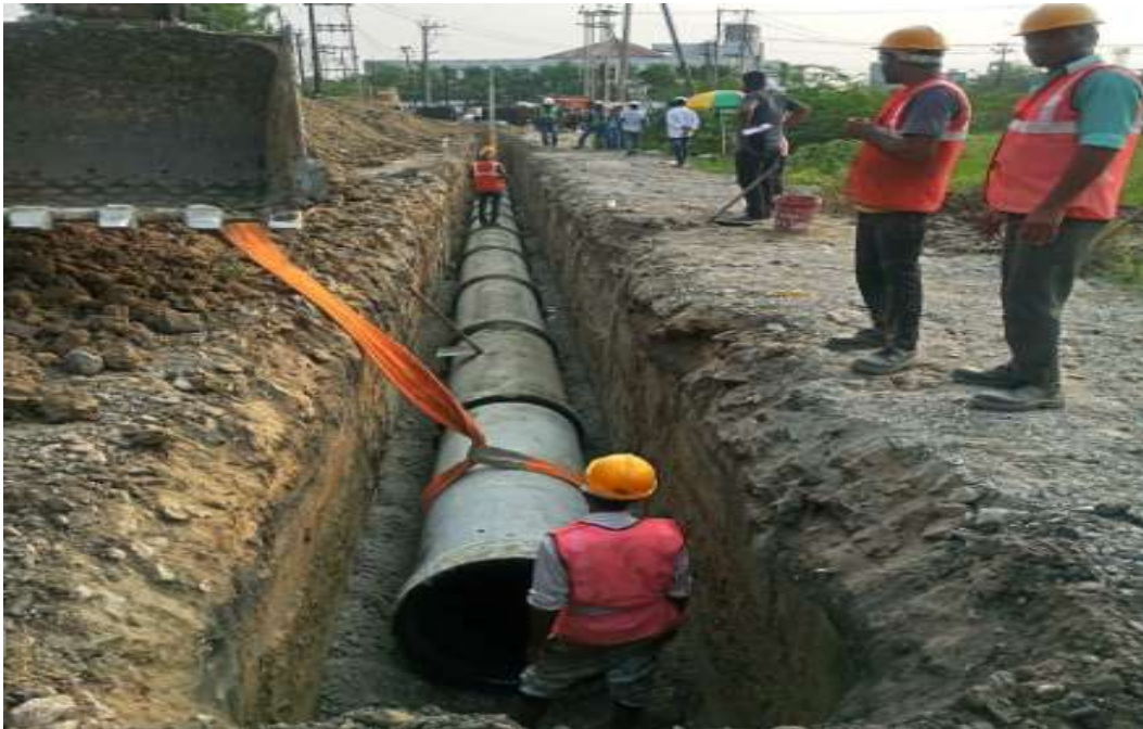
Ongoing work of RCC Pipe laying
