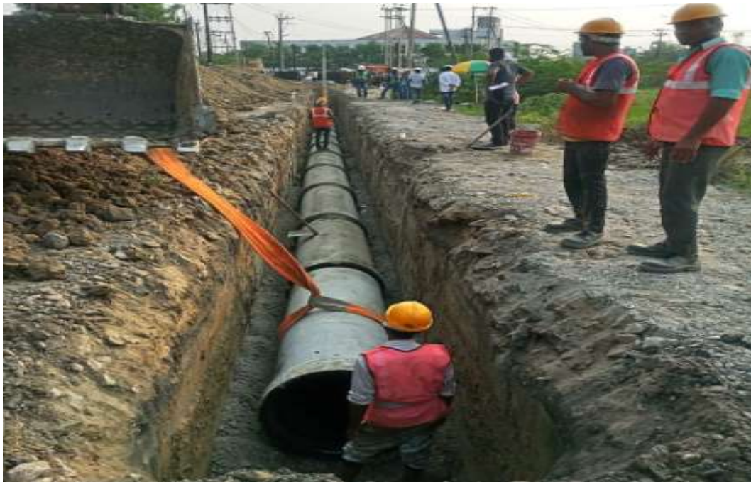
RCC Pipe Laying
