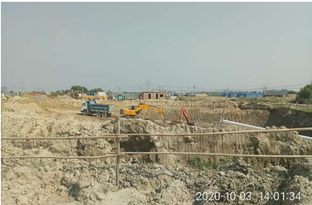
MPS Excavation work
