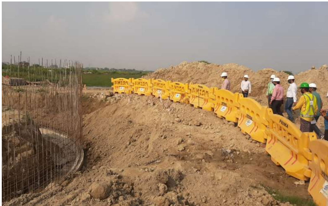
Hard Barricade around excavation
