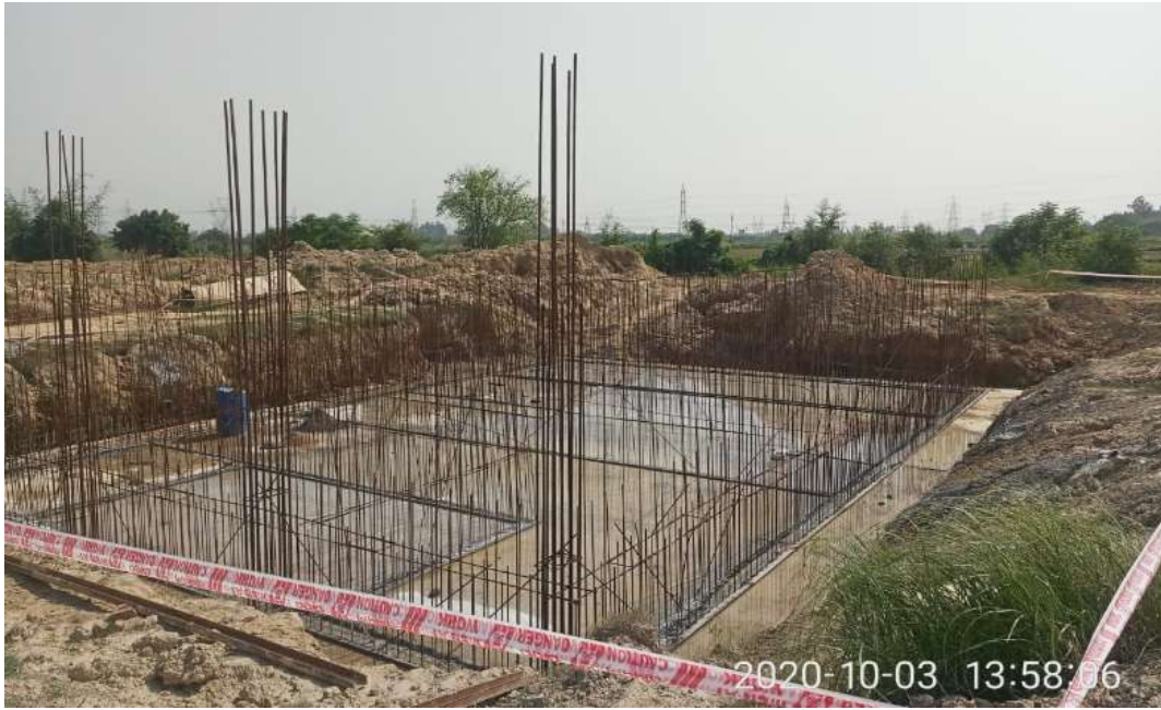
CCT steel binding works
