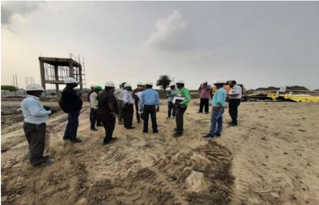
Site inspection by SMCG & SMEC on 01.10.2020
