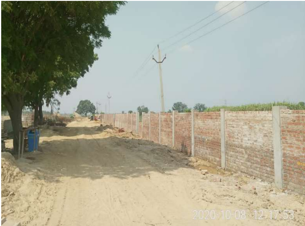
Boundary Wall work
