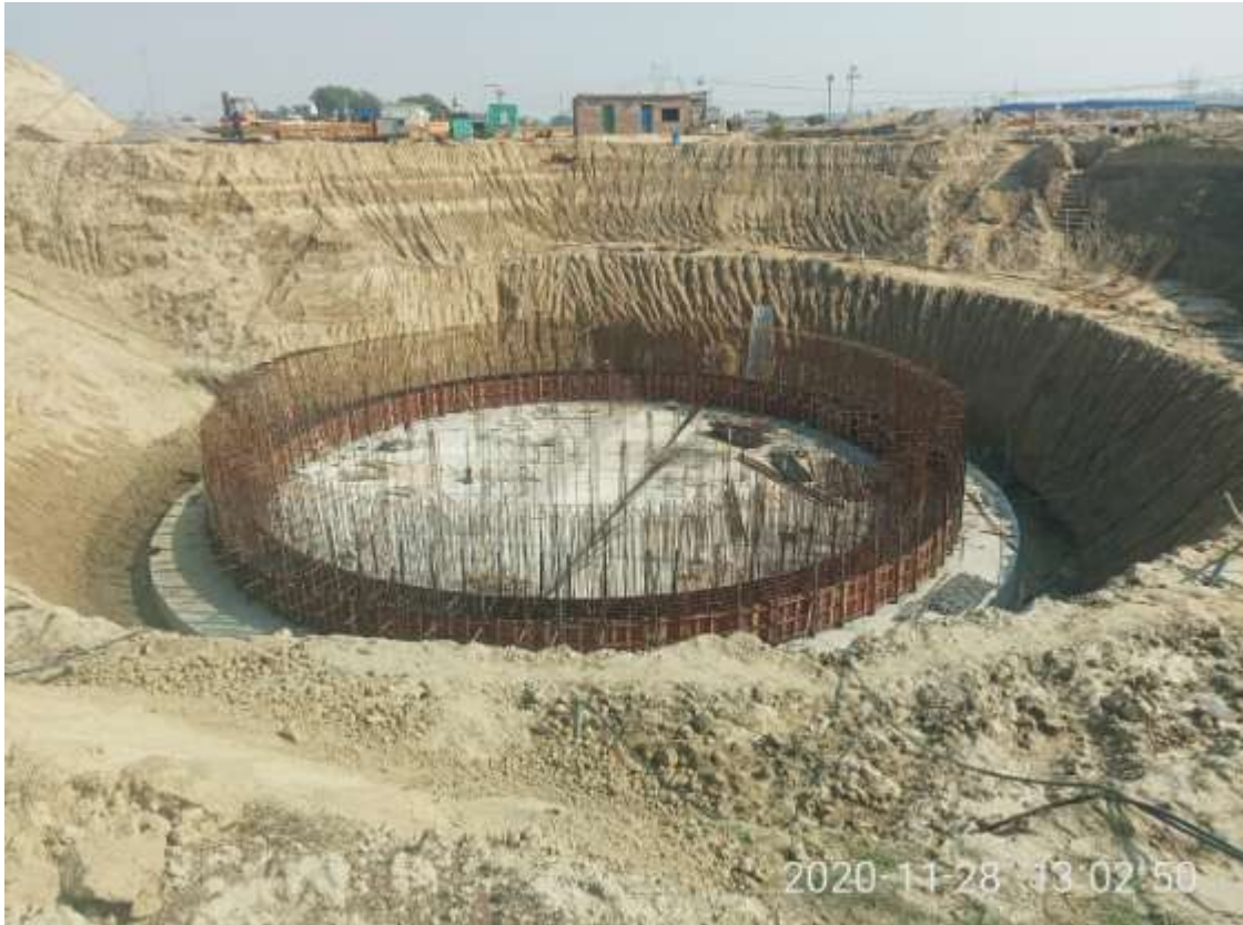
Ongoing works of MPS
