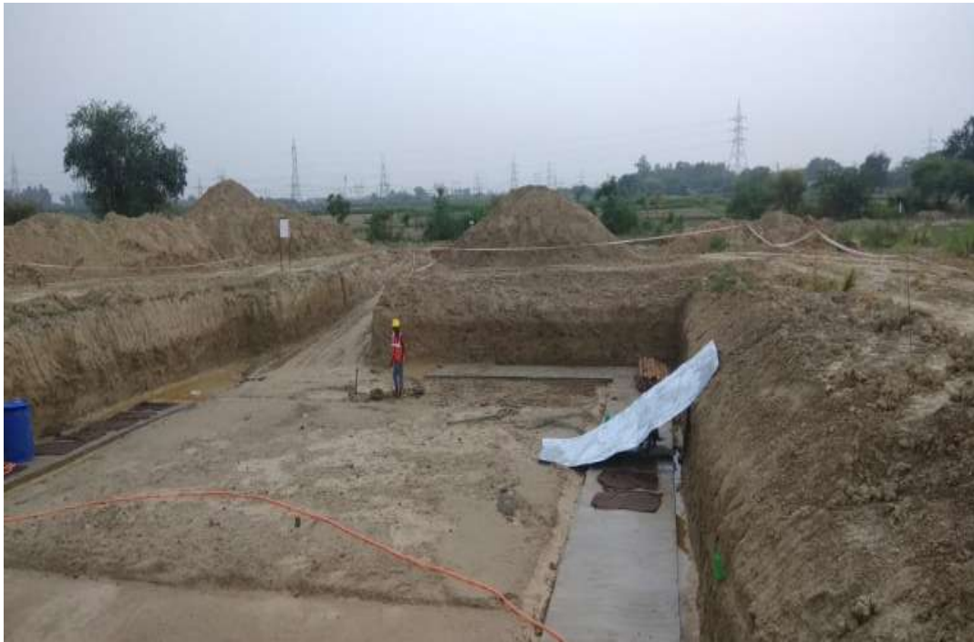
Ongoing Excavation work
