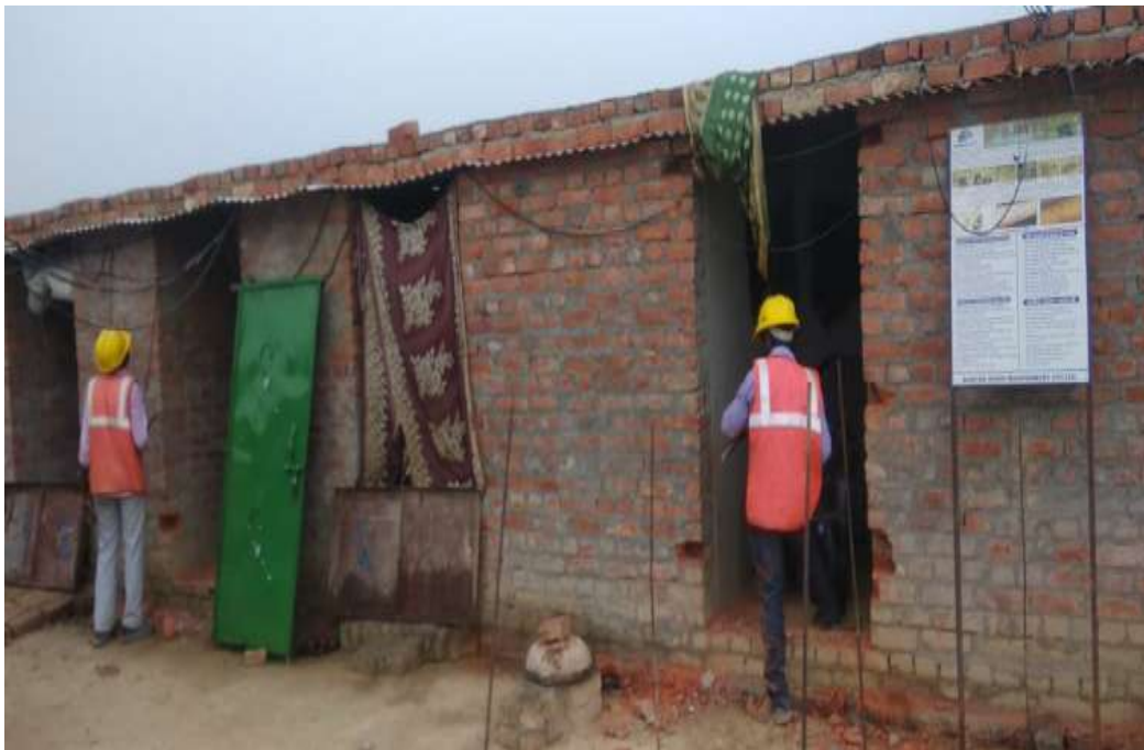
Ongoing work of Labour Kitchen
