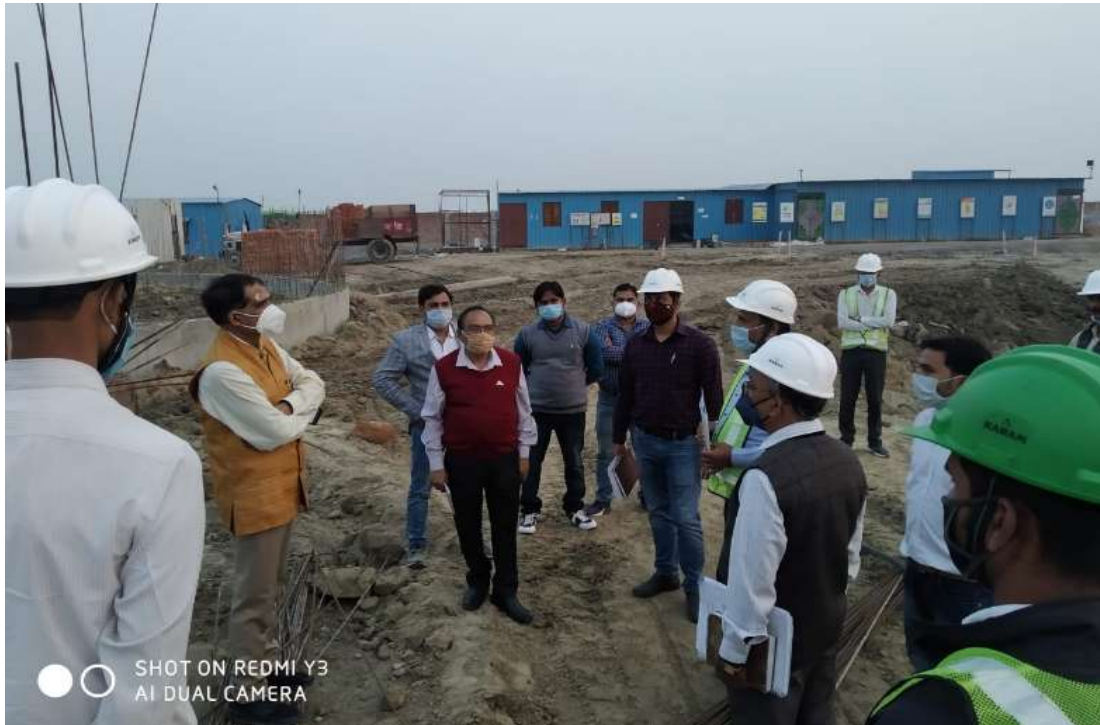
Inspection by CE, UPJN Lucknow on 19.11.2020
