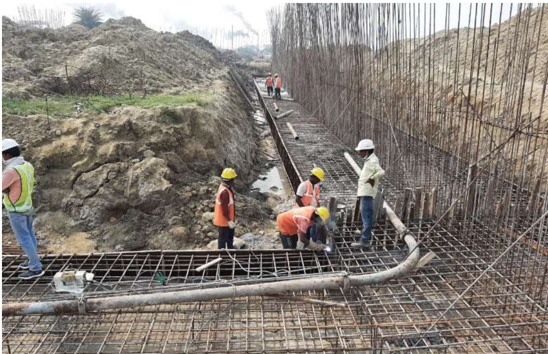
SBR Concrete work
