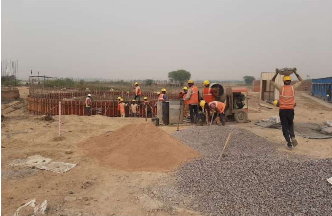
Ongoing work of Sludge Thickener
