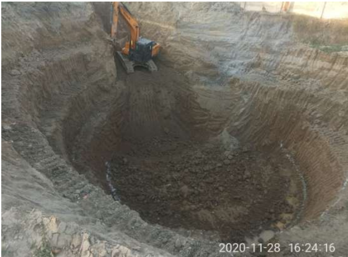
Sundar Nagar IPS excavation
