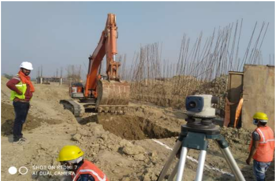
Excavation for 1200mm sewer laying work
