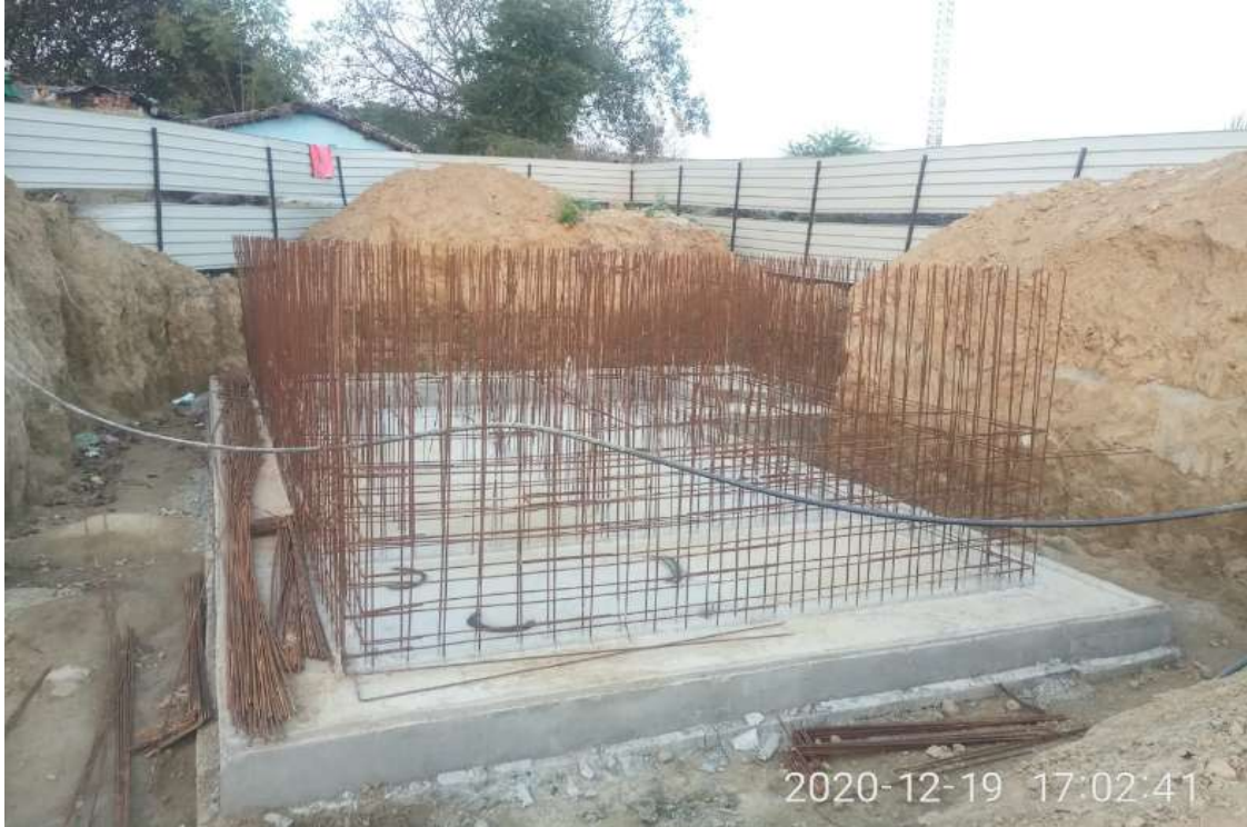
I&D work at ICI nalla
