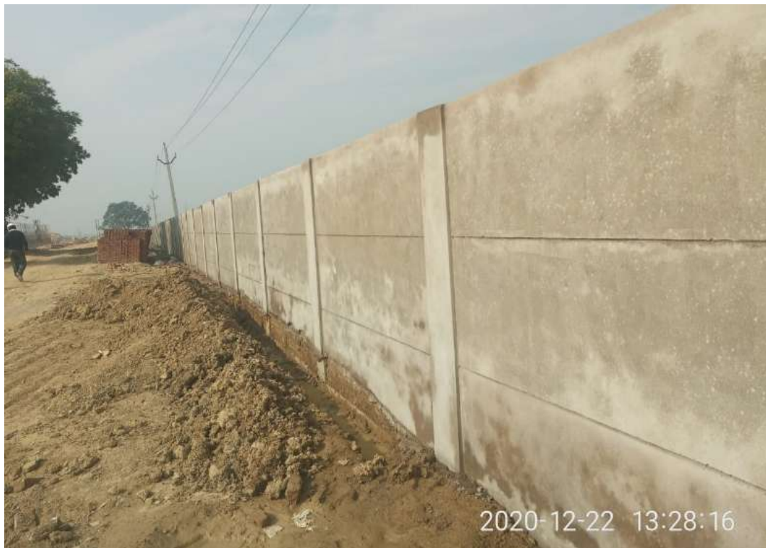
Boundary Wall work
