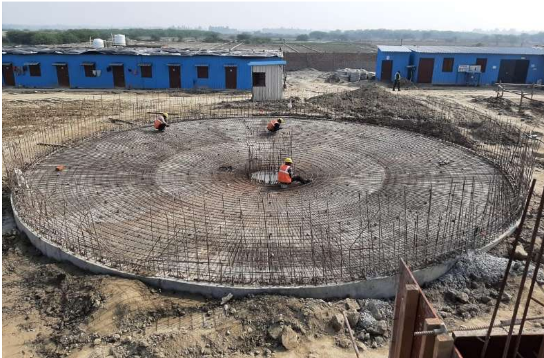
Supernatant Sump work
