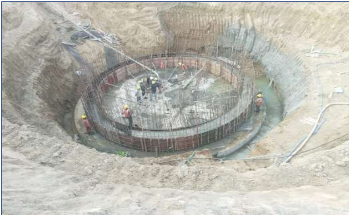
Sundar Nagar IPS wall casting
