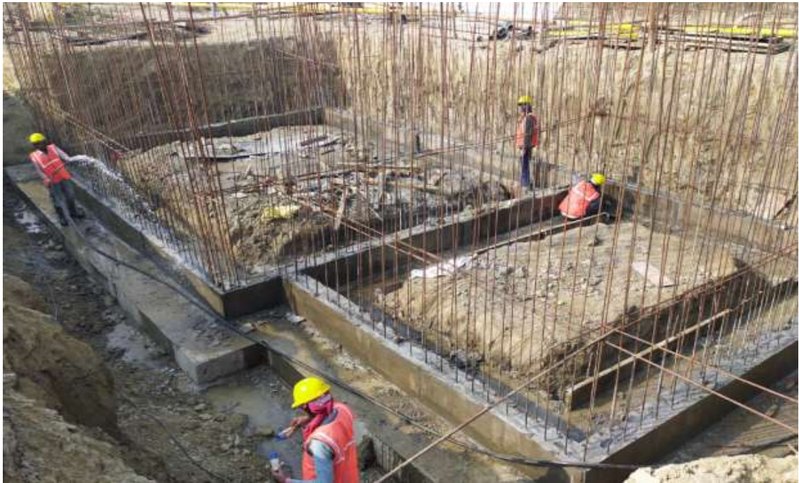
Curing at Centrifuge Building
