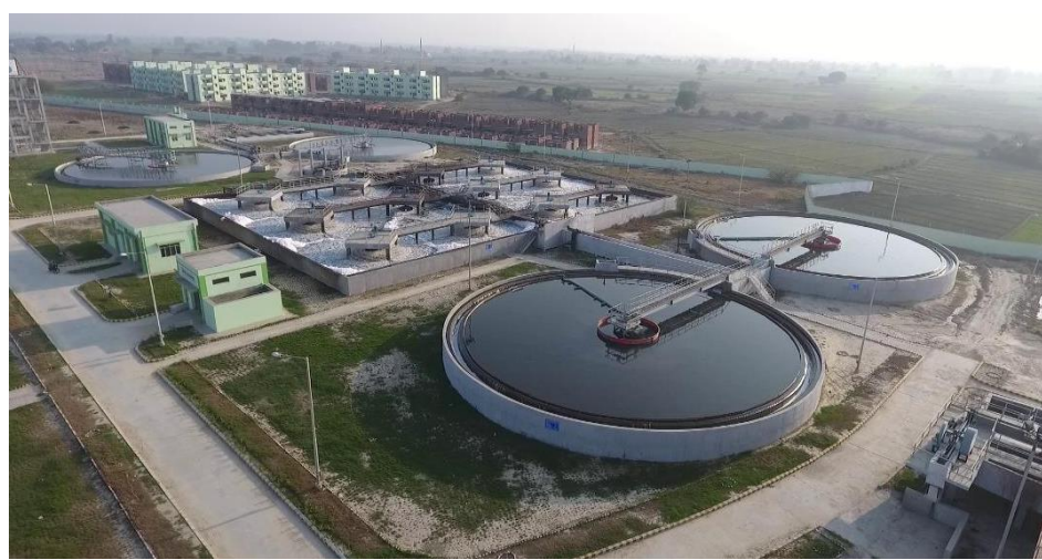
Sajari 42 MLD STP (ASP)
