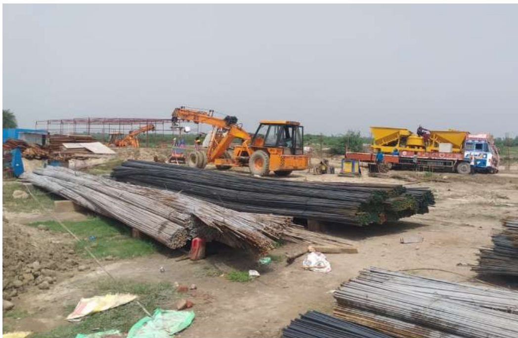
Steel / RMC plant unloading
