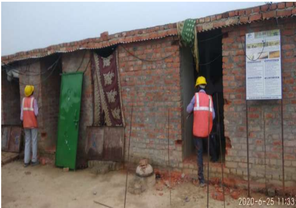
Ongoing work of Labour Kitchen
