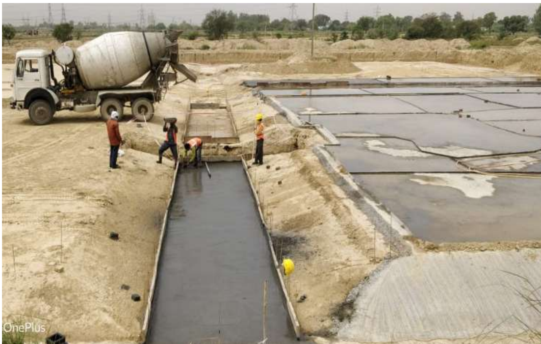
PCC work of SBR
