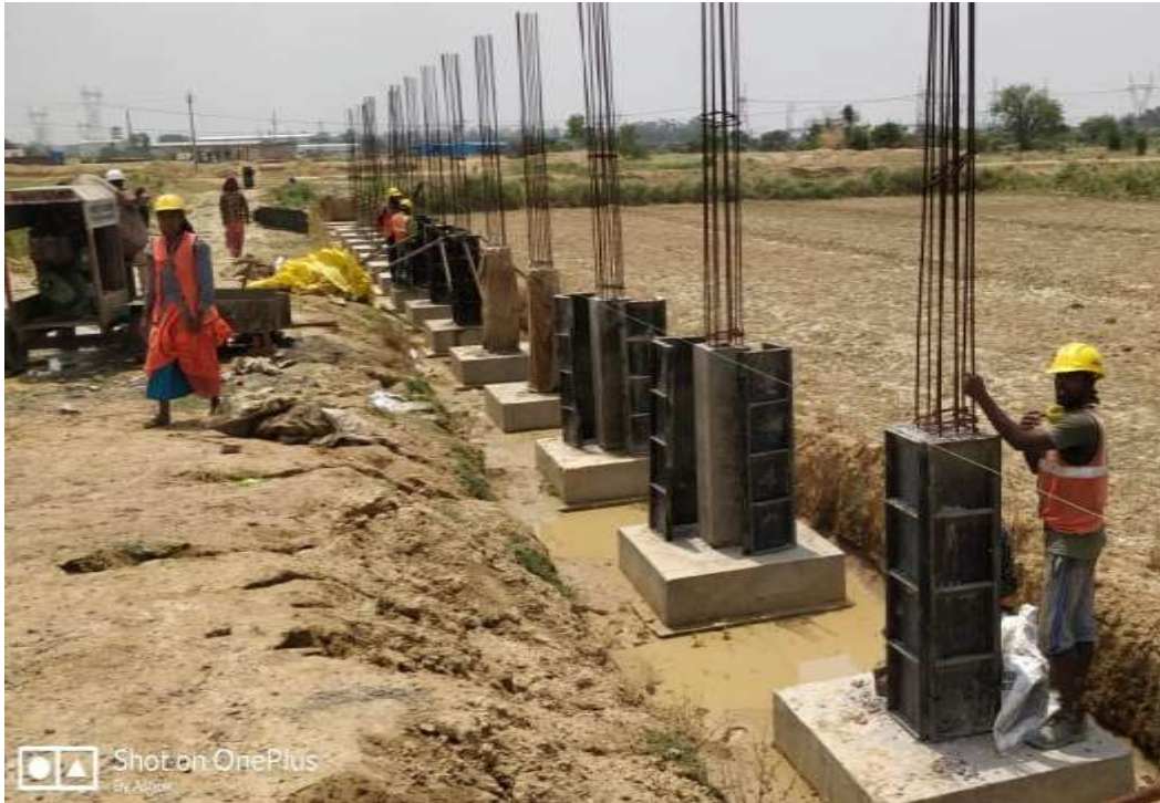
Boundary Wall work
