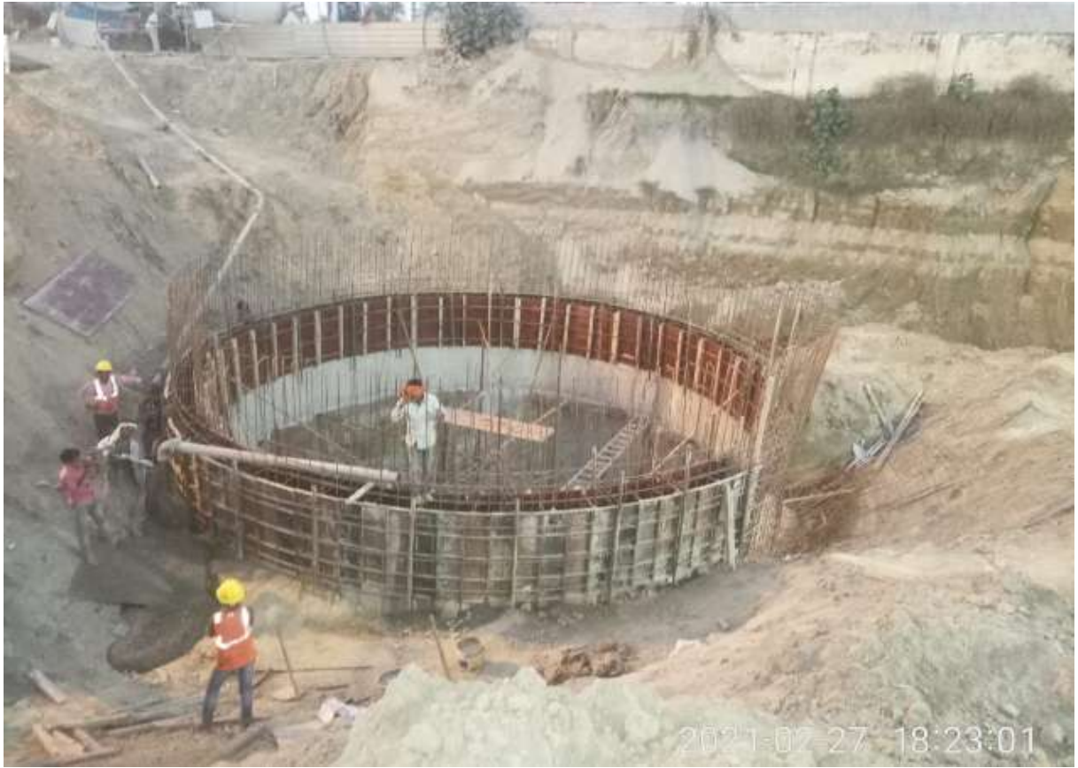
Sundar Nagar IPS Wall casting
