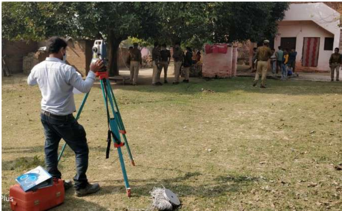
Geo Tech Survey work
