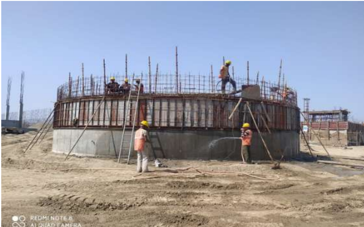
Sludge Thickener
