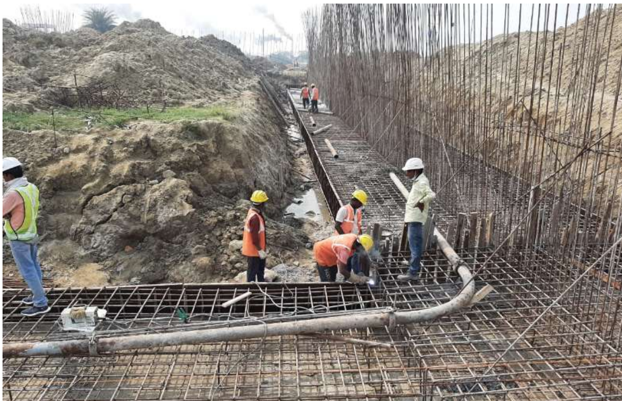
SBR Concrete work
