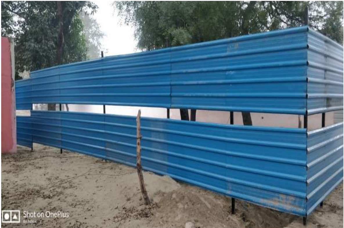
Fencing of the STP site
