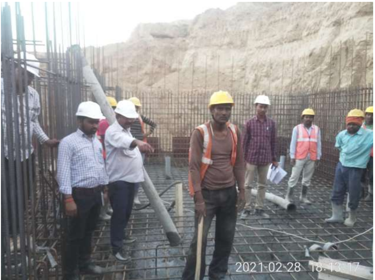
MPS receiving chamber raft casting
