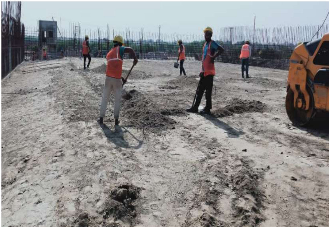
SBR filling, levelling & compacting
