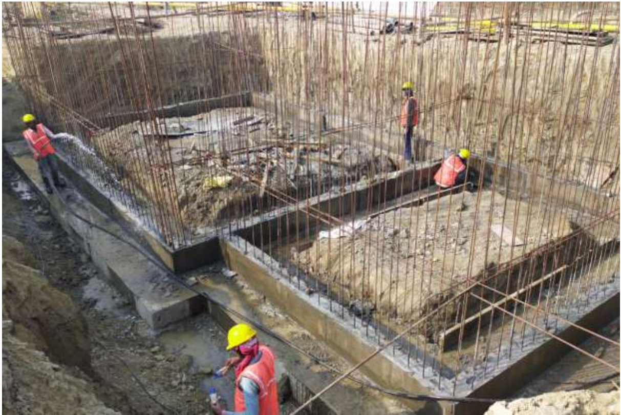
Centrifuge Building Curing
