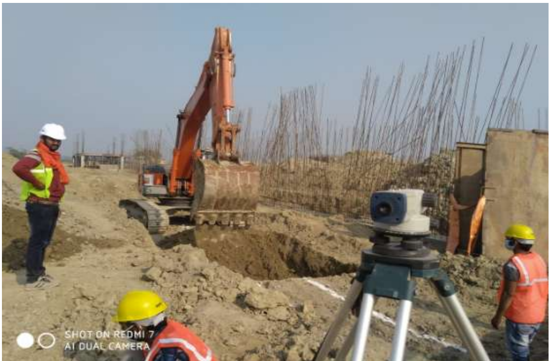
Excavation for 1200mm sewer laying work
