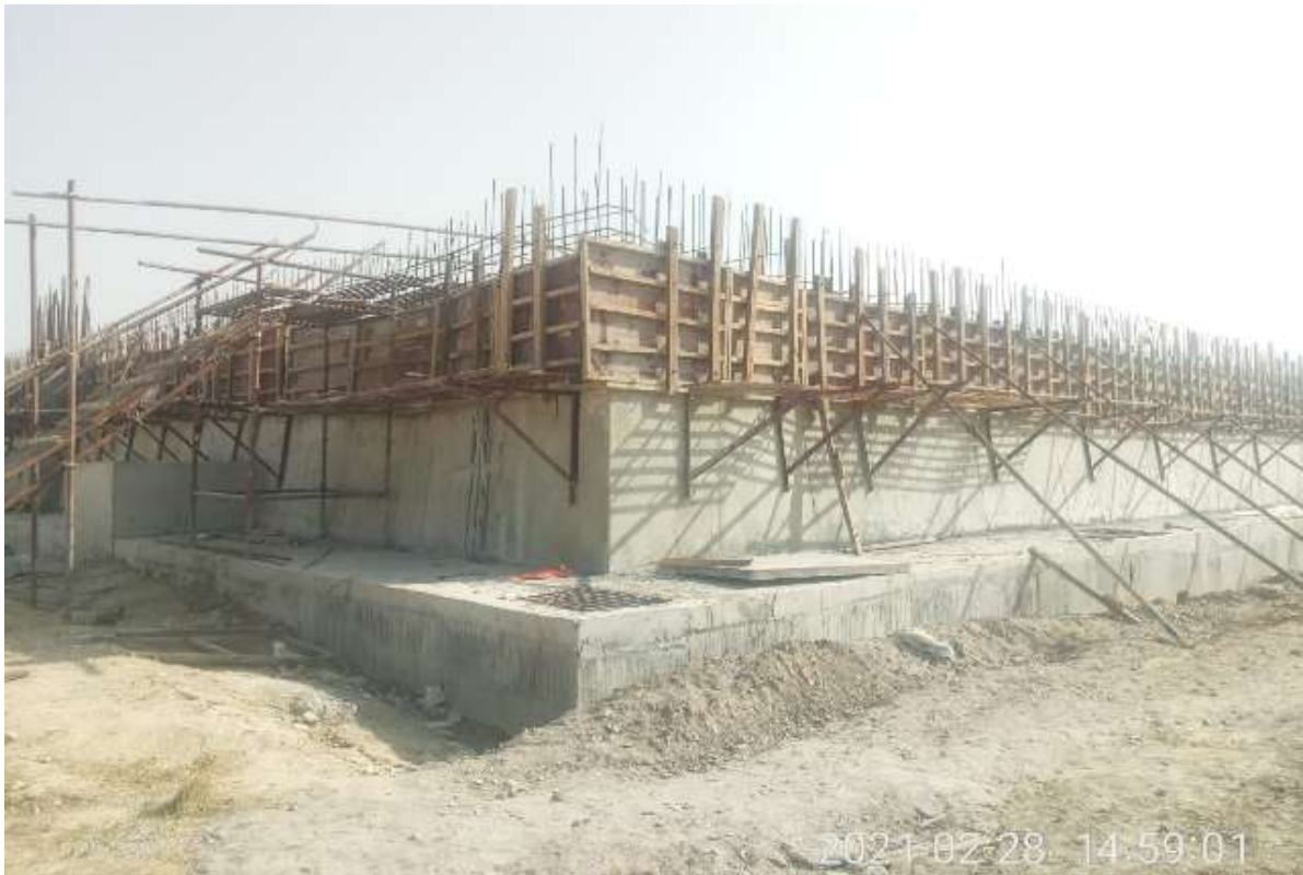
SBR Wall Shuttering
