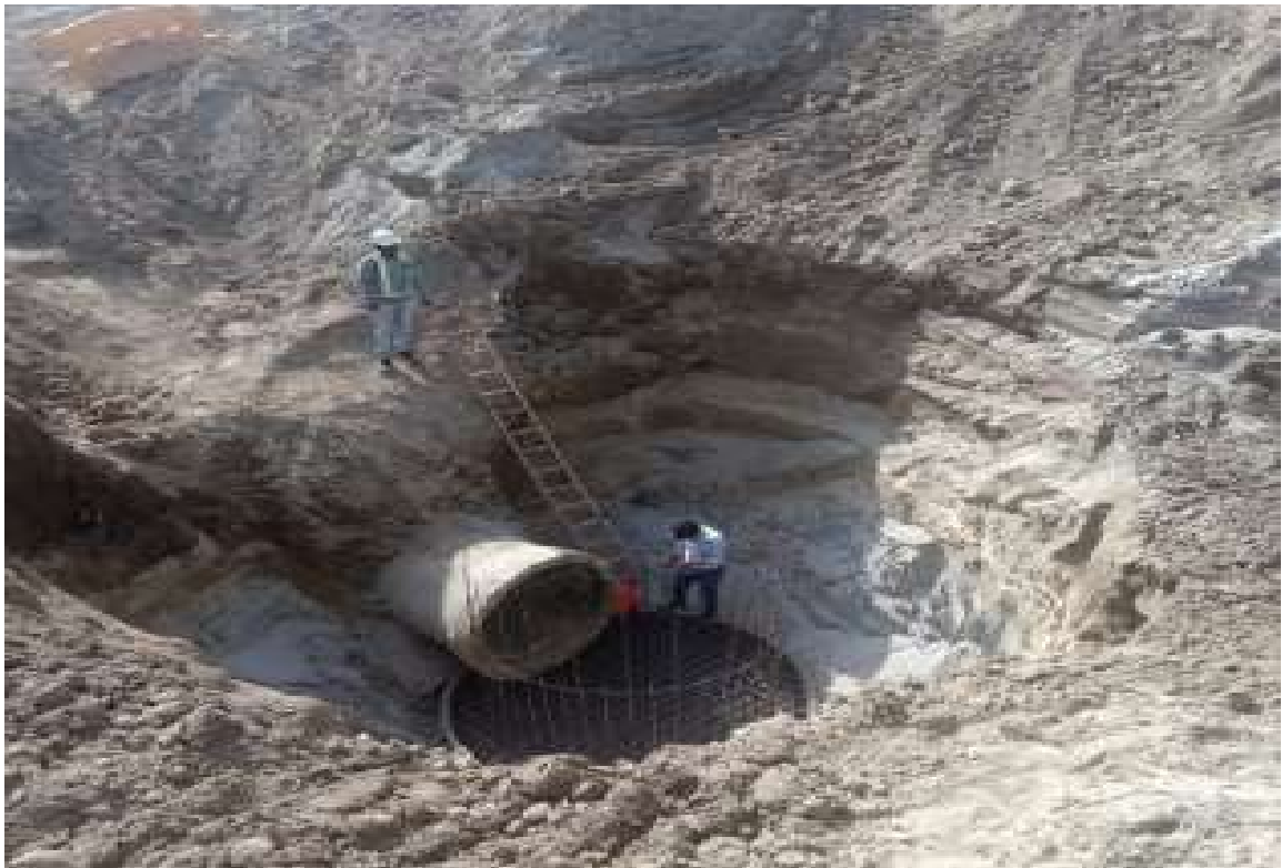
1200mm sewer laying work
