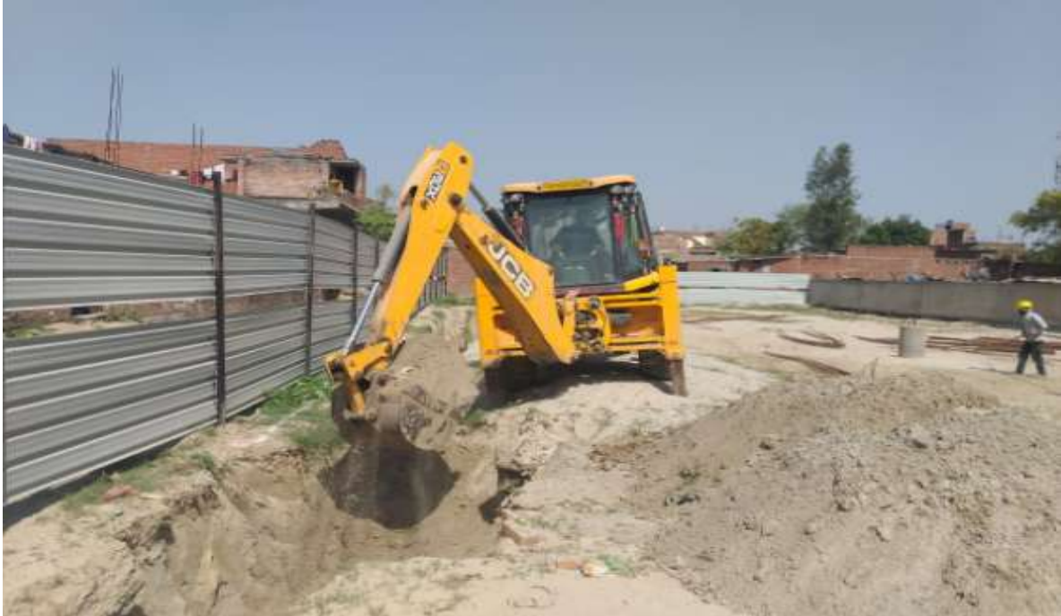
Boundary Wall excavation work
