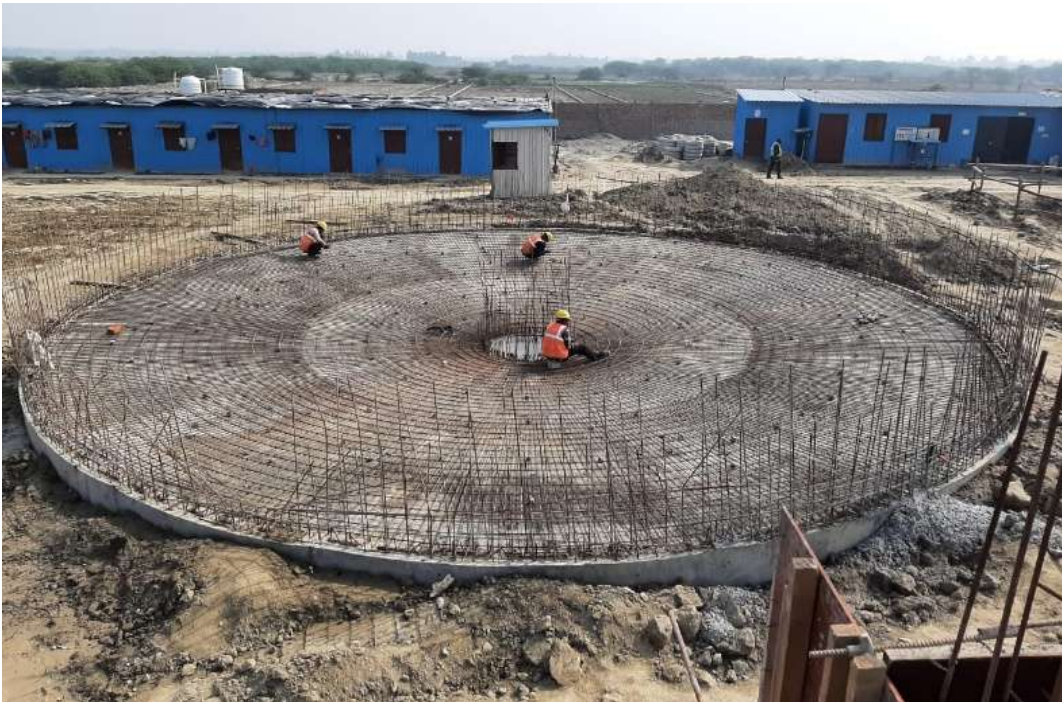
Supernatant Sump work
