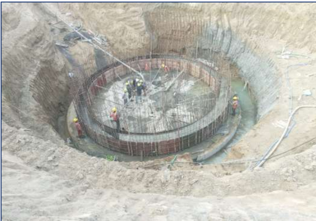
Sundar Nagar IPS Wall casting
