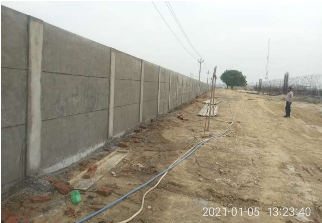
Boundary Wall work
