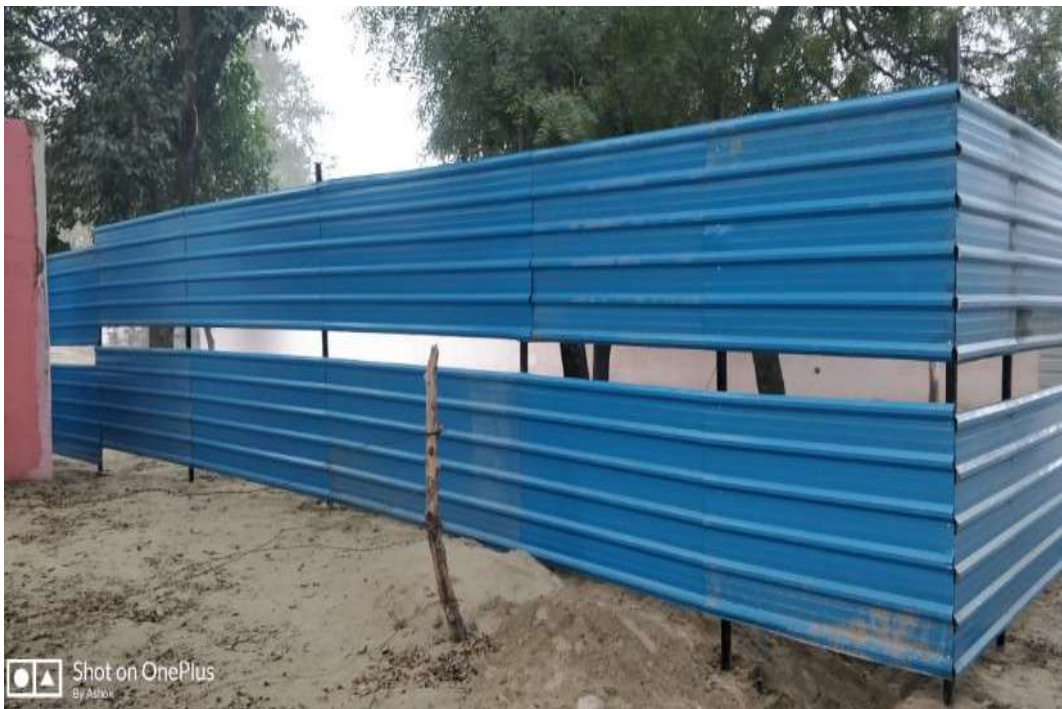
Fencing of the STP site
