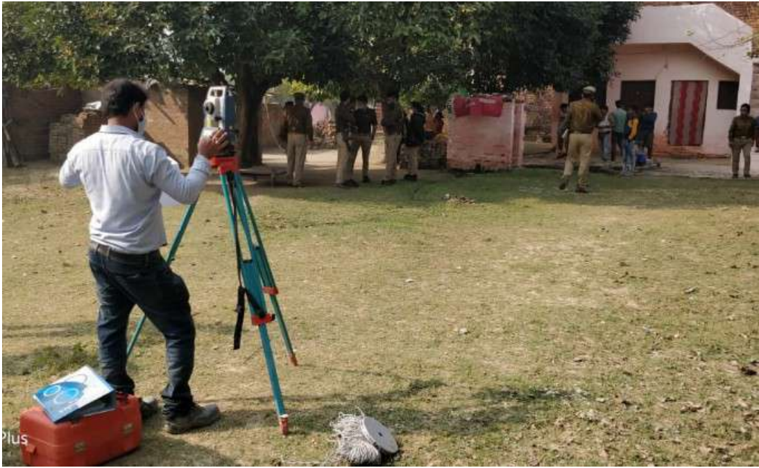
Geo Tech Survey work
