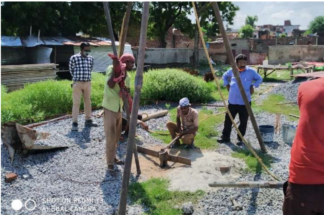
Geo Tech Survey work
