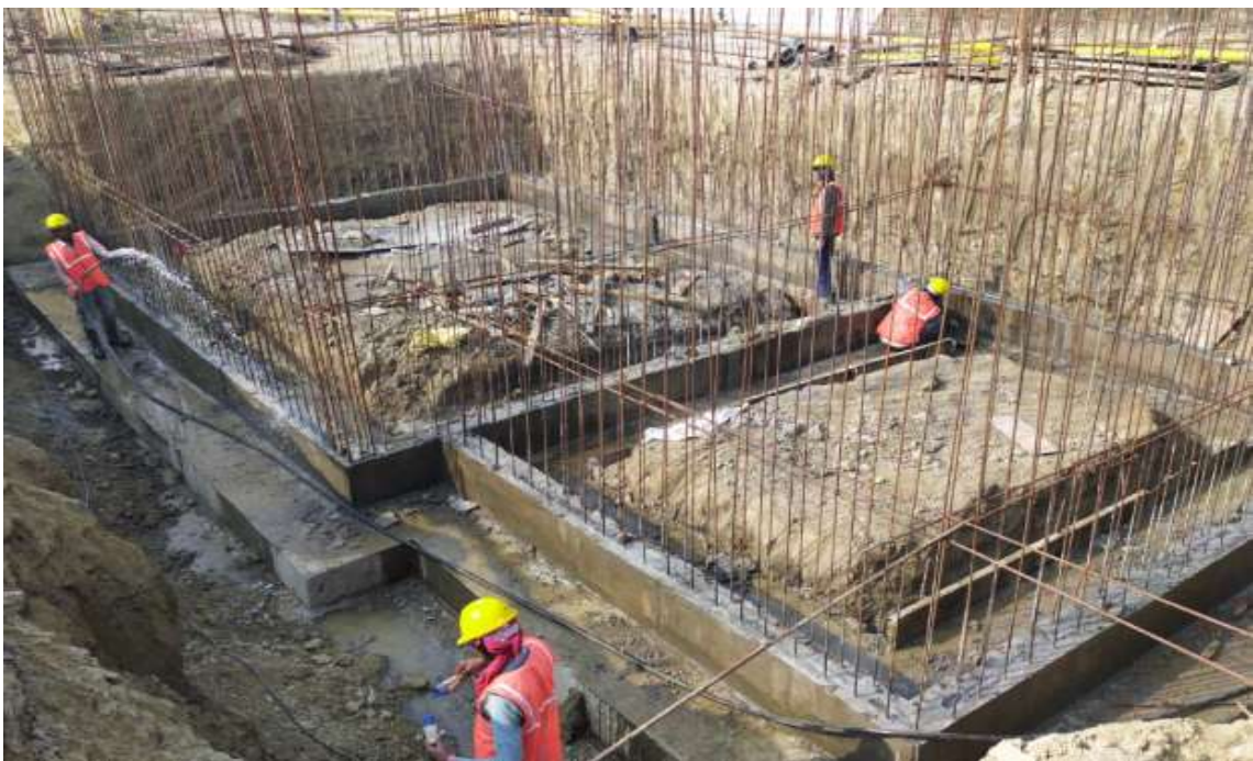
Curing at Centrifuge Building
