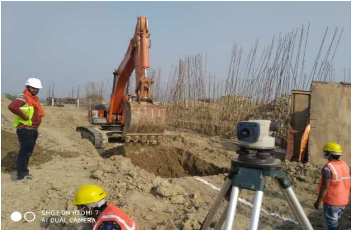
Excavation for 1200mm sewer laying work
