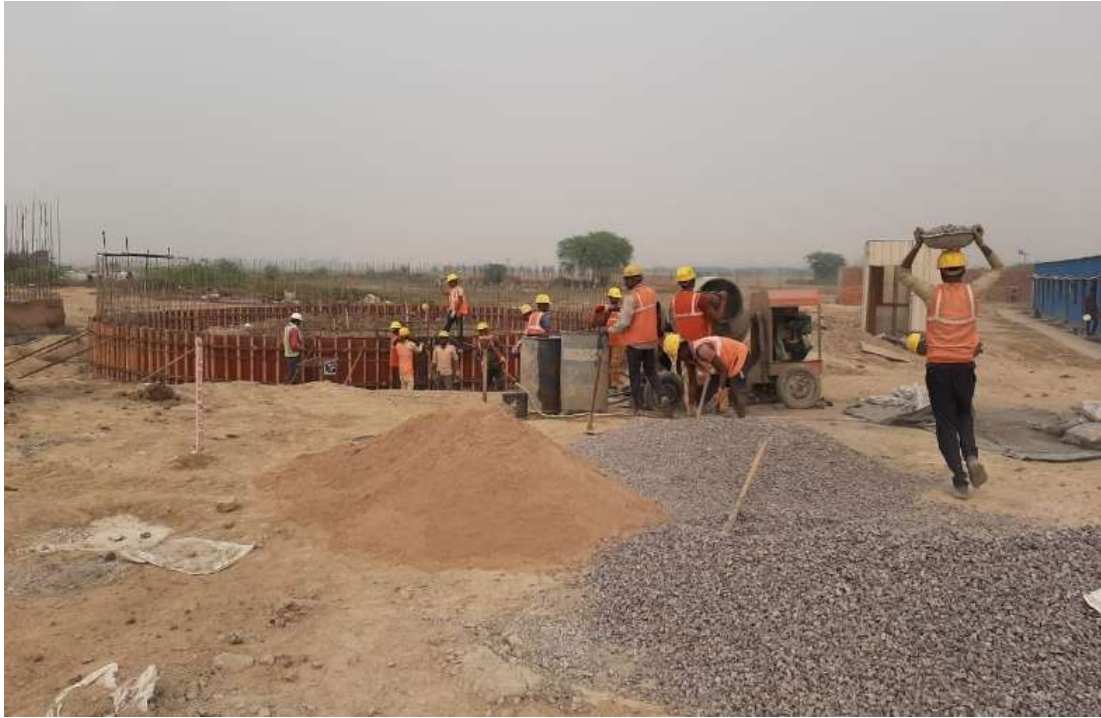
Ongoing work of Sludge Thickener
