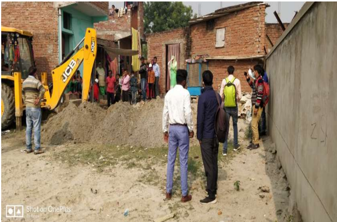
Geo Tech Survey work
