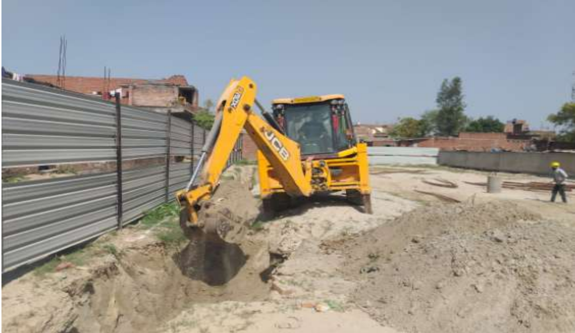
Boundary Wall excavation work
