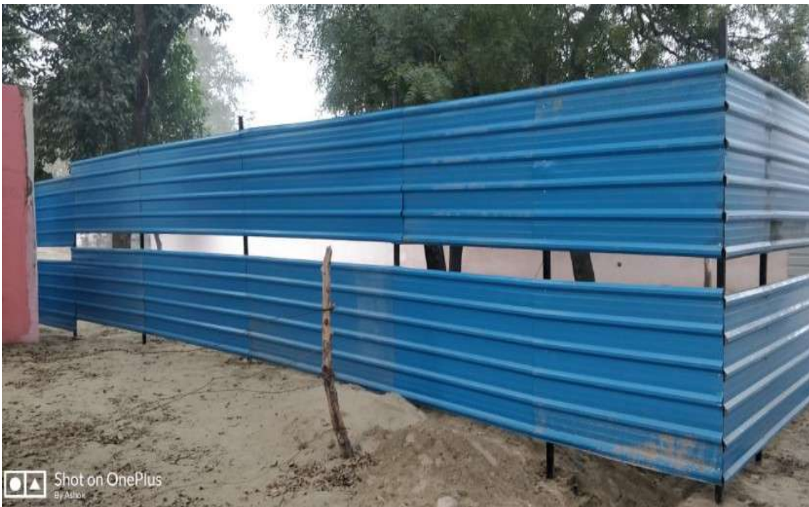
Fencing of the STP site
