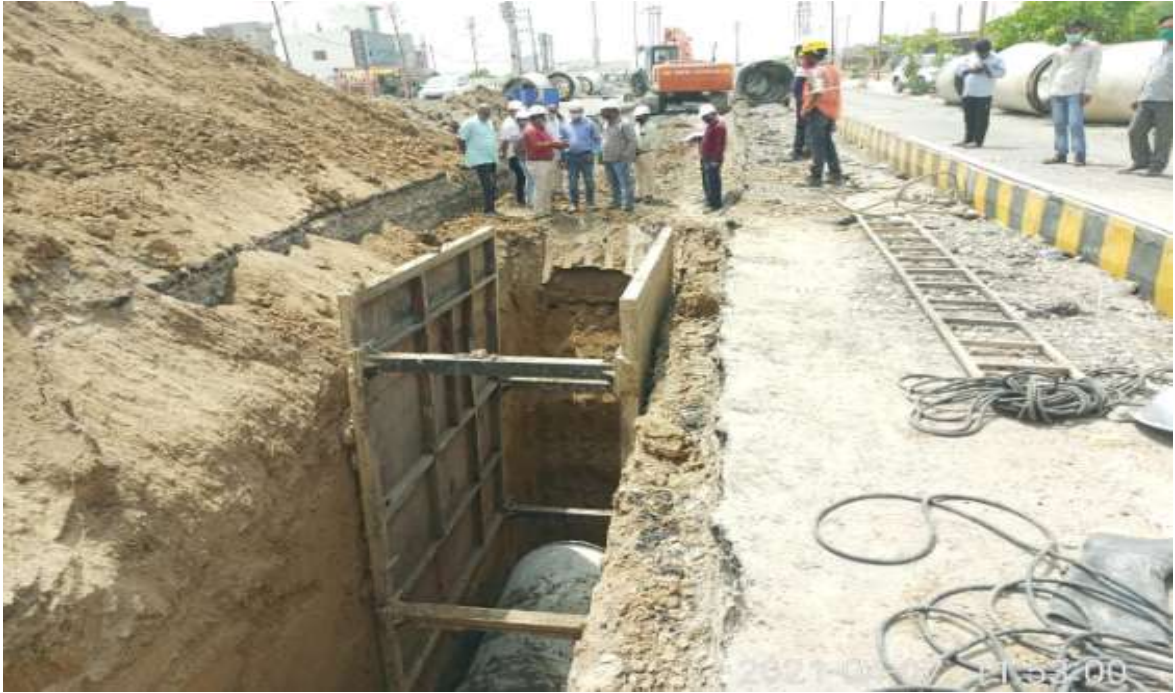
1200 dia pipe laying during GM visit
