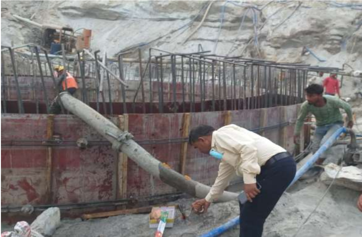
MPS wall 3rd lift RCC
