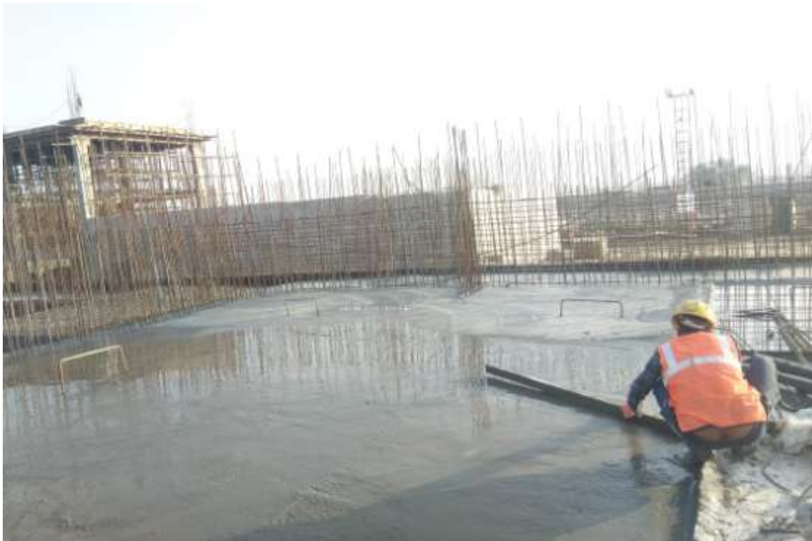
SBR Raft casting work
