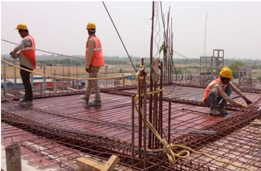
CCT Building Roof Slab
