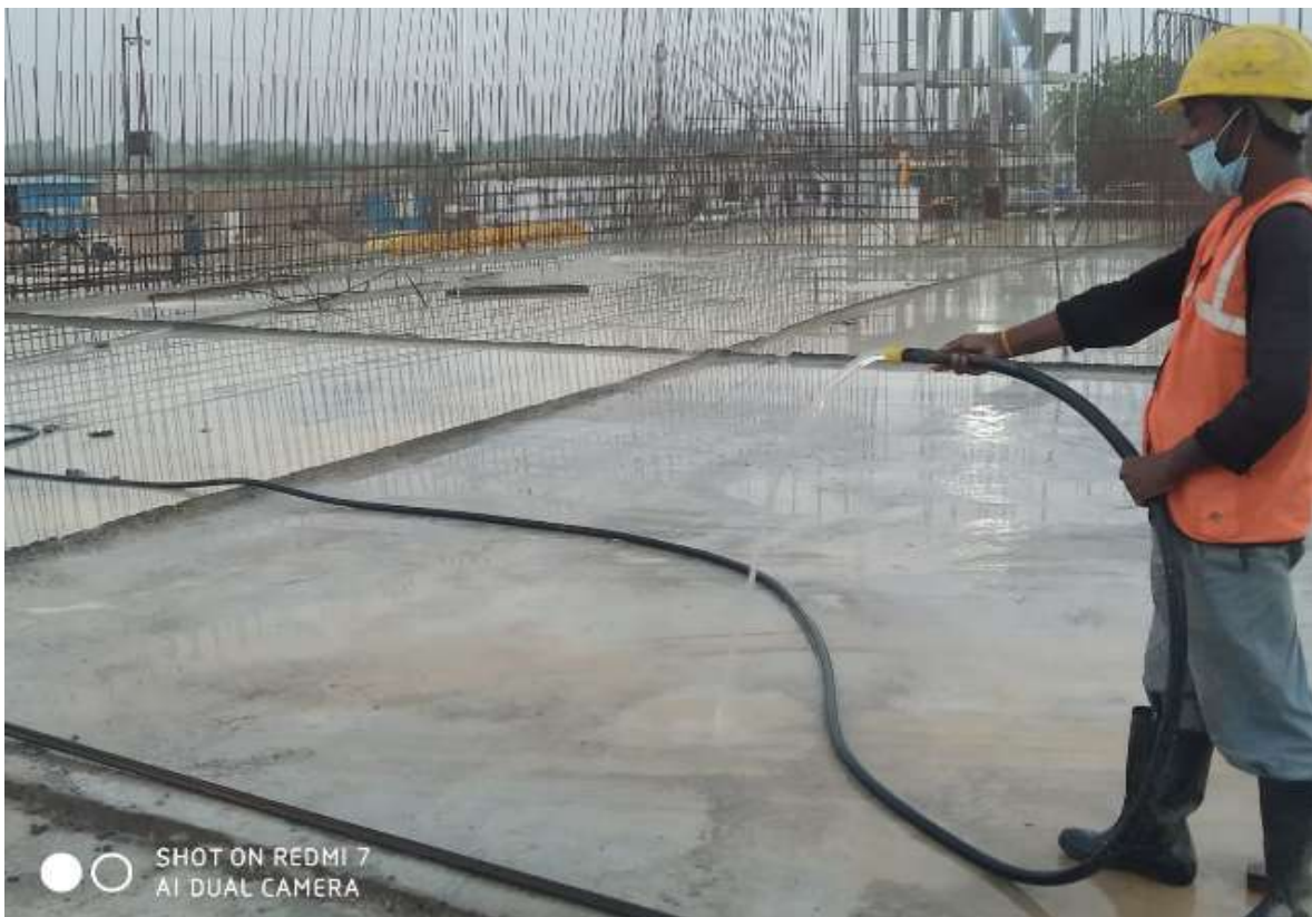
SBR floor curing
