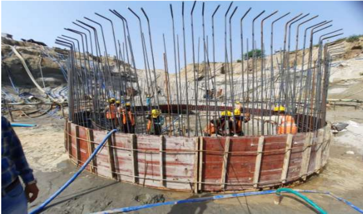
MPS steel binding work
