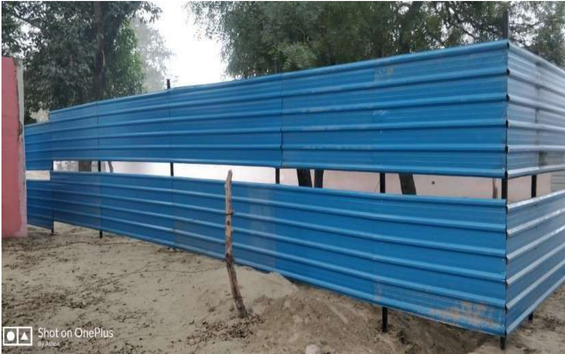
Fencing of the STP site
