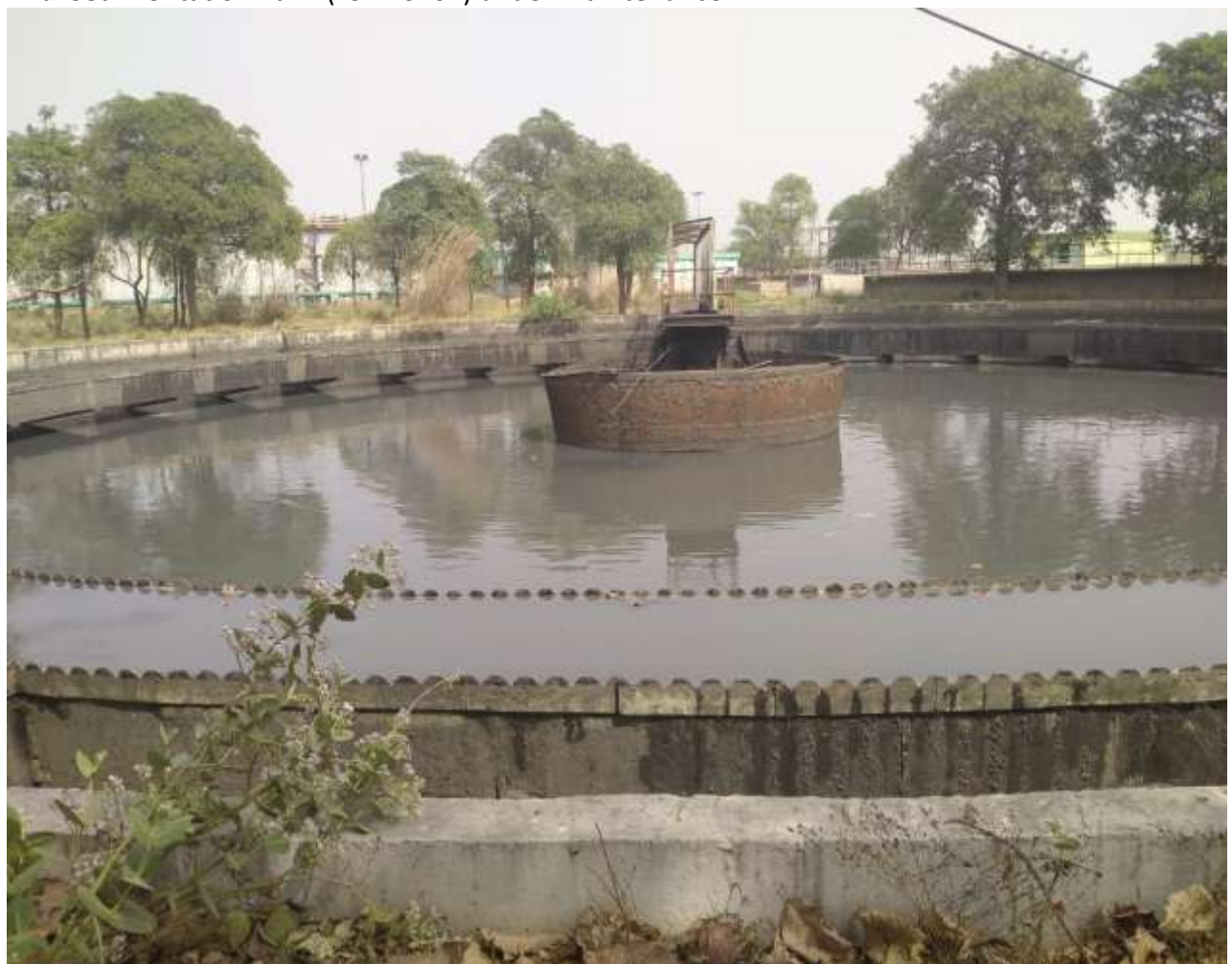
Final Sedimentation Tank (FST no. 01) under maintenance
