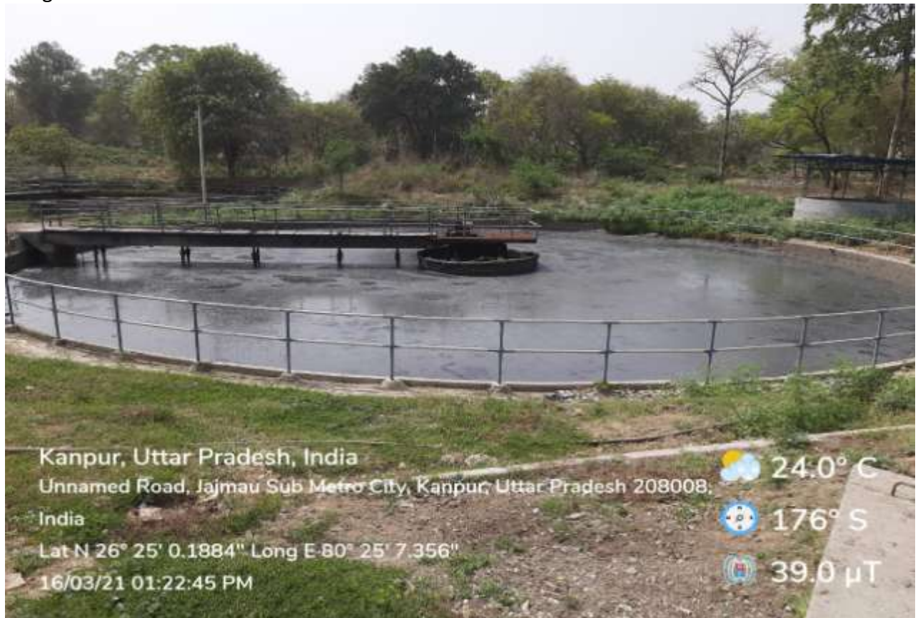
Sludge Thickener
