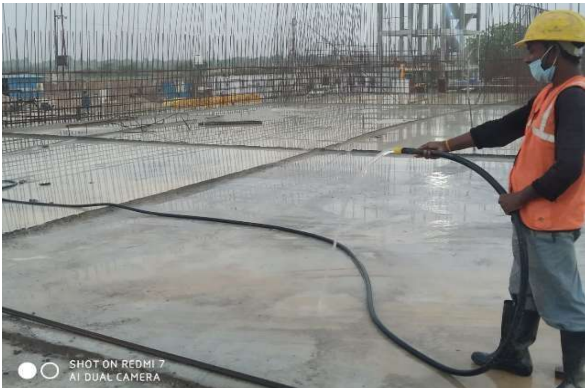
SBR floor curing
