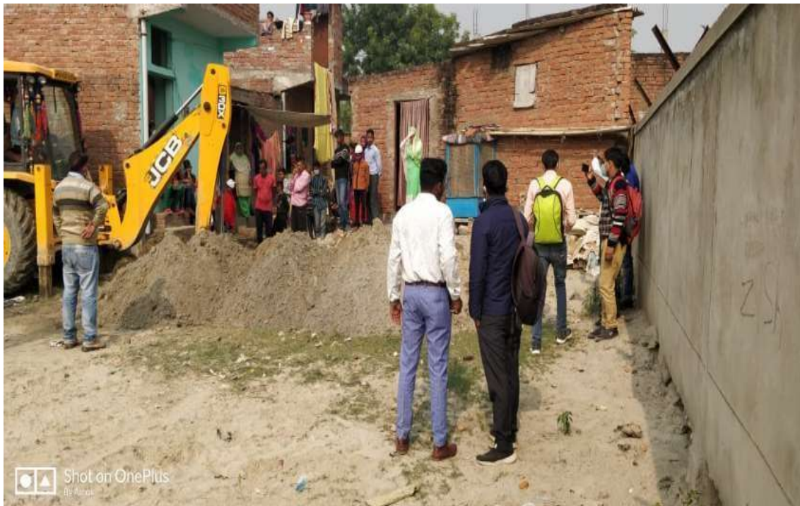
Boundary Wall excavation work
