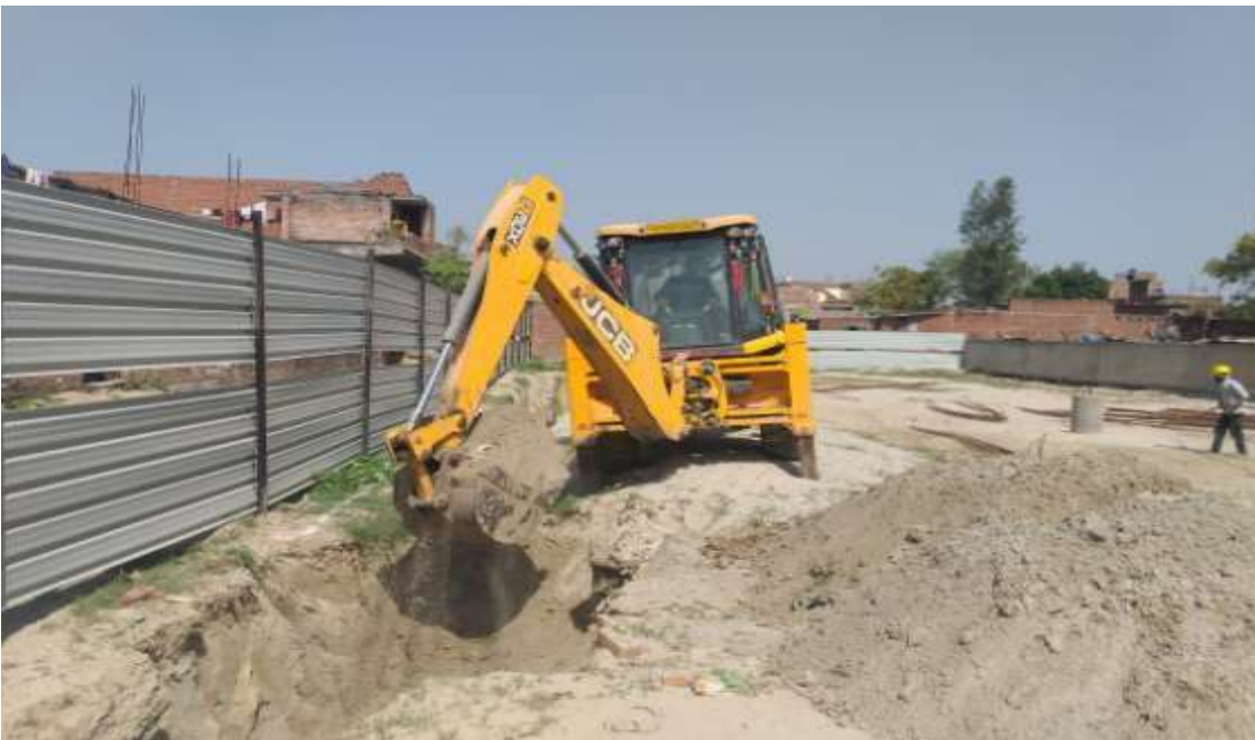
Boundary Wall excavation work
