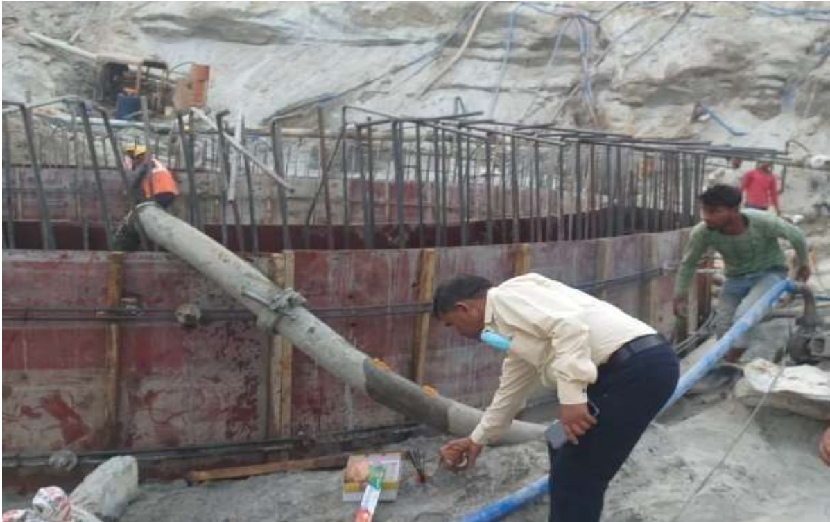
MPS wall 3rd lift RCC
