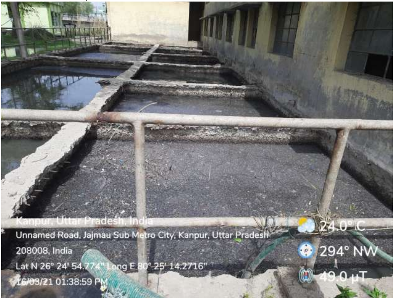
Treated Effluent Sump
