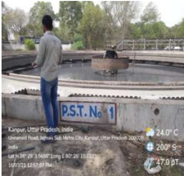
PST no. 01 under maintenance.
