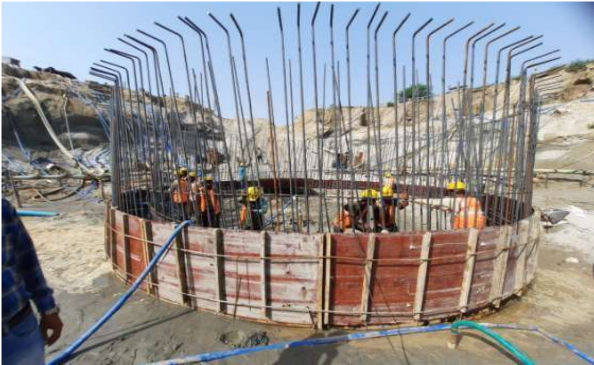
MPS steel binding work
