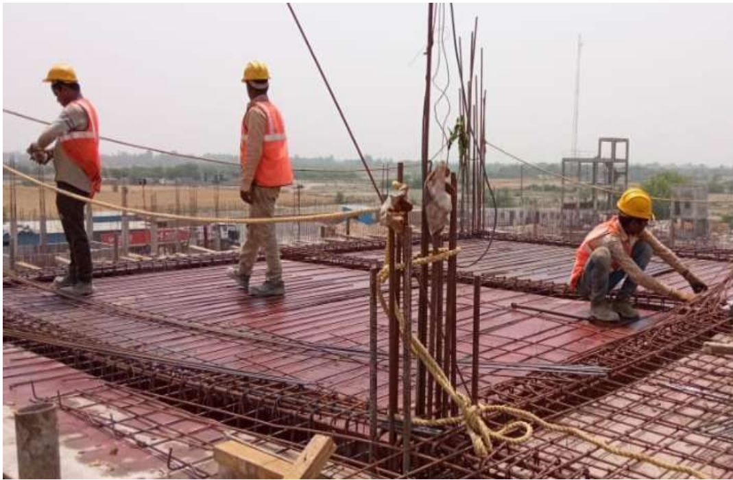
CCT Building Roof Slab
