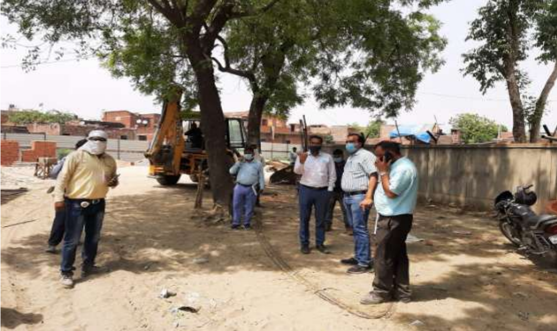
CE UPJN, Lucknow visit dated 09.04.2021
