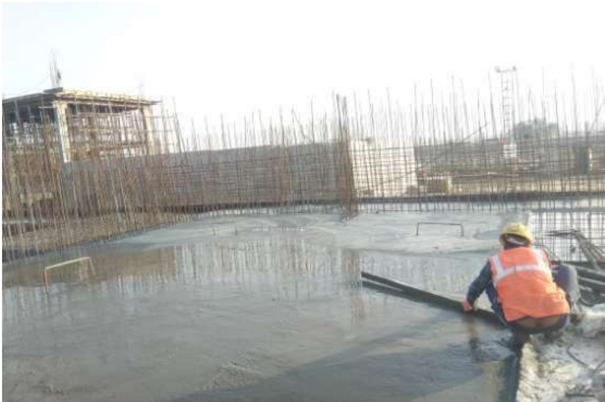
SBR Raft casting work
