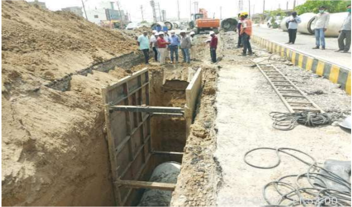
1200 dia pipe laying during GM visit
