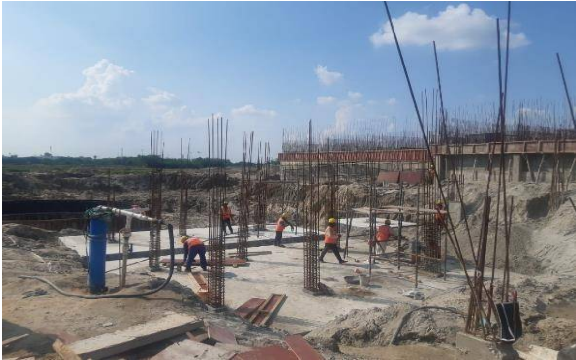
Admin Building works
