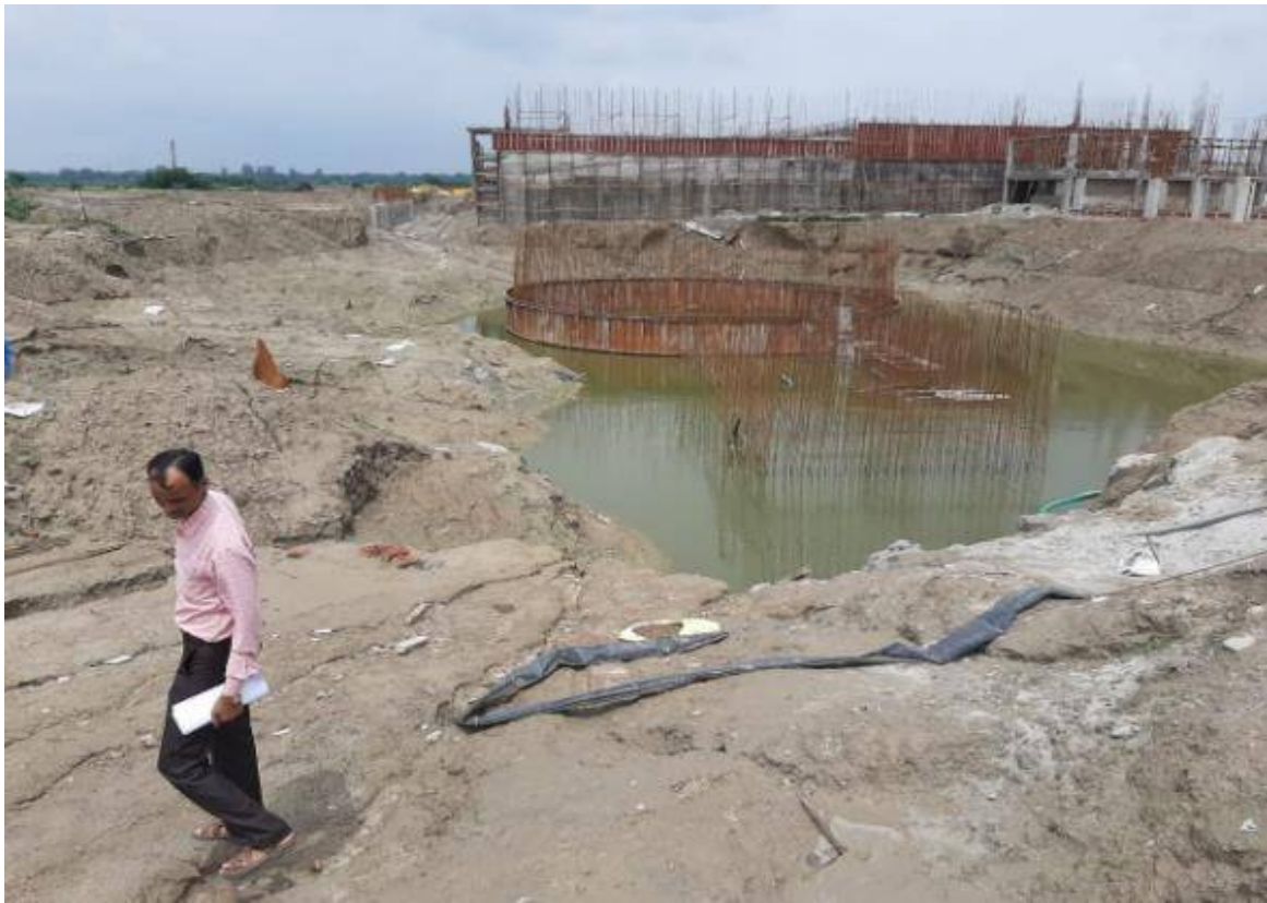
No work at MPS due to rain water logging
