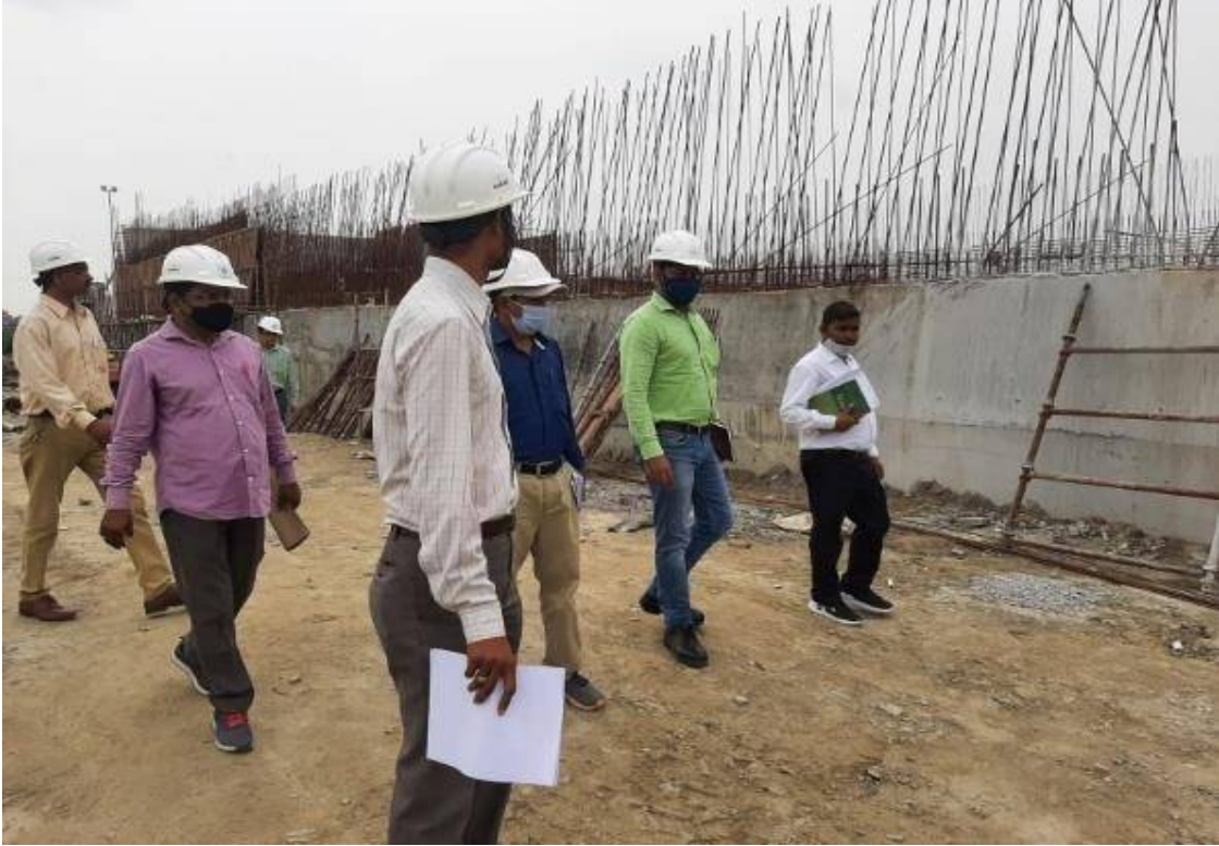
SBR wall steel binding
