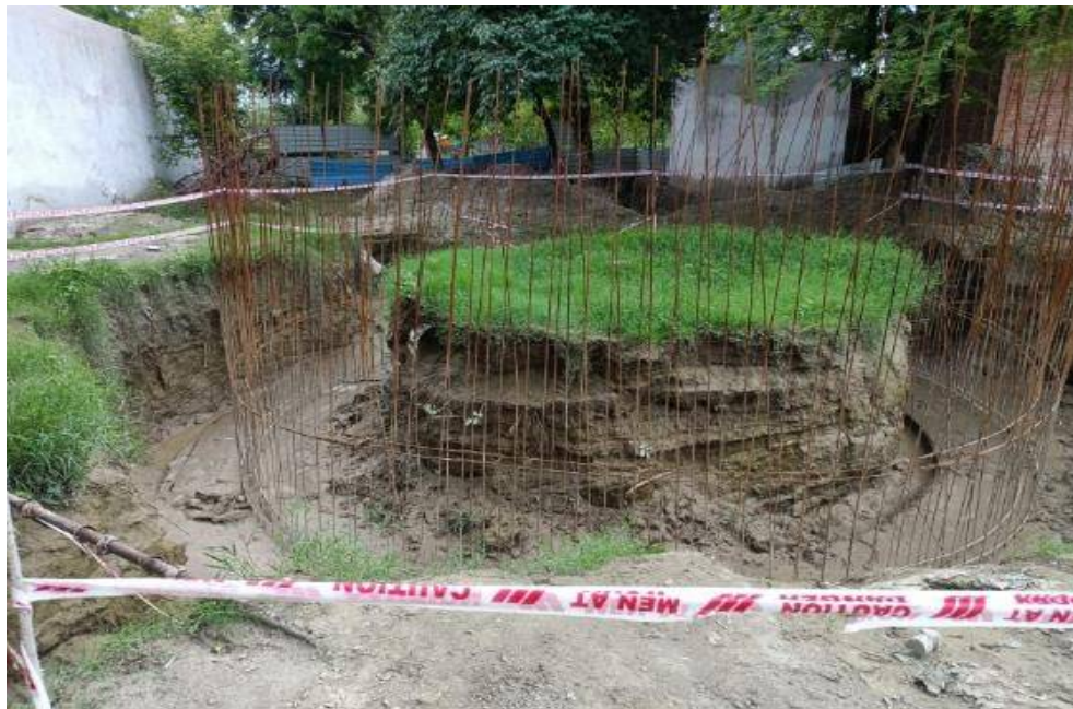
Sludge Thickener PCC
