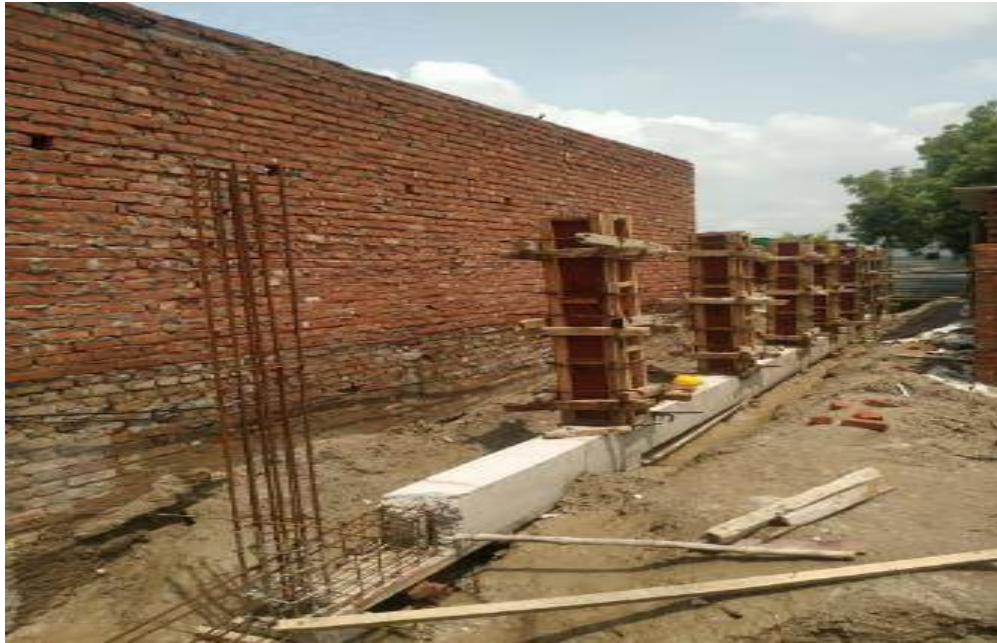
Boundary Wall work
