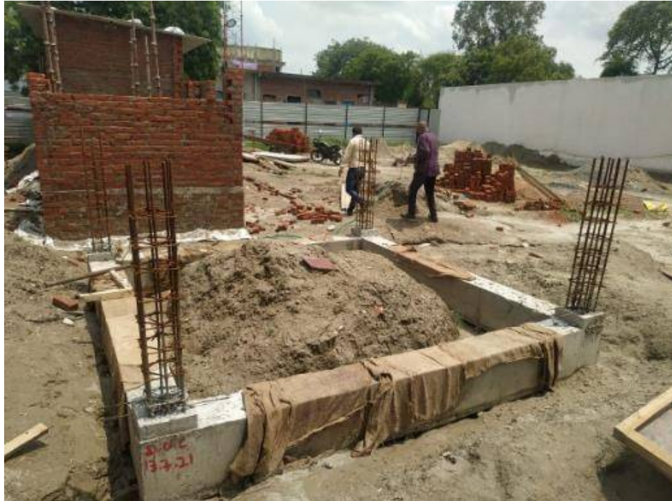
Guard Room Works
