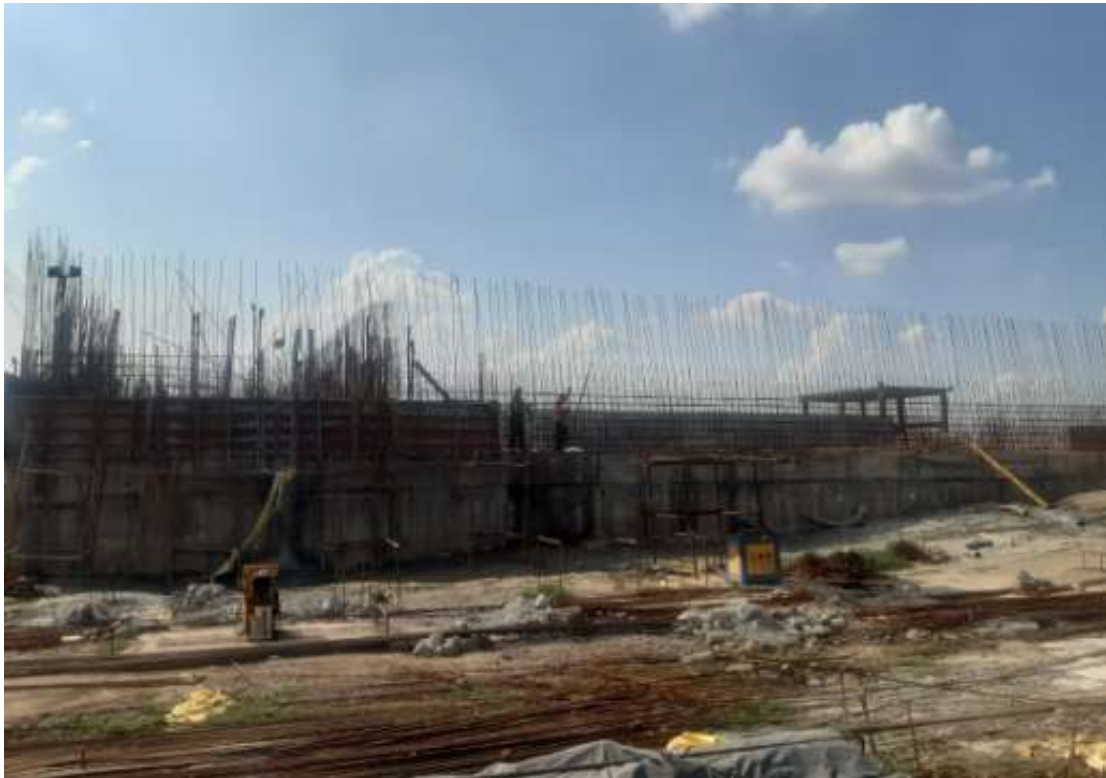
SBR wall lift work
