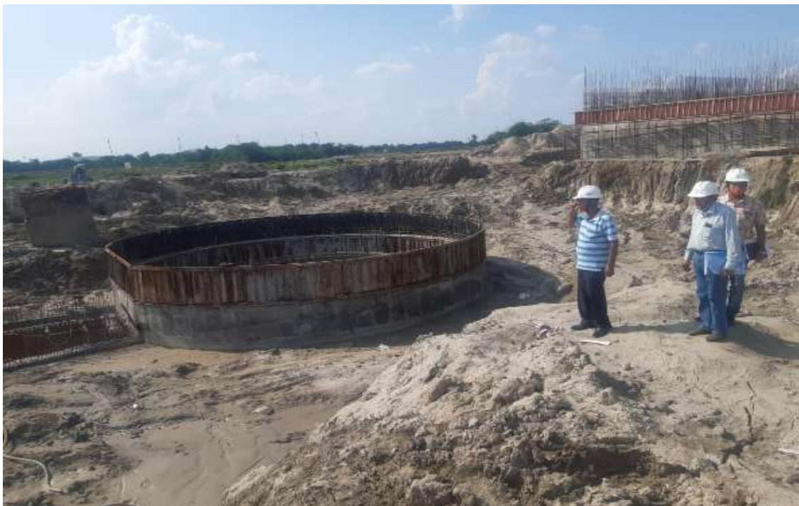
MPS works Inspection by PE dated 13.07.2021
