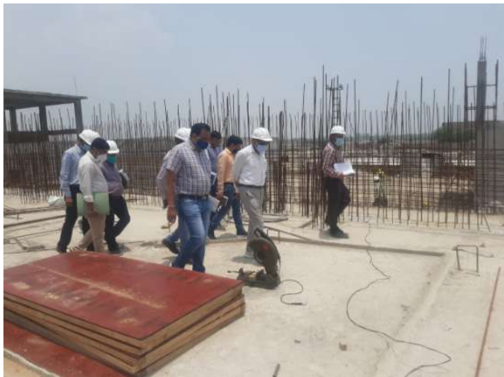
Unnao work inspection by CE, Lucknow dated 07.07.2021
