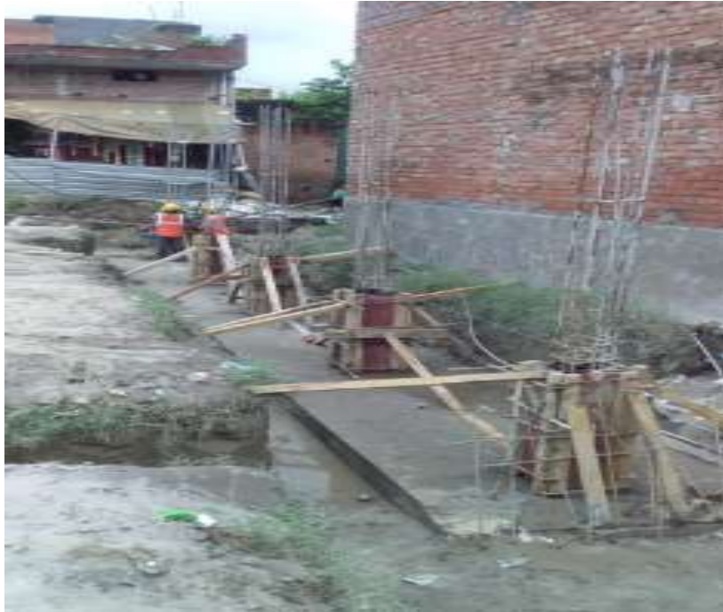
Boundary Wall work
