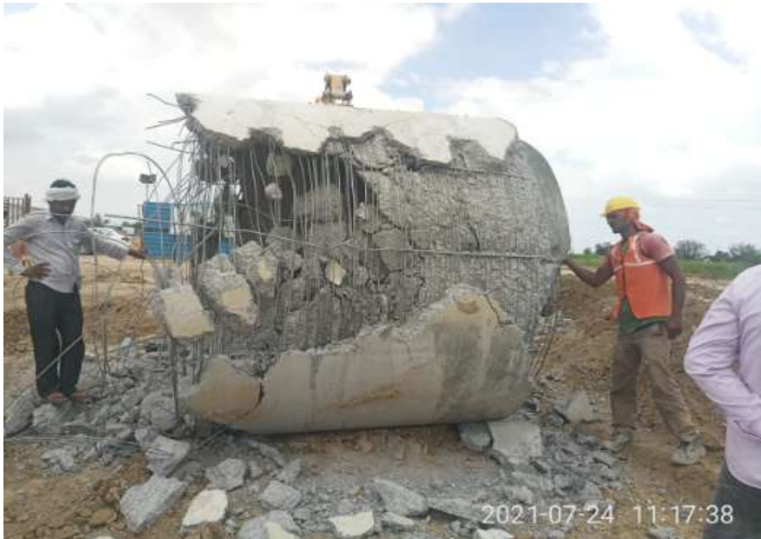
RCC pipe 1600 dia testing for reinforcements
