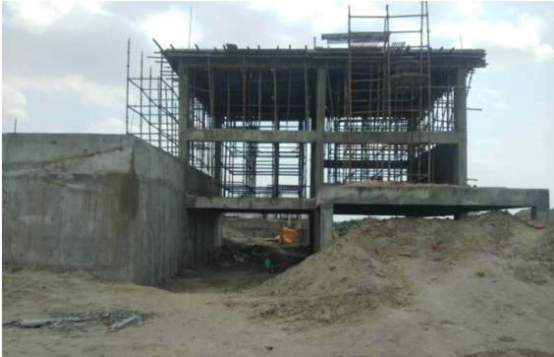
CCT Building work
