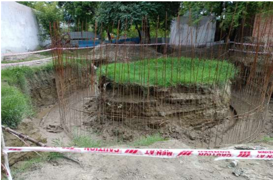
Sludge Thickener PCC
