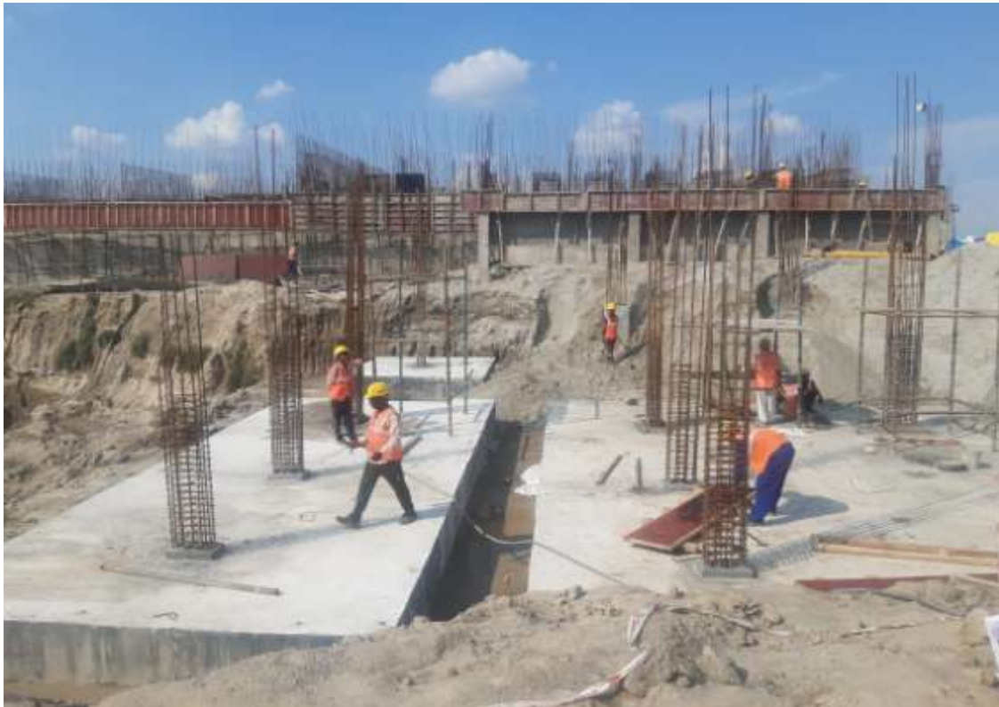
Admin building foundation
