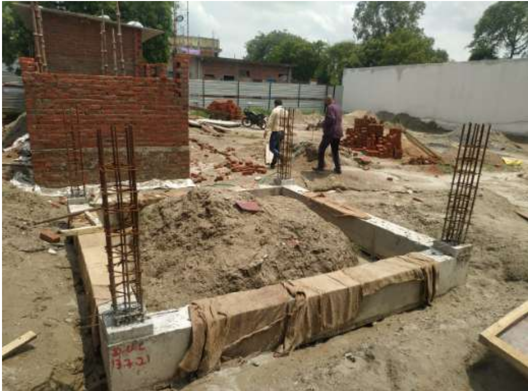
Guard Room Works
