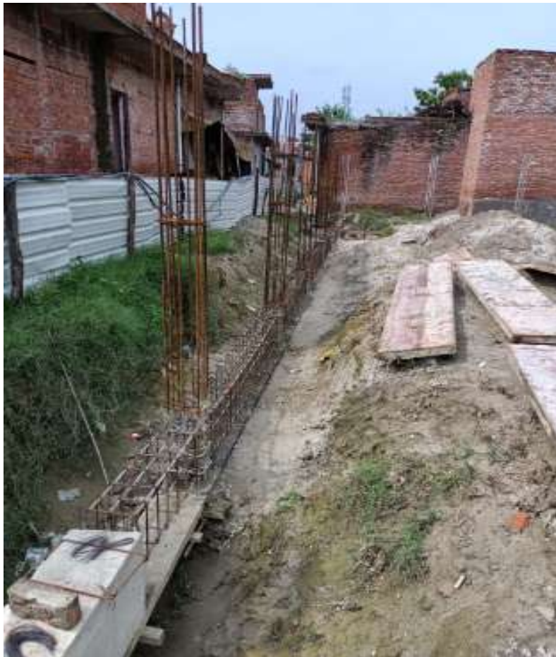
Boundary Wall work
