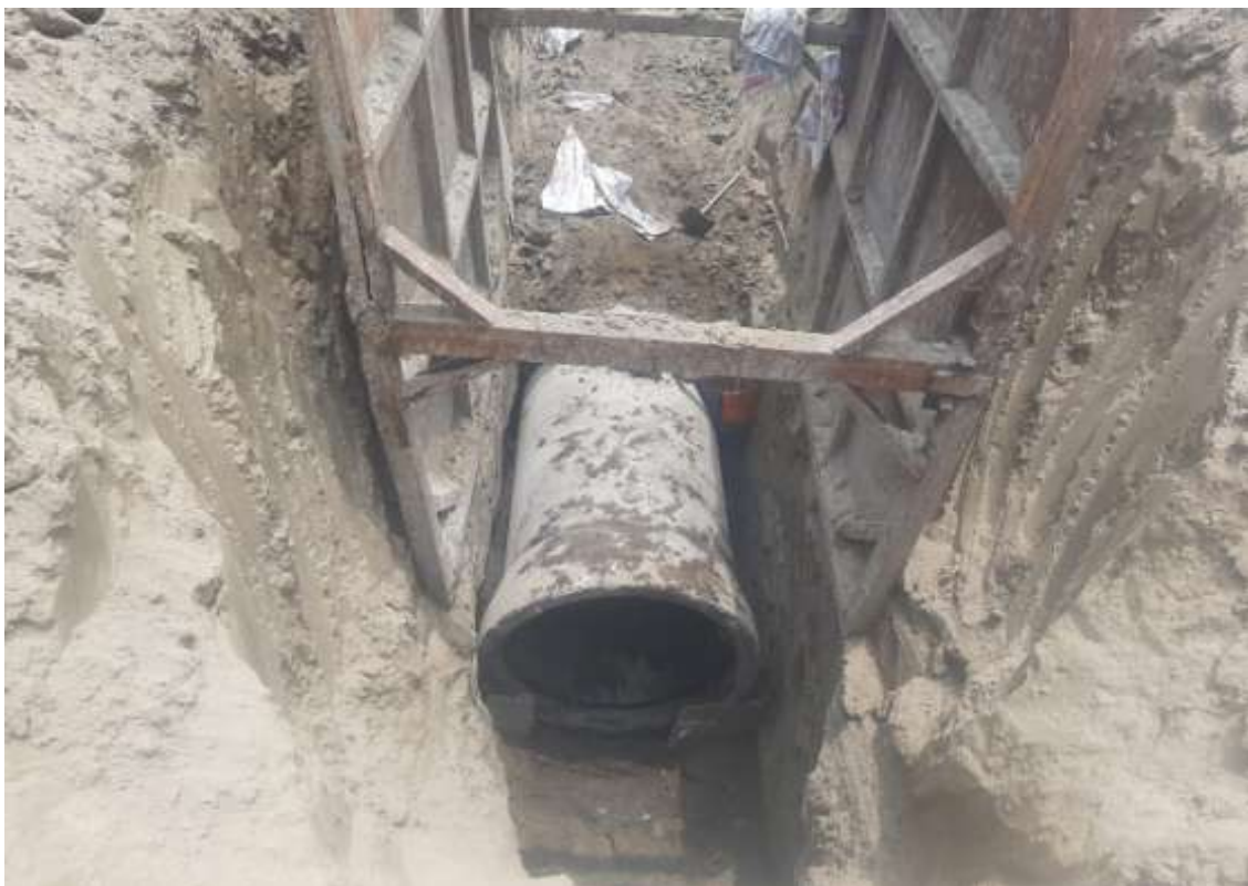
1200 mm Sewer Laying works
