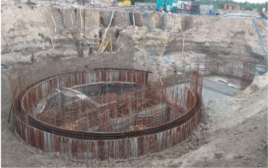
MPS steel binding work
