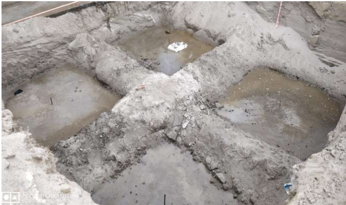
Guard Room PCC Works
