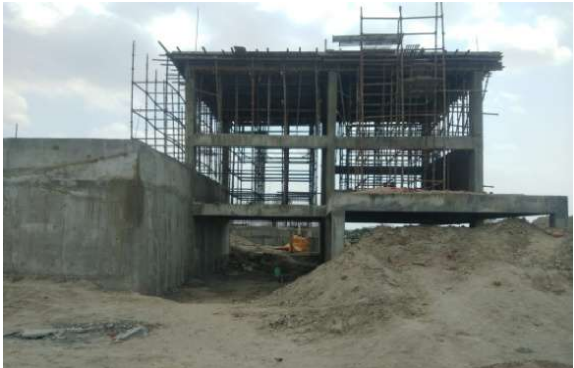
CCT Building work
