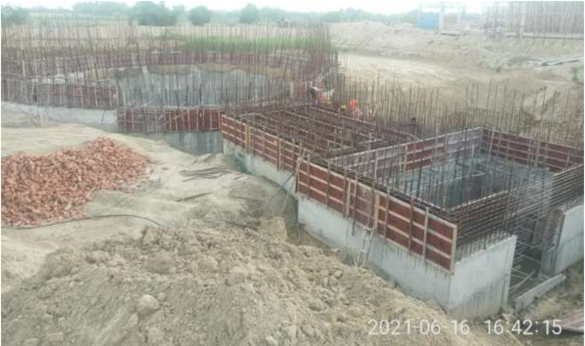
MPS and Receiving chamber
