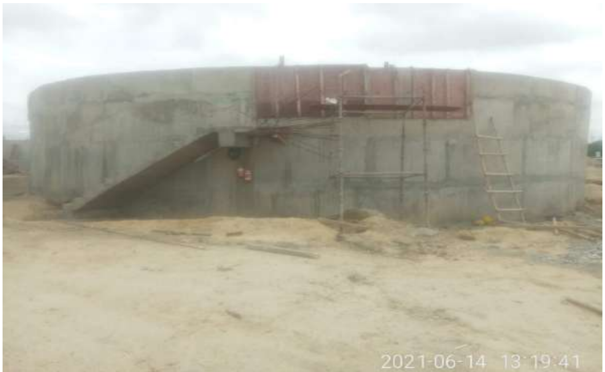
Sludge Thickener
