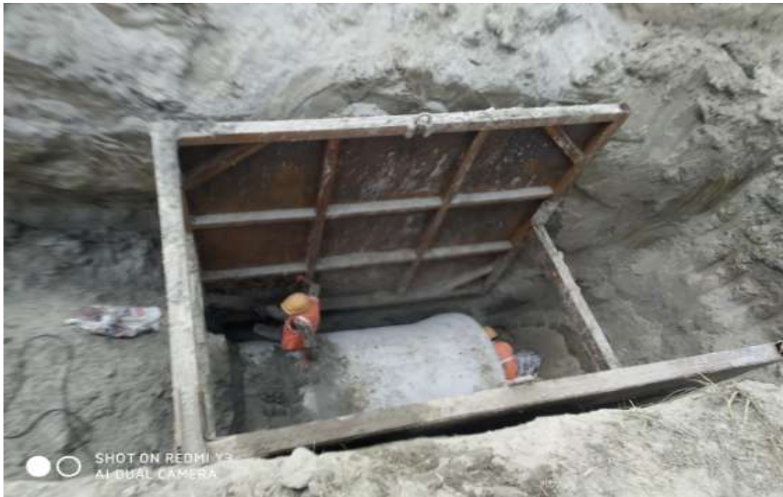
1200 mm Sewer Laying works
