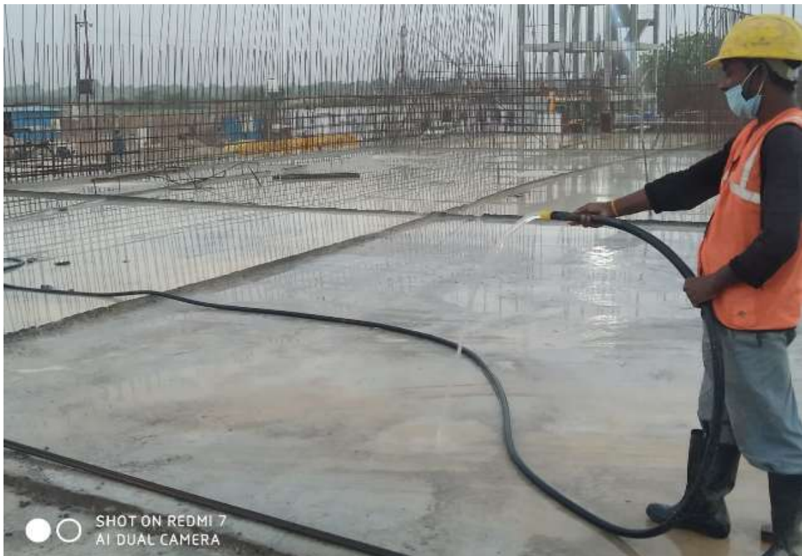
SBR floor curing
