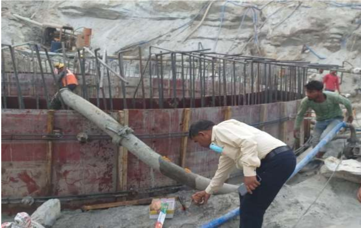
MPS wall 3rd lift RCC
