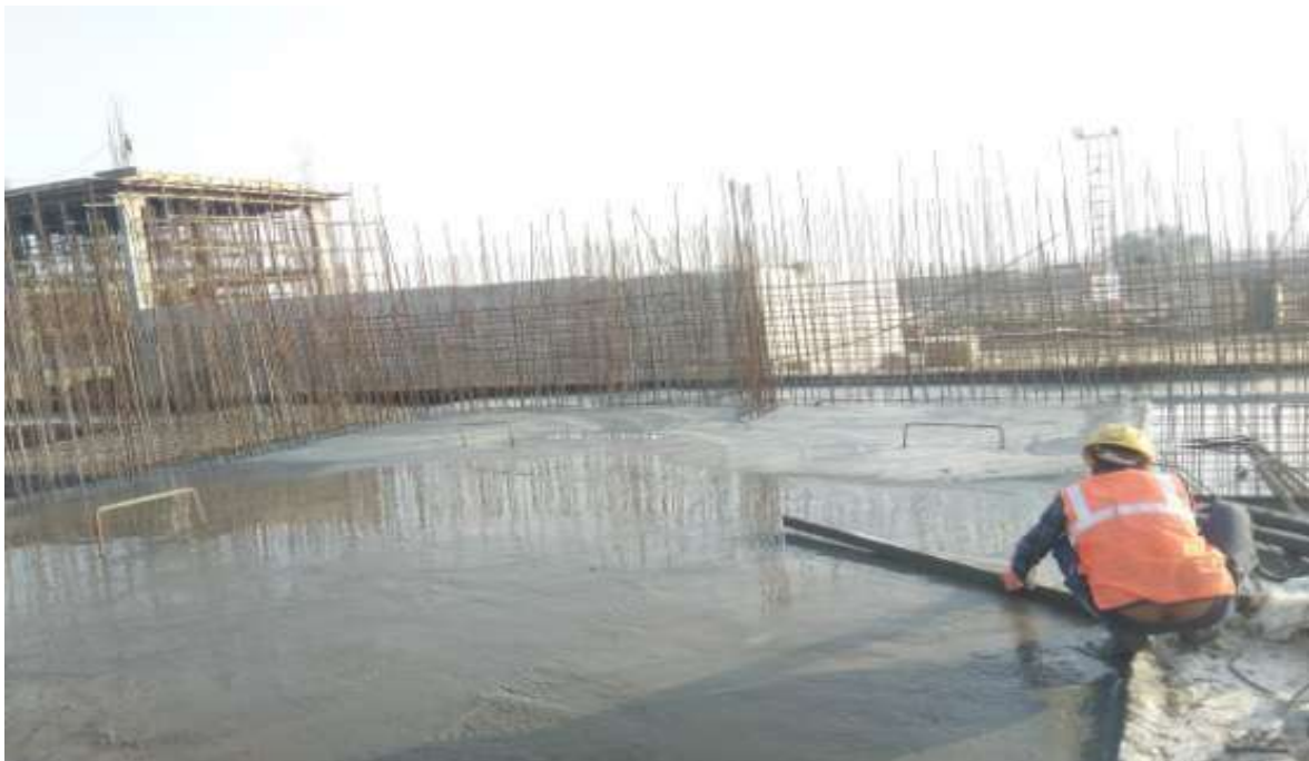
SBR Raft casting work
