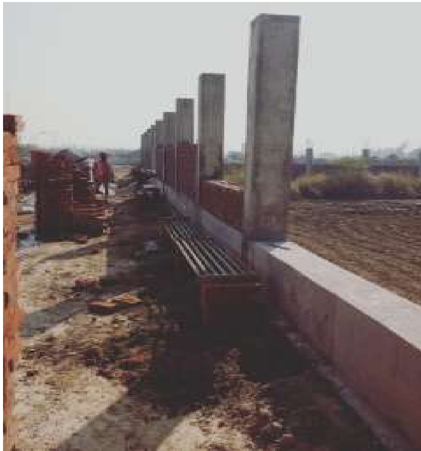
Boundary Wall work
