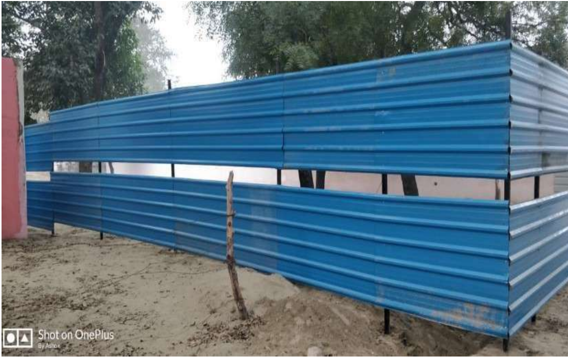
Fencing of the STP site
