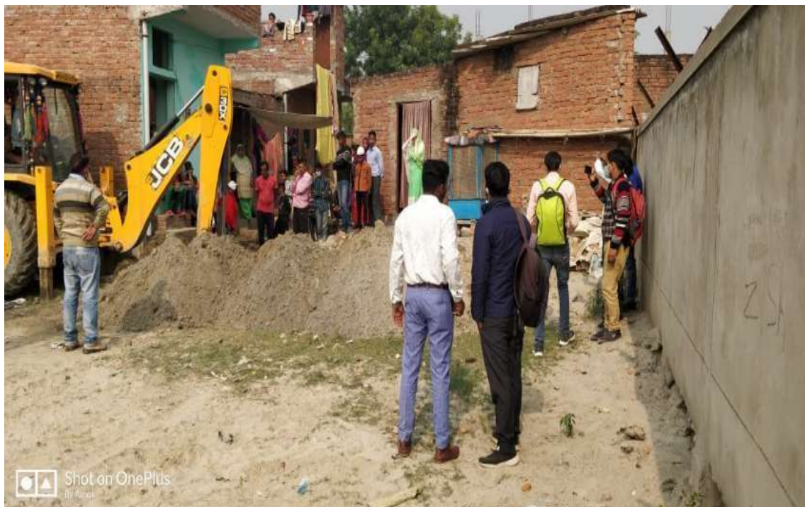
Boundary Wall excavation work
