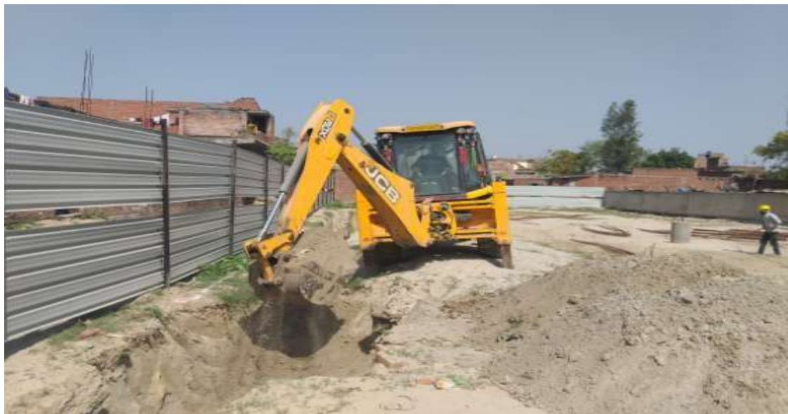
Boundary Wall excavation work
