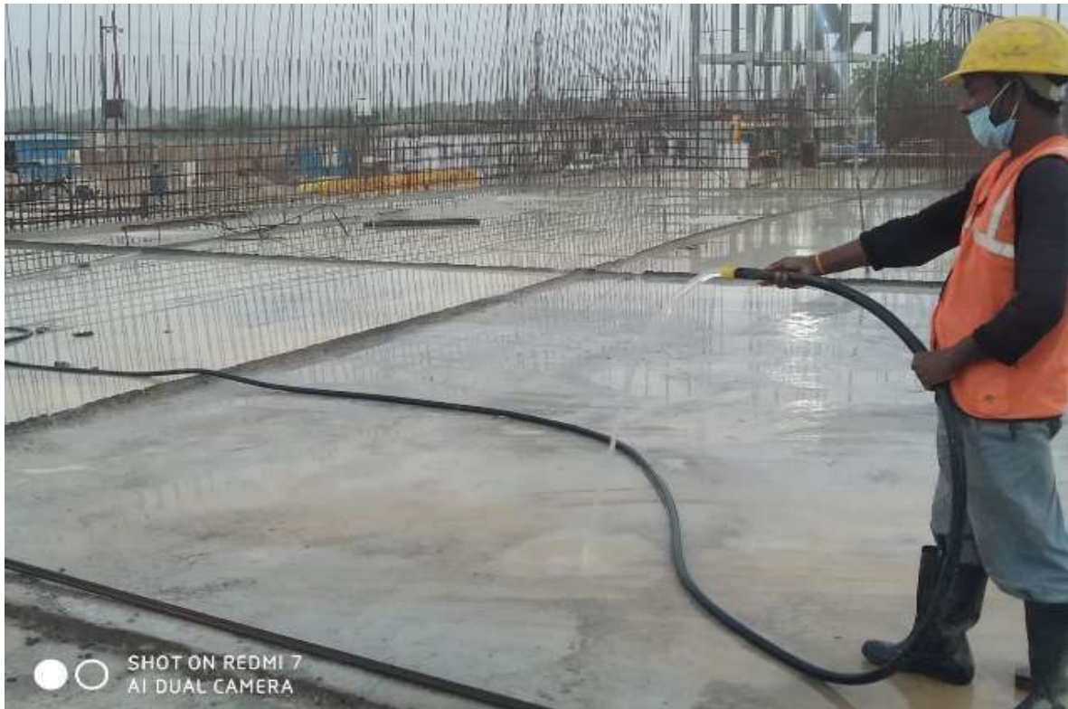
SBR floor curing
