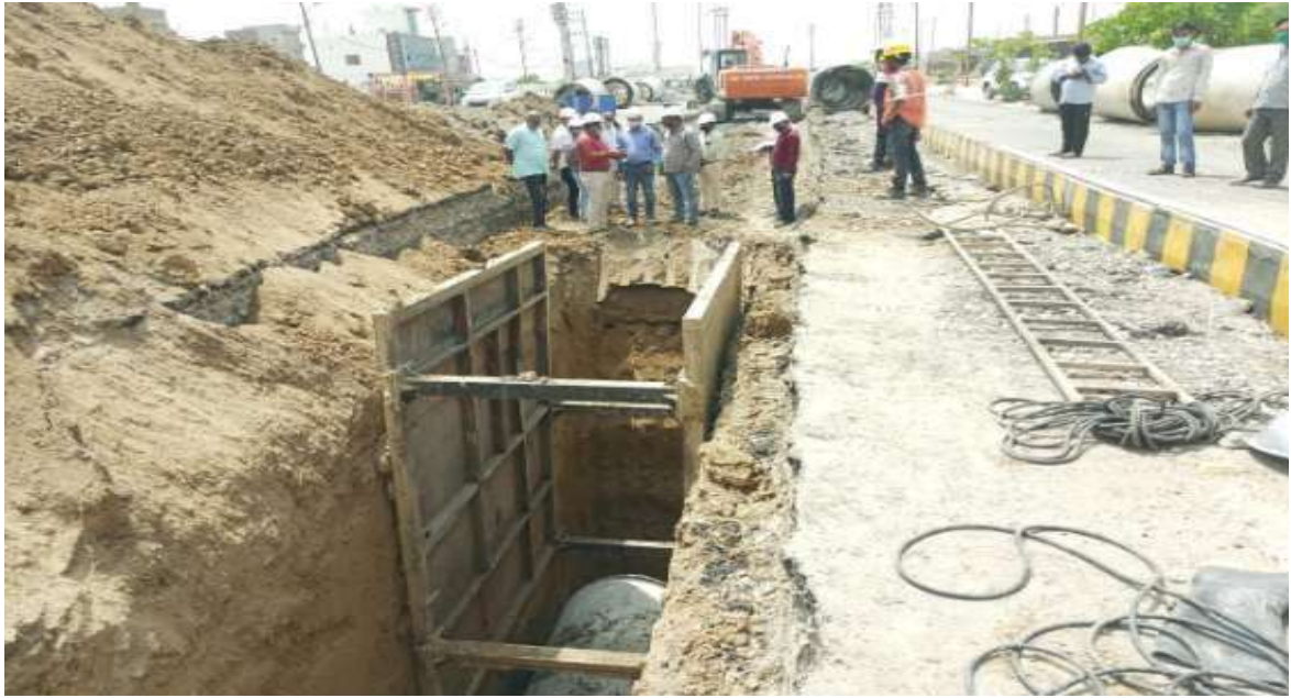
1200 dia pipe laying during GM visit
