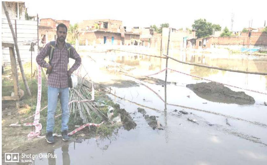
Flooding inside STP campus on 27.10.2021
