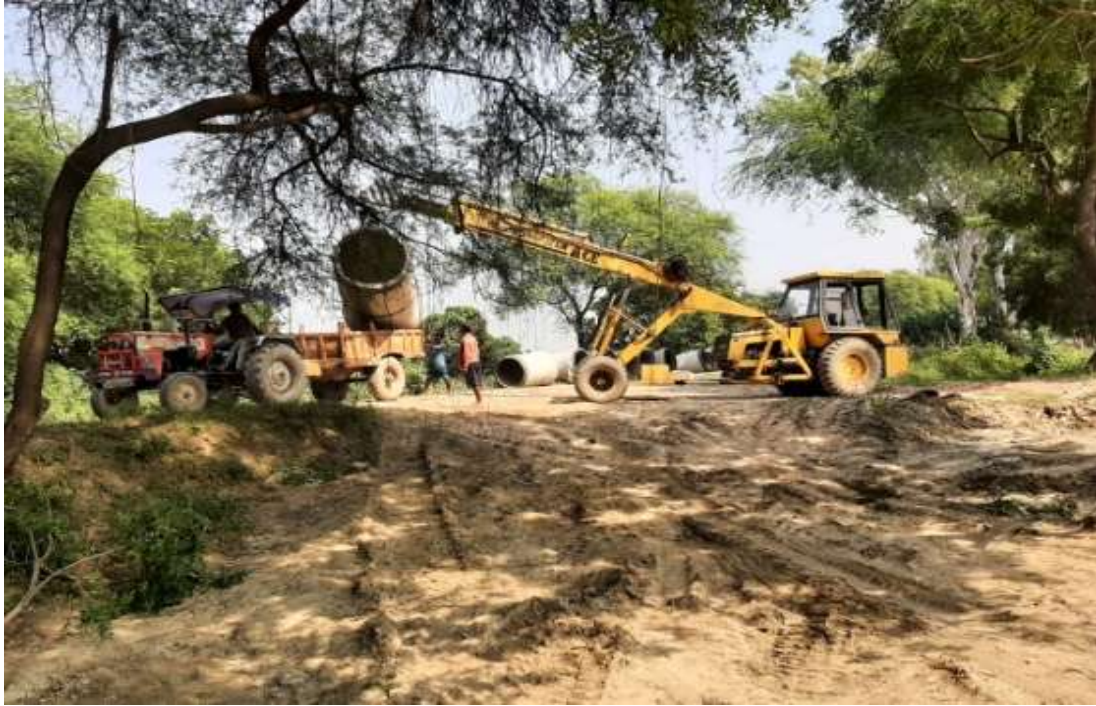
I&D site pipe shifting
