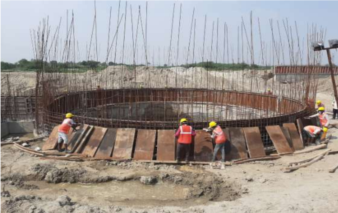
MPS shuttering & Steel binding works
