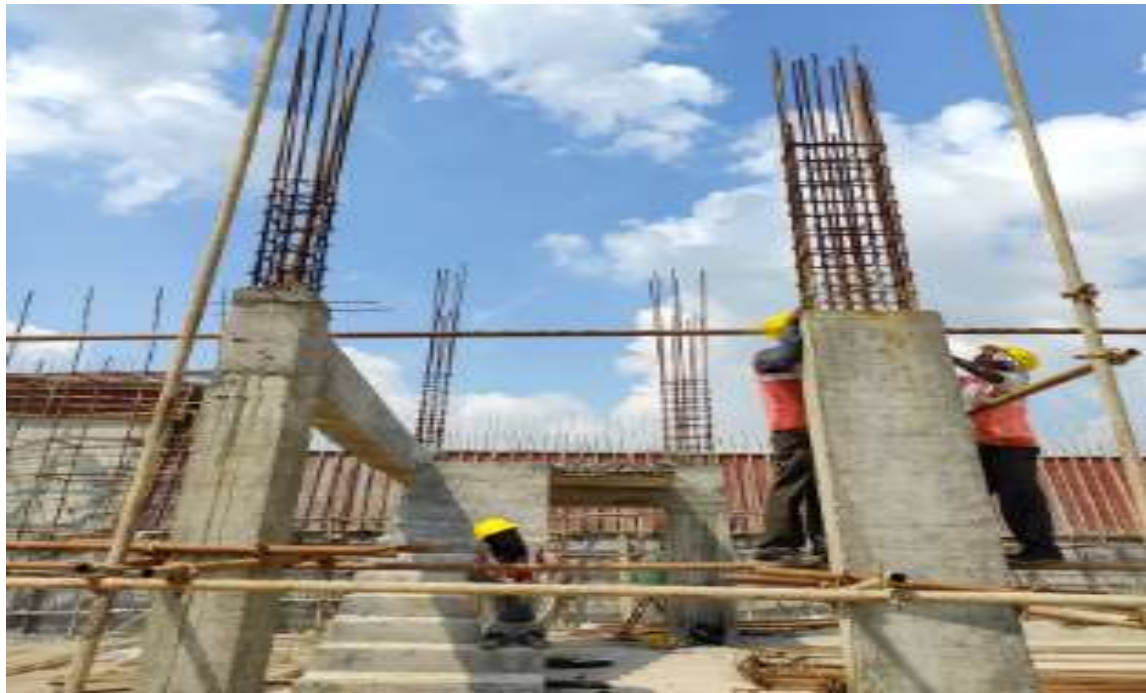
Centrifuge Building Column & Beam works
