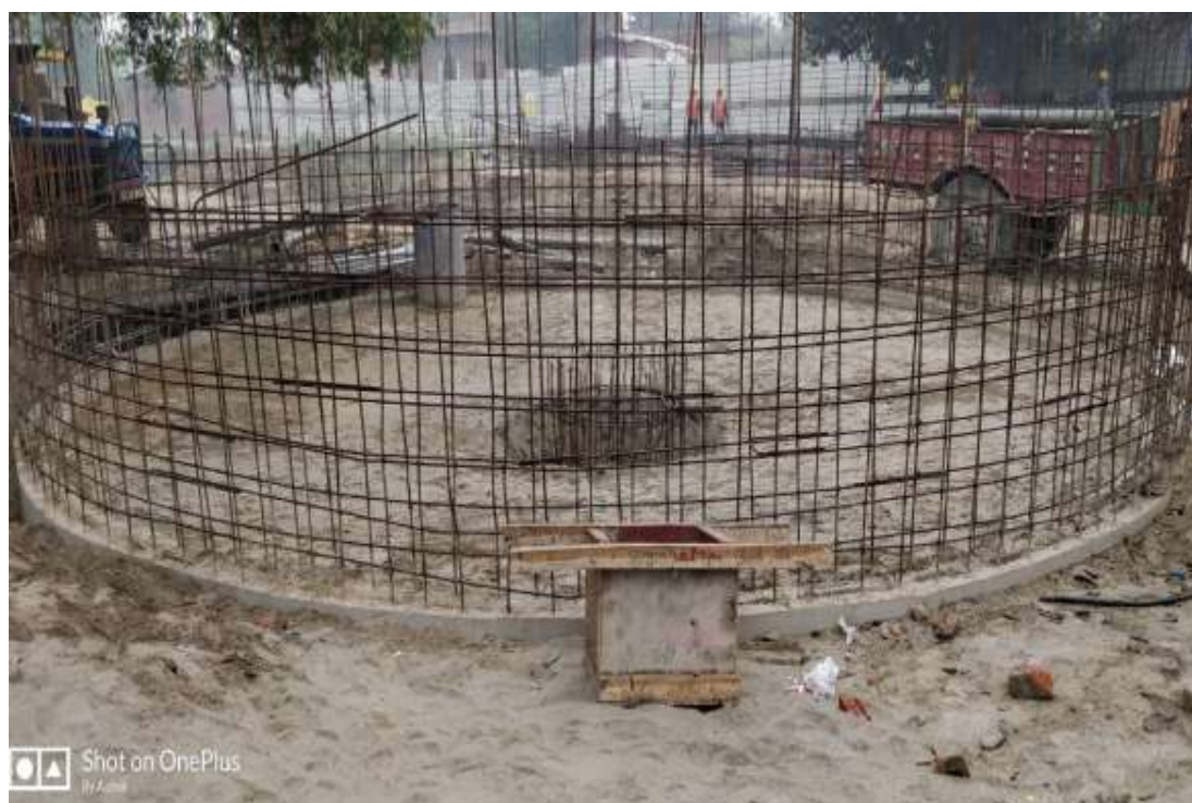
Sludge Thickener Steel Binding works
