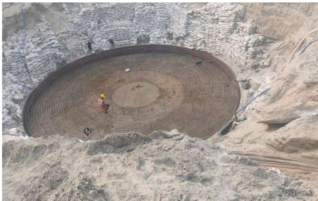
Steel binding is in progress of MPS
