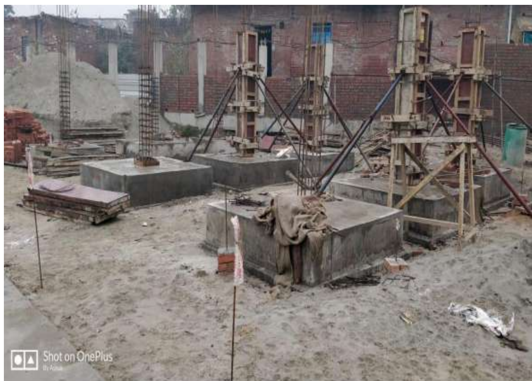
Footing of Staff Quarter & Column casting
