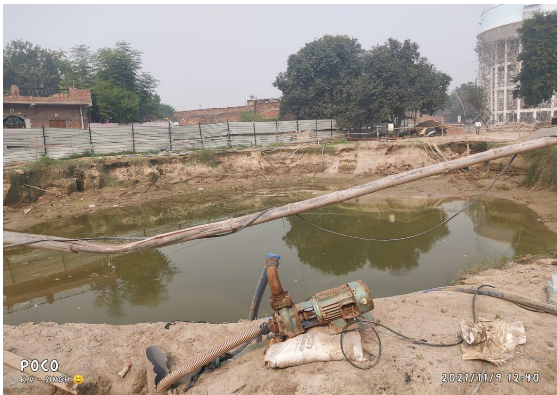
Dewatering is in progress of MPS
