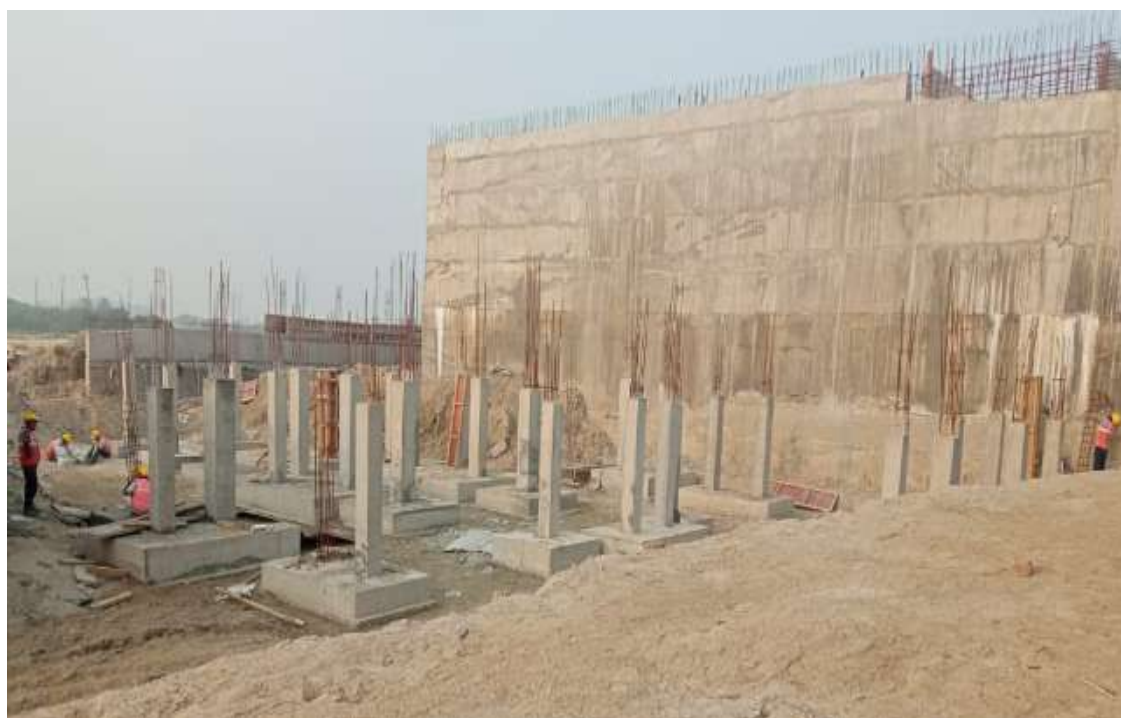
PCC, Footings and Columns 1st lift of PTU
