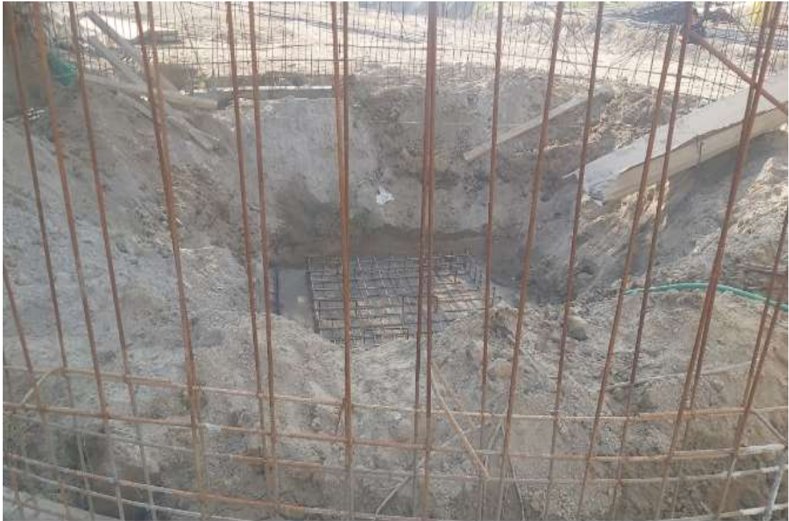
Supernatant Sump Steel binding
