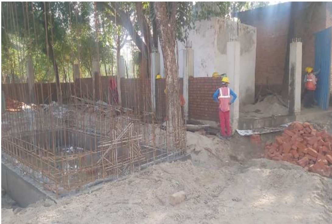
Sludge Thickener steel works
