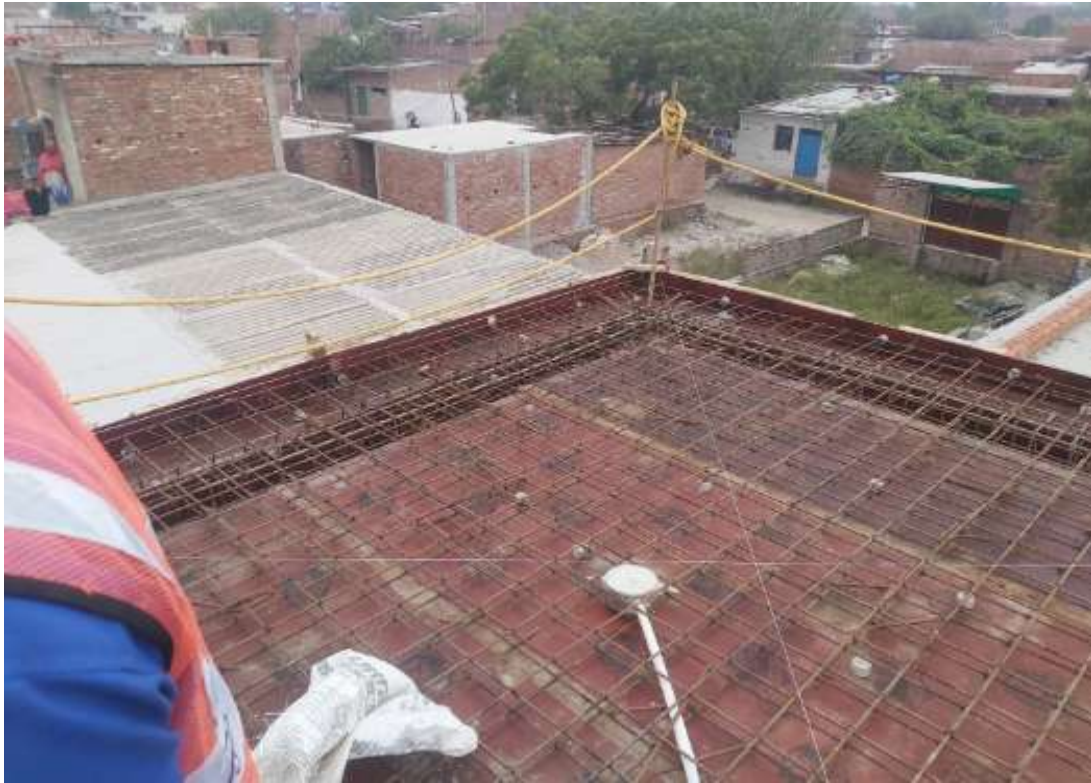
Roof Slab casting Guard Room
