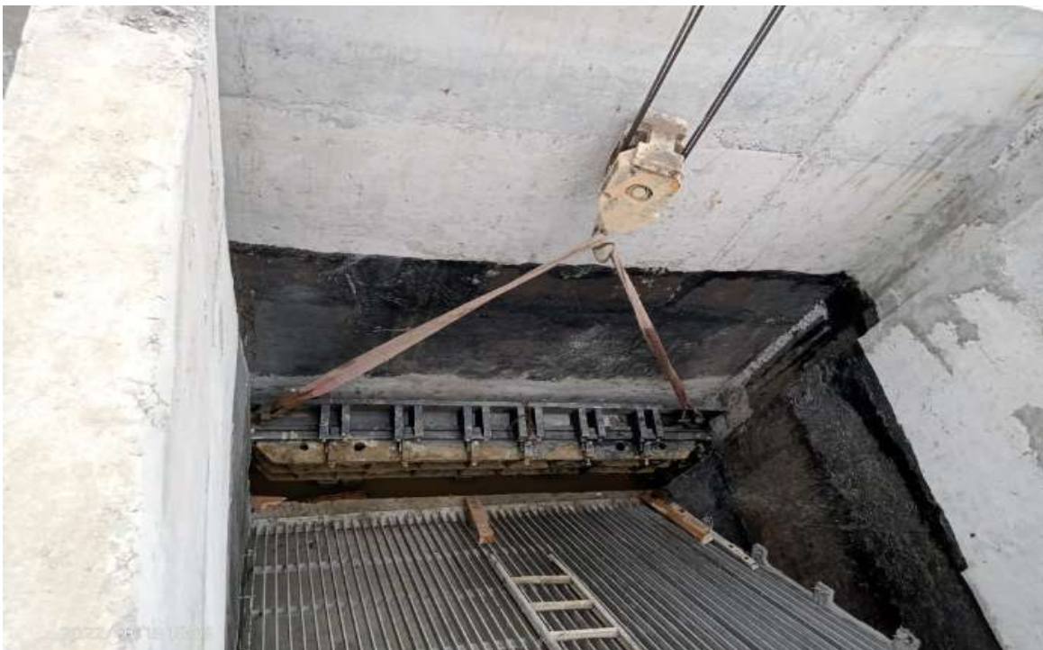
Thermal Nala A Gate Installation
