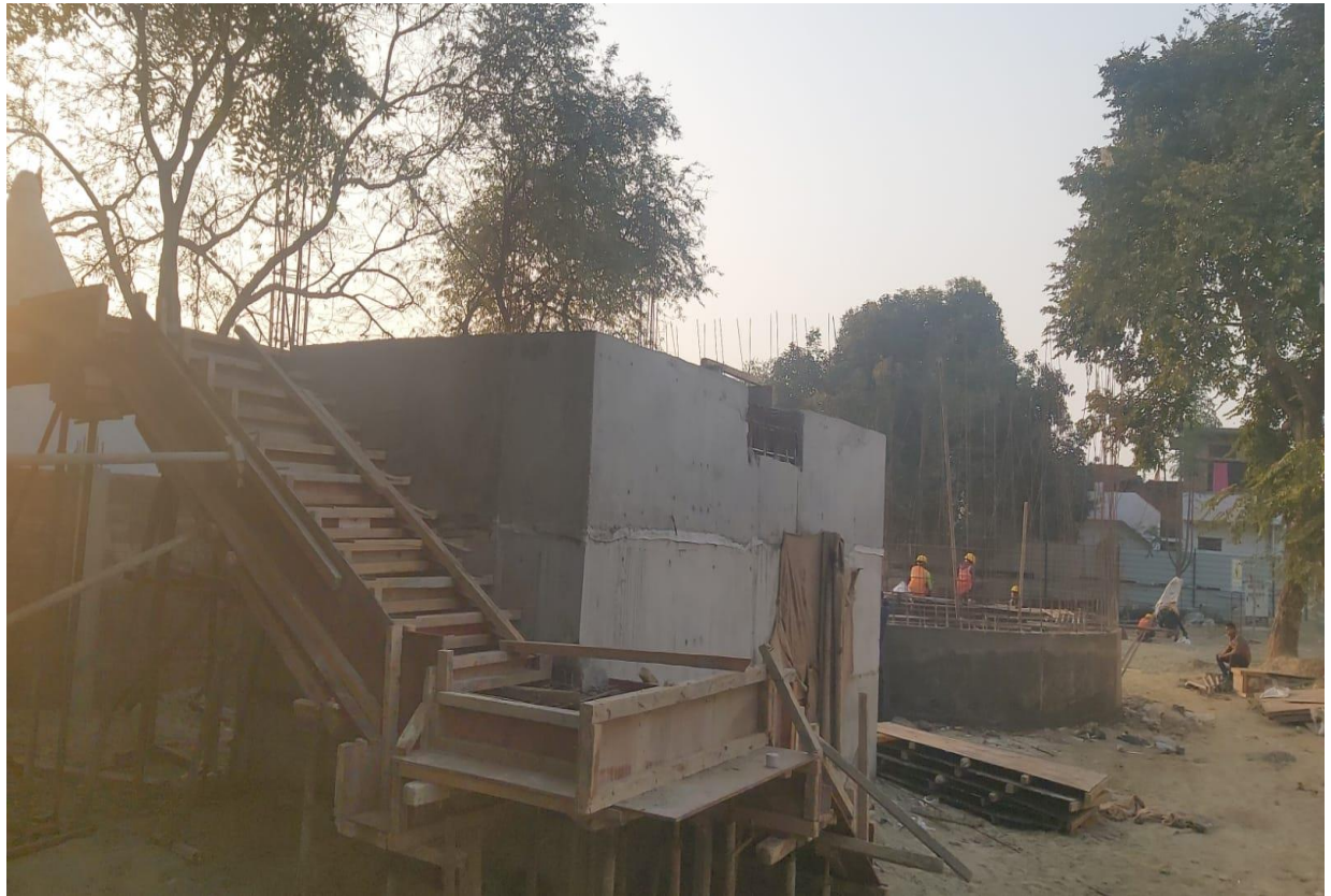
Supernatant Sump, Reinforcement of Slab and Stair is in progress
