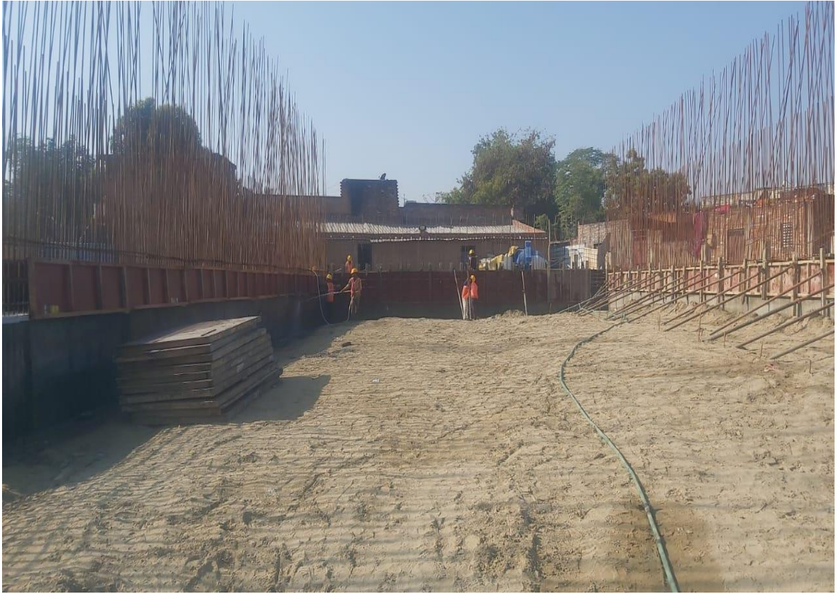
Reinforcement and Shuttering of SBR is in Progress
