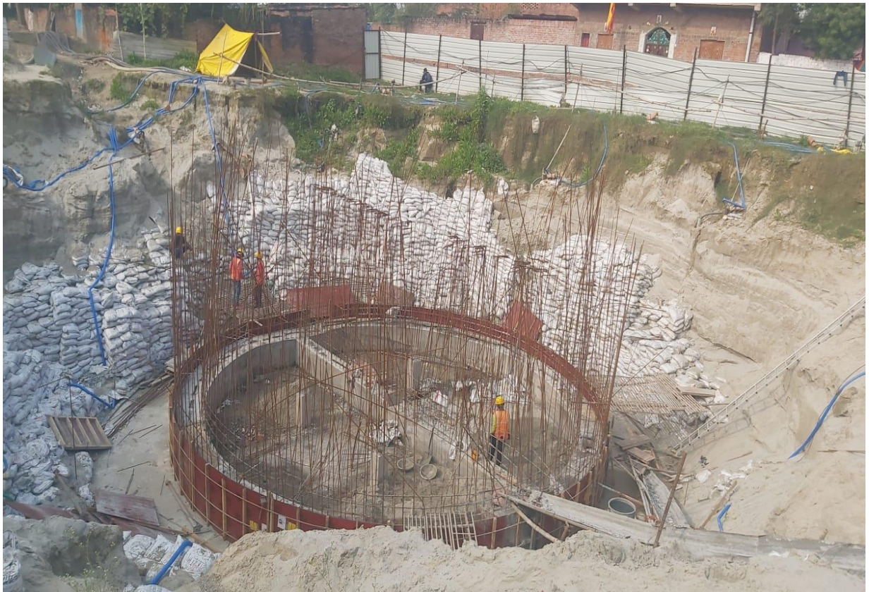
Steel binding is in progress of MPS
