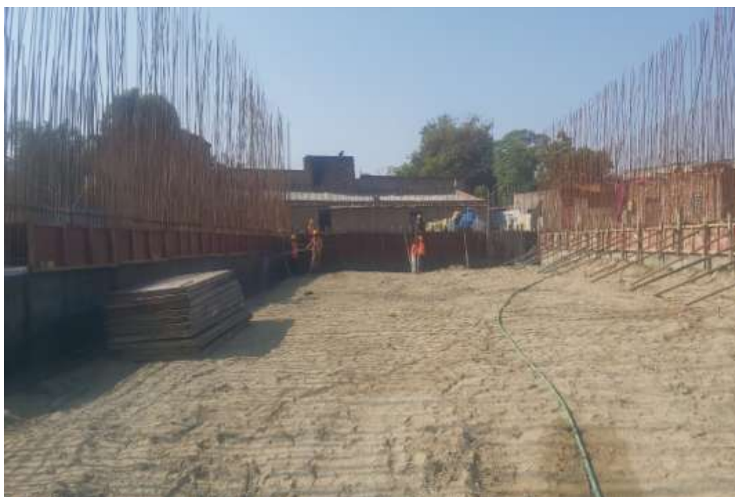
SBR wall Steel binding work
