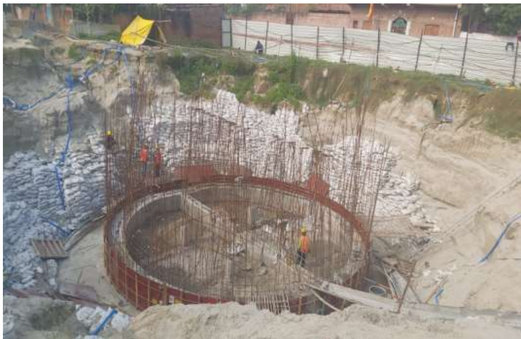
Steel binding is in progress of MPS
