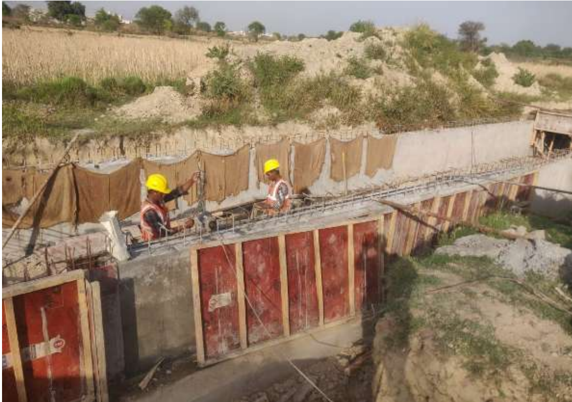
I&D wall de-shuttering works
