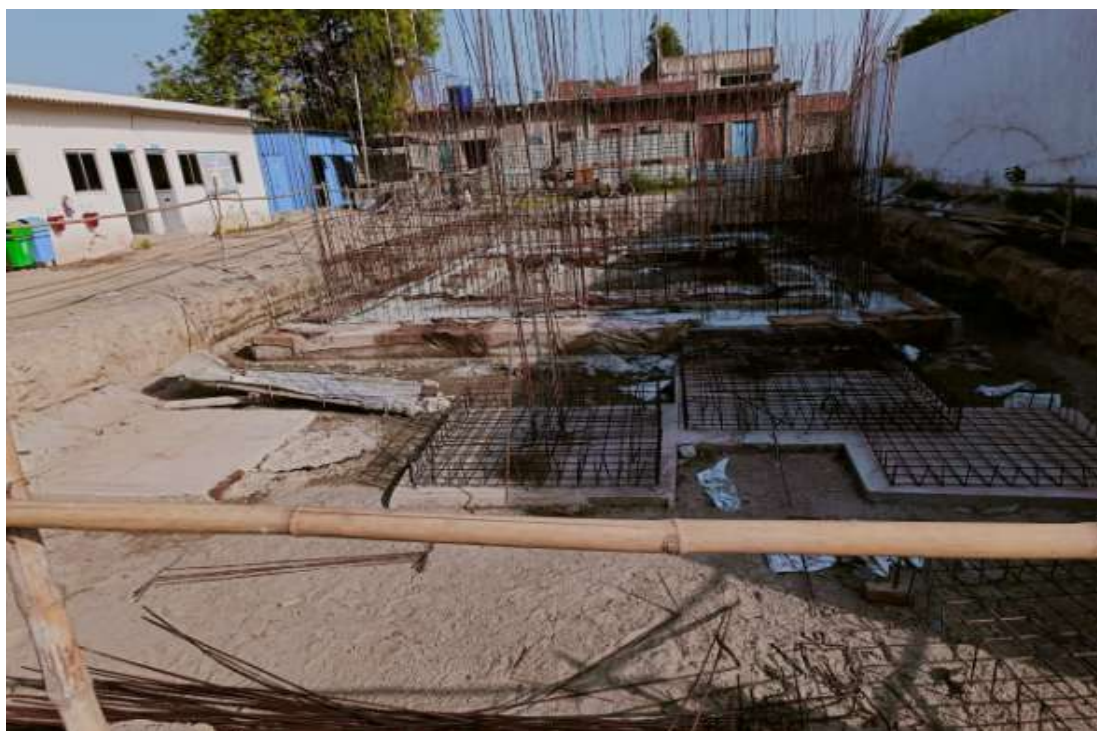
Steel binding is in progress of CCT
