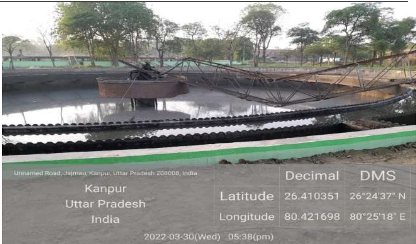
FST 01 under renovation,Mechanical bridge collapsed on 15.01.2022
