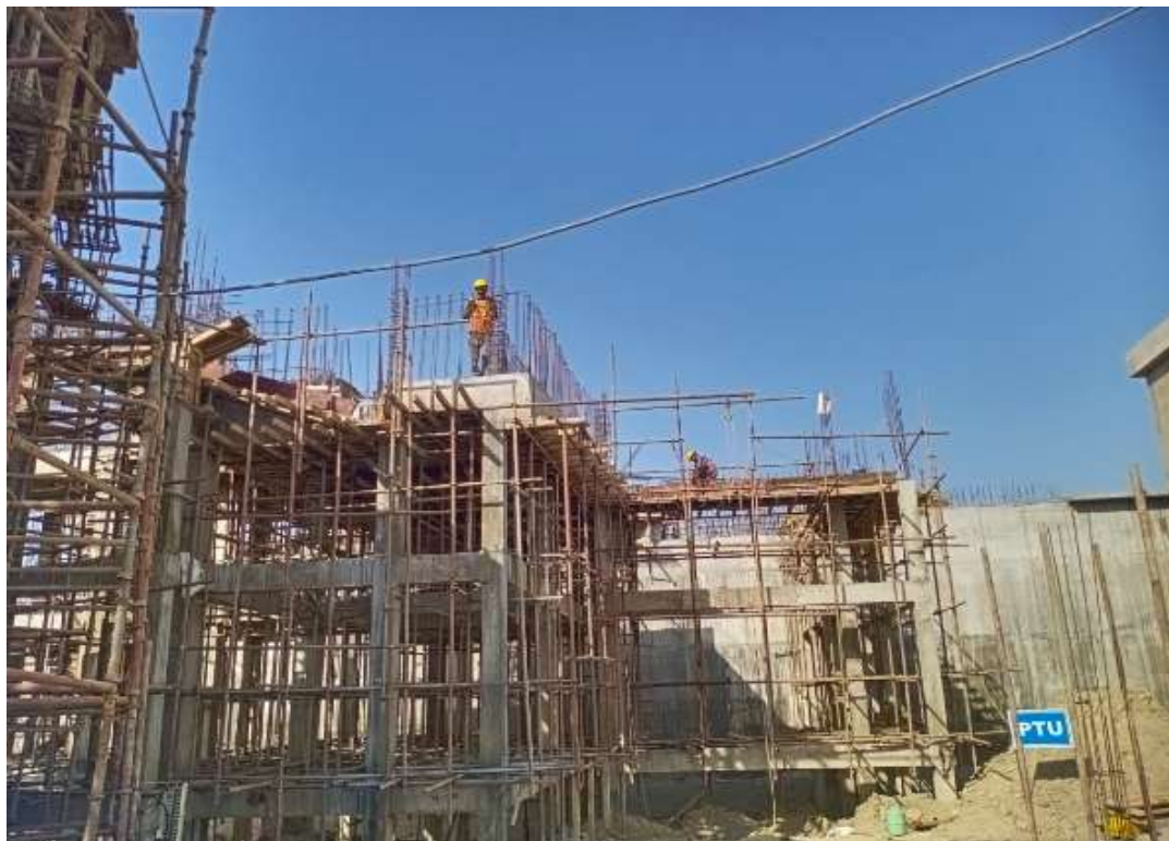
Shuttering and reinforcement work in PTU
