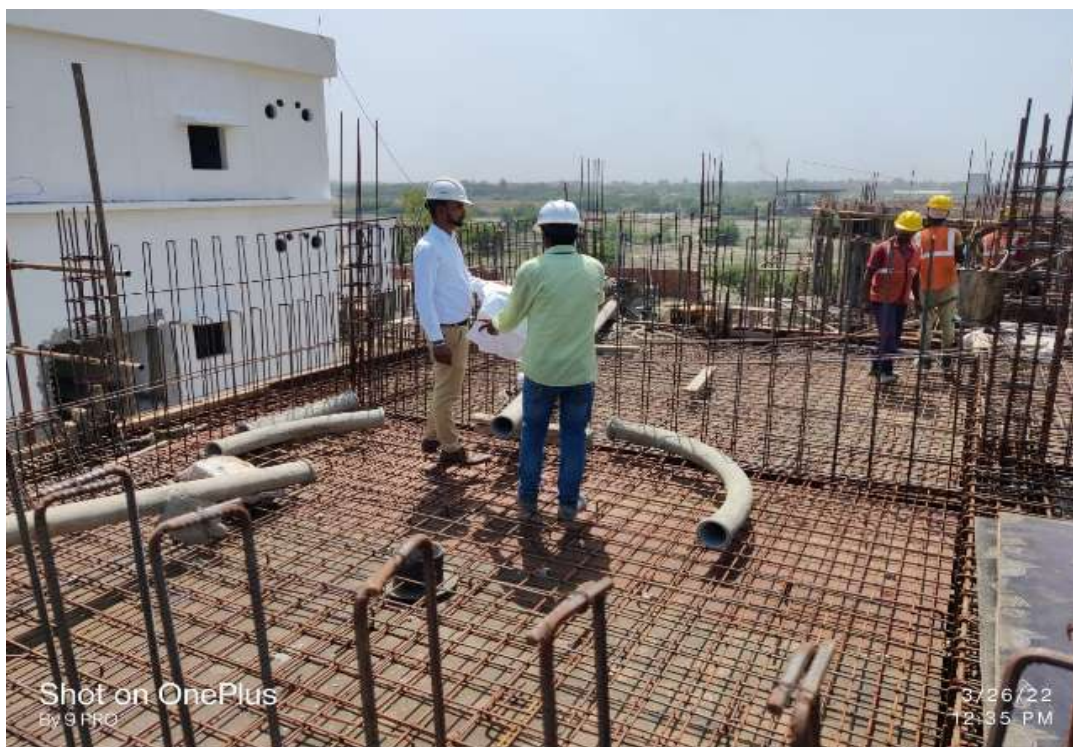
Casting of roof slab of PTU Grit Chamber
