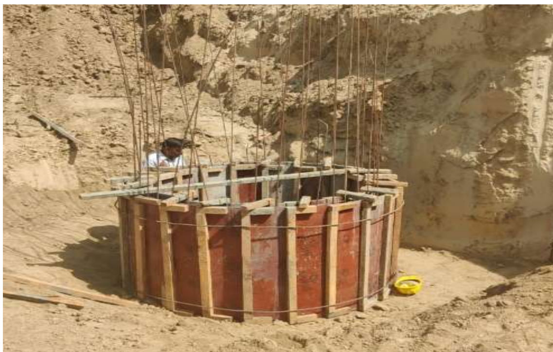
Manhole casting works
