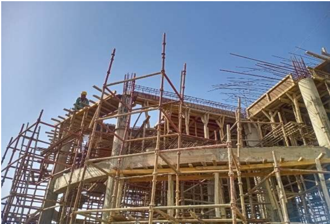
I&D wall de-shuttering works
