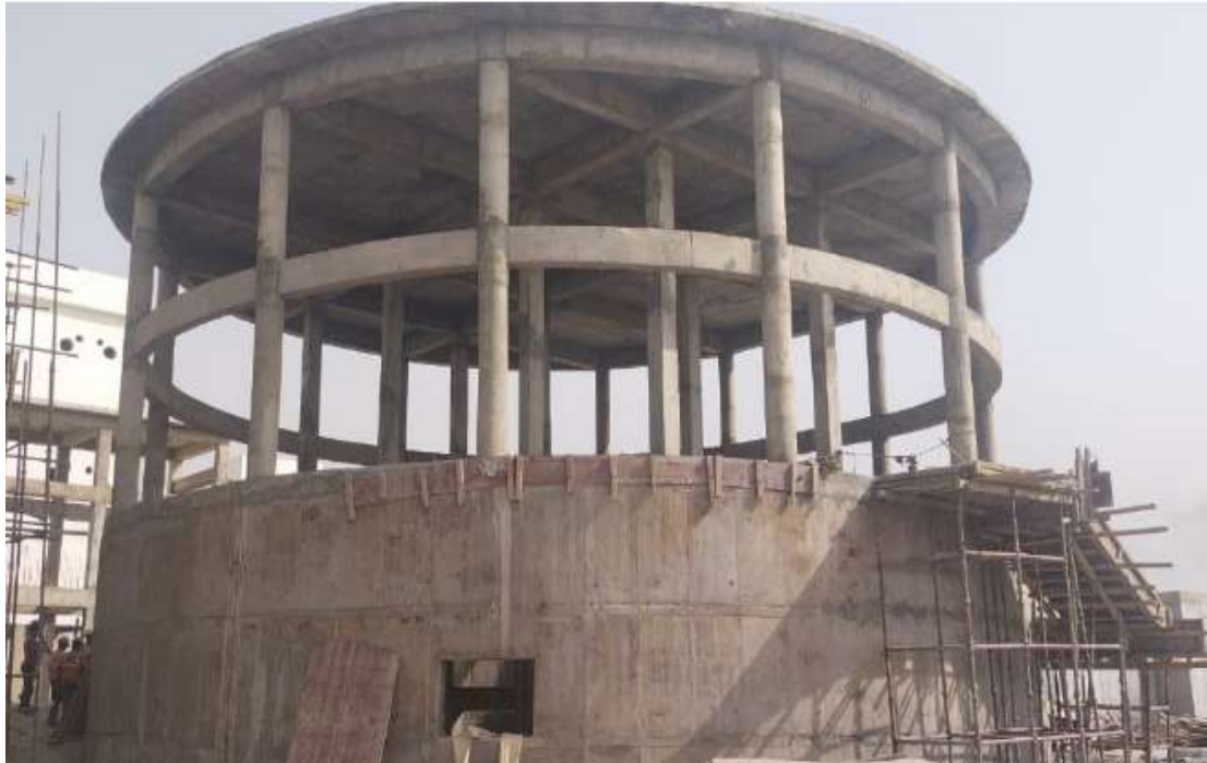
MPS de-shuttering work
