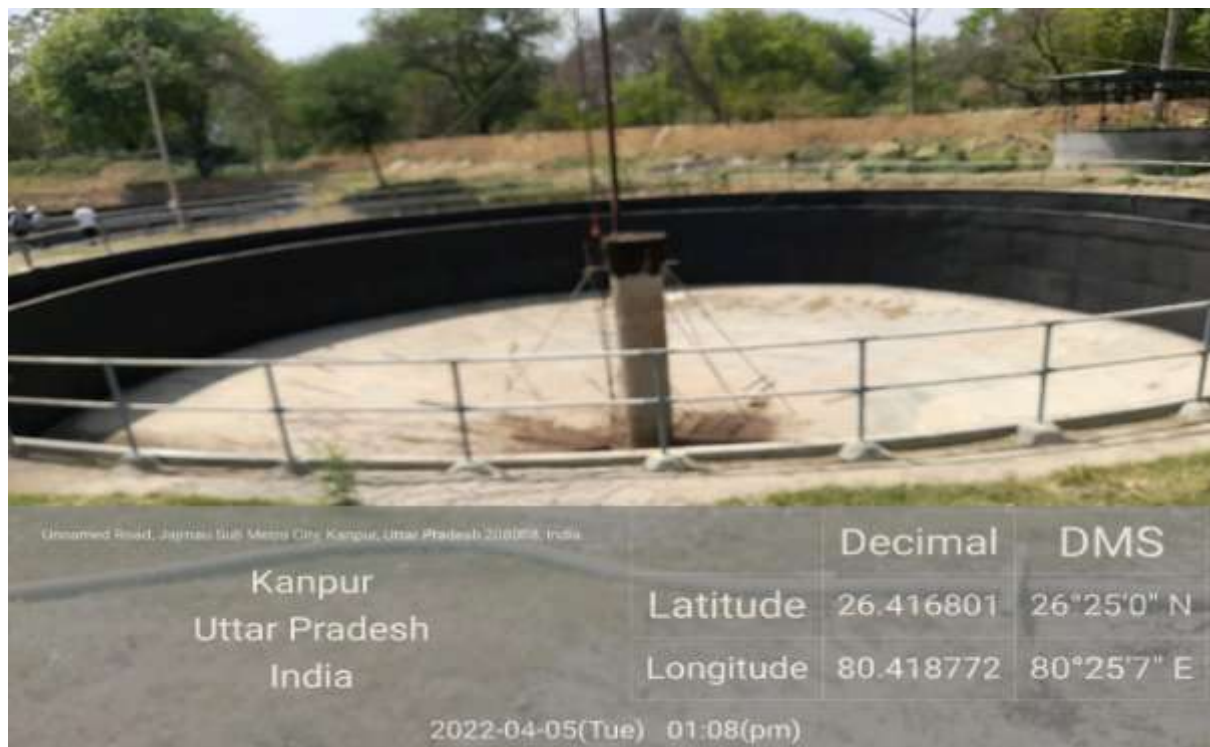
Sludge thickener 01&02 is in under renovation
