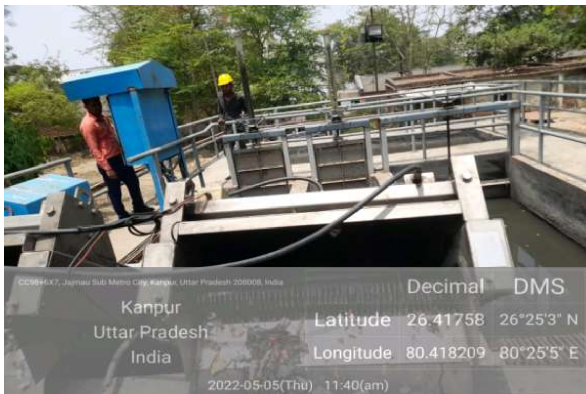
Mechanical fine screen under O&M
