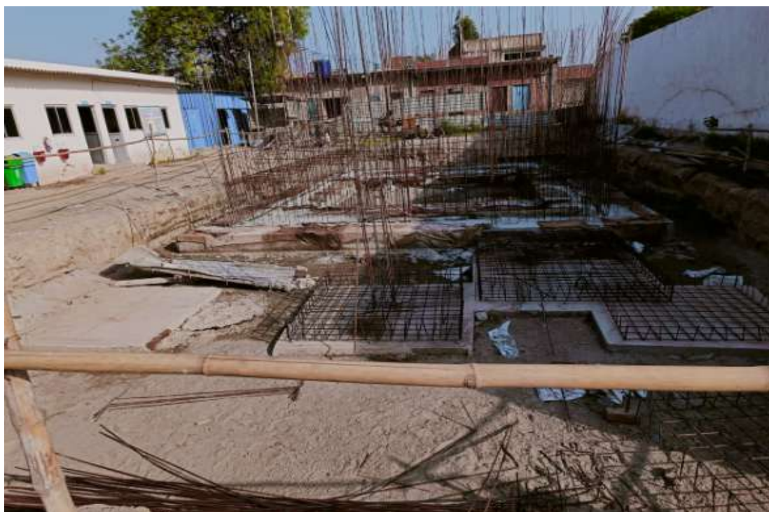
Steel binding is in progress of CCT
