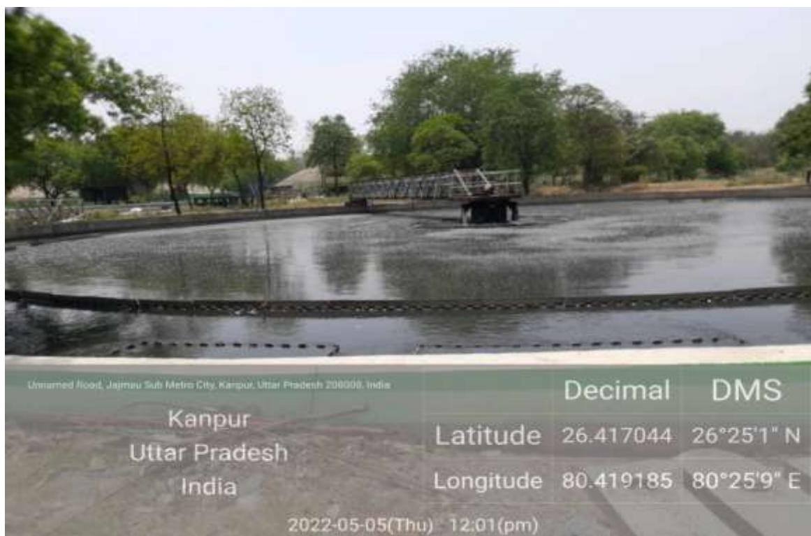
Primary sedimentation tank under O&M
