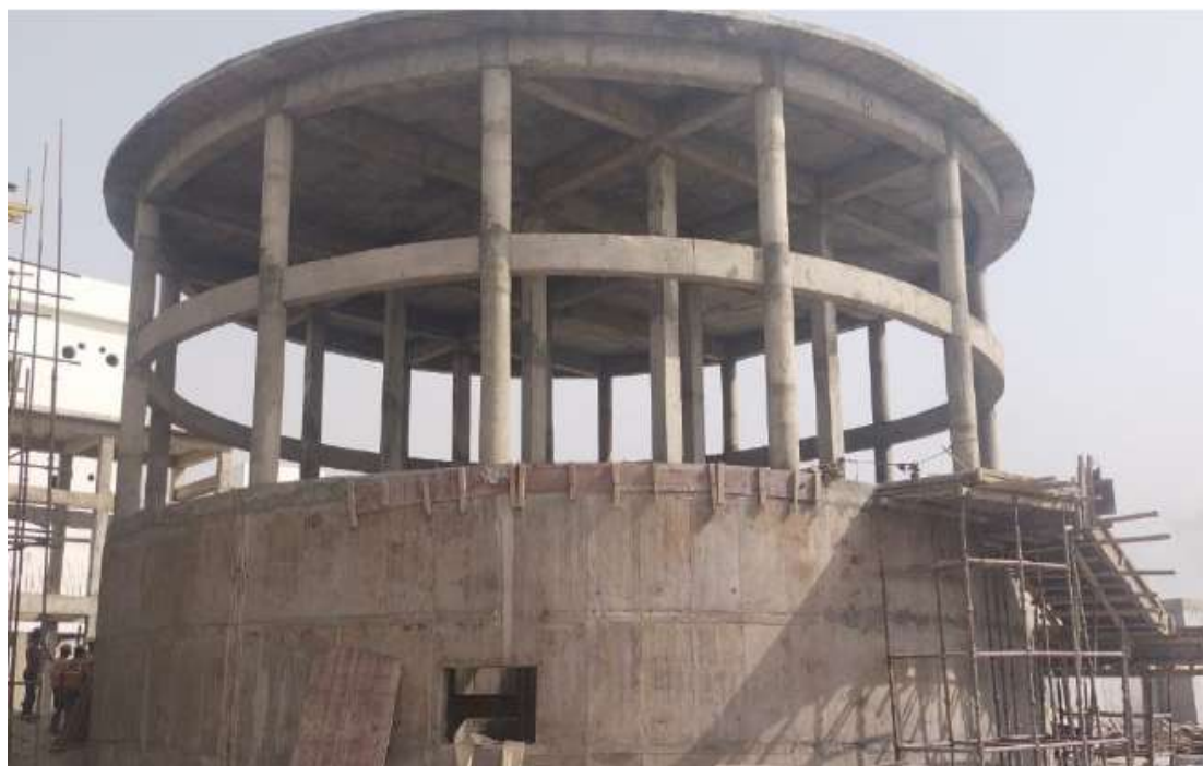
MPS de-shuttering work
