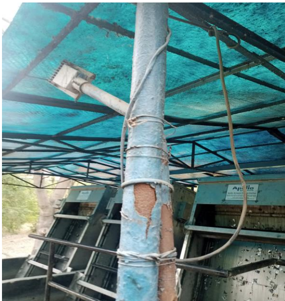
PTU Shed Corroded
