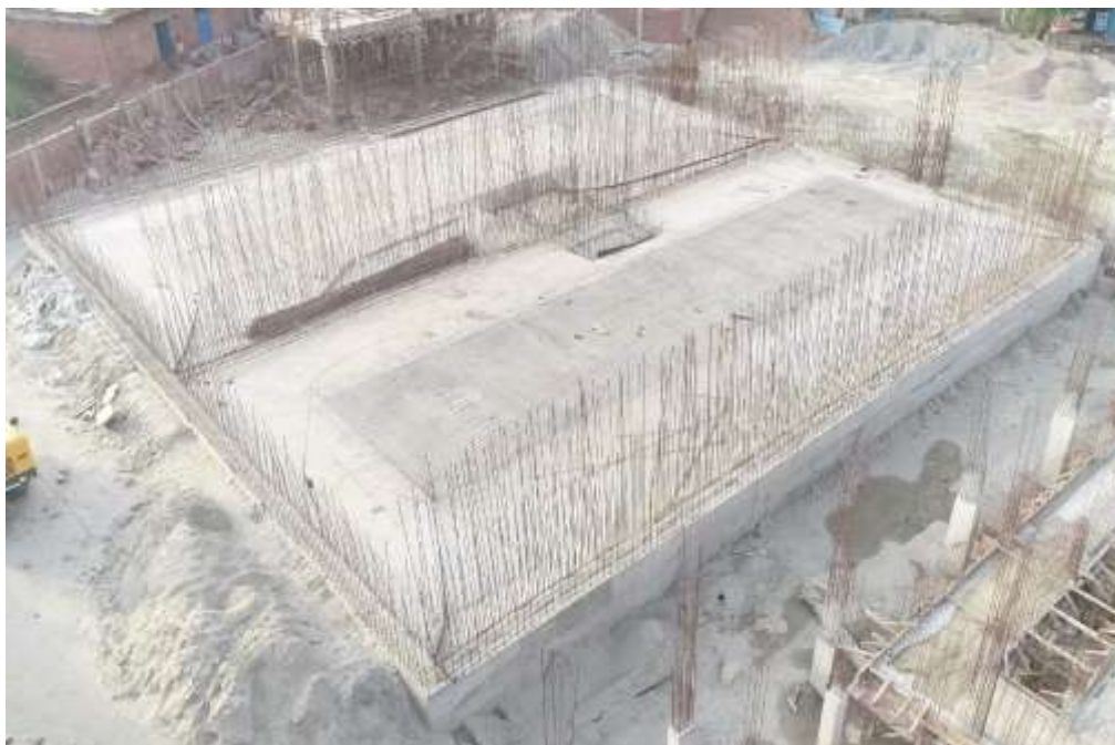
SBR floor & steel works
