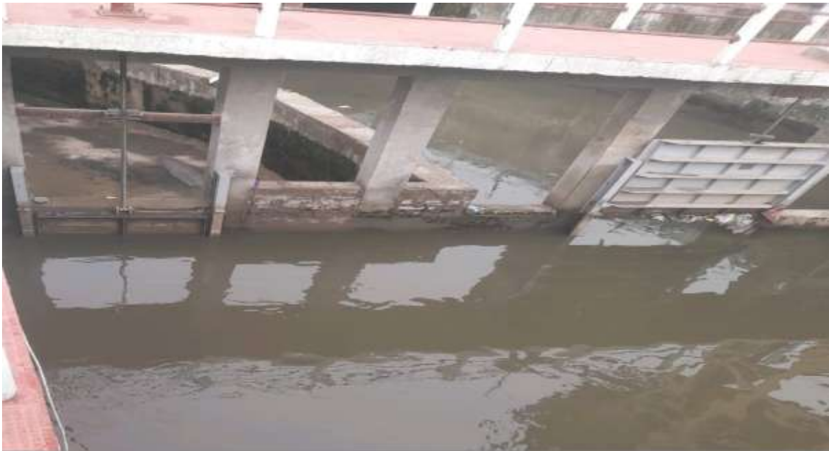
Over flow condition happens during peak hour at Shishamau IPS
