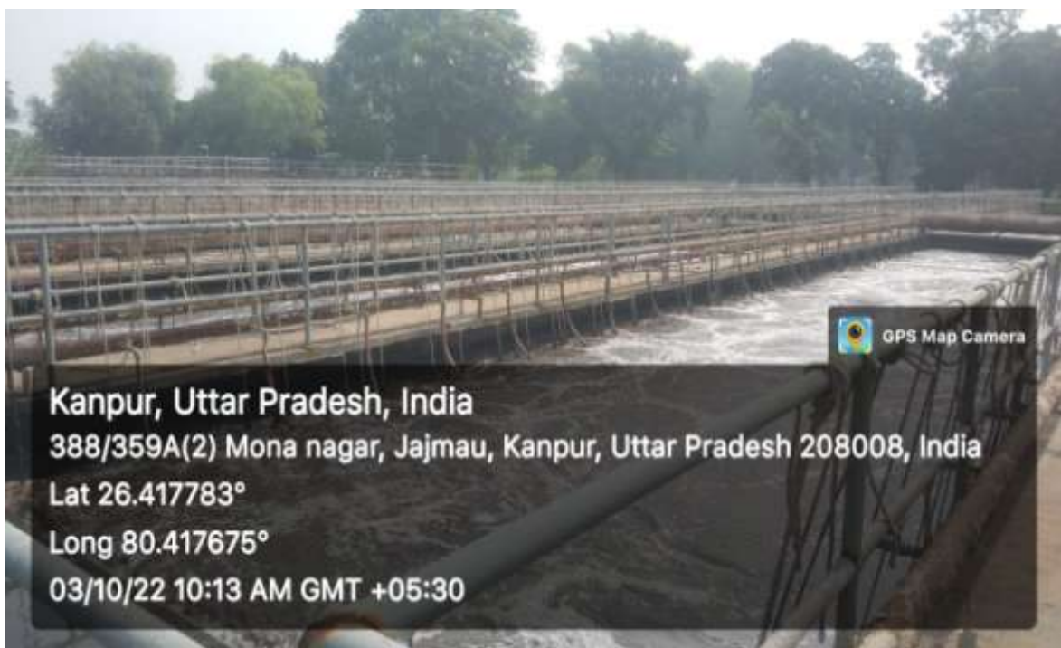
Aeration tank under operation of 43 MLD STP Jajmau
