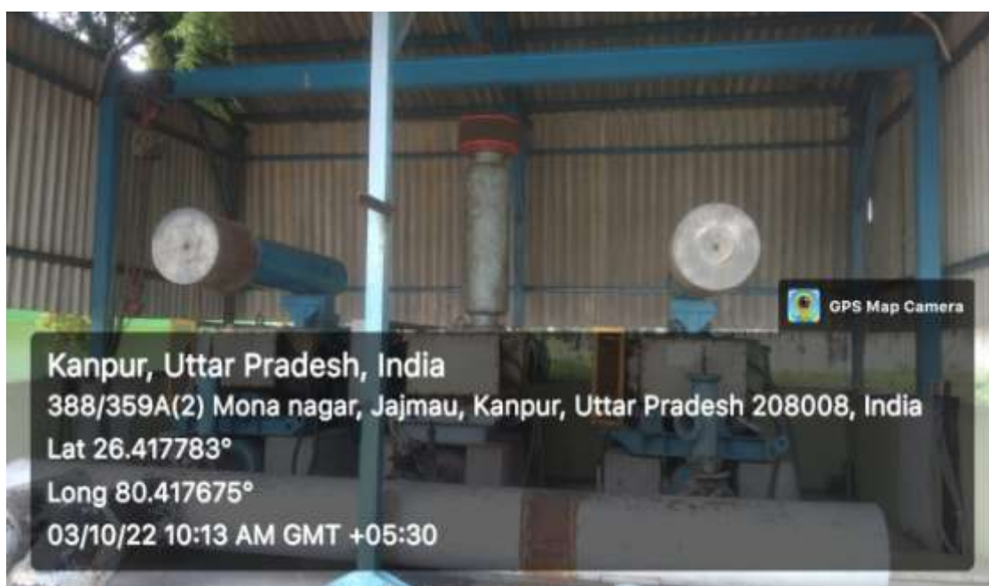
Only 2 out of 3 nos. Air blower under operation of 43 MLD STP Jajmau
