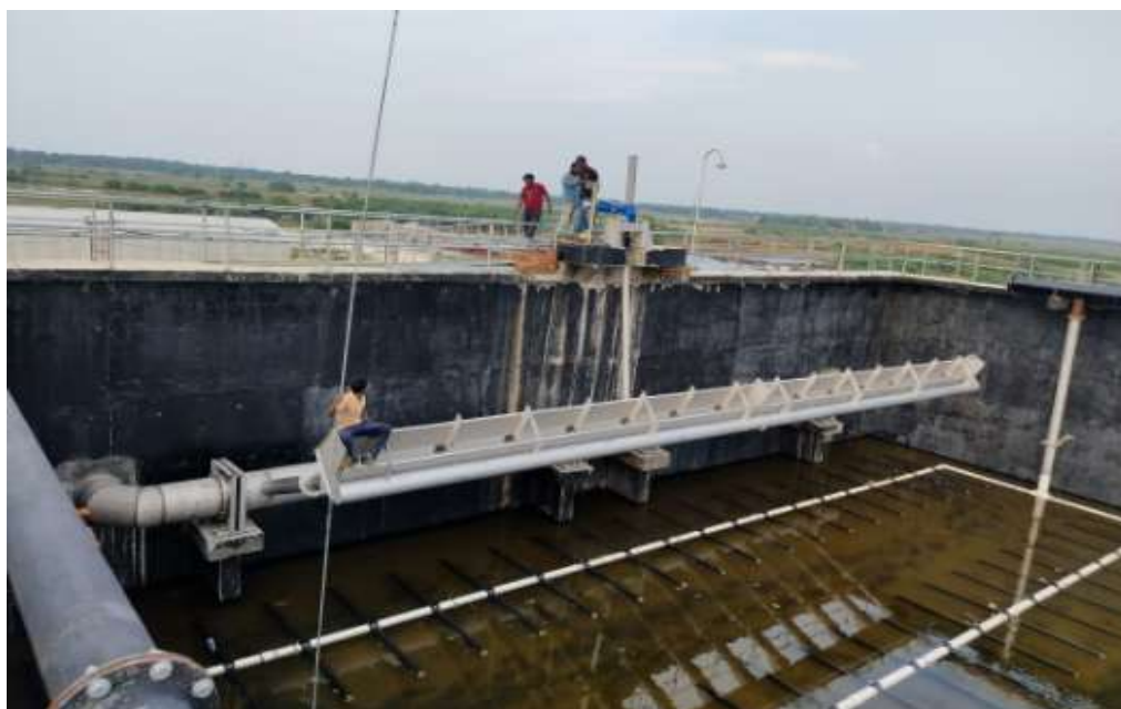
Decanter Installation & Testing
