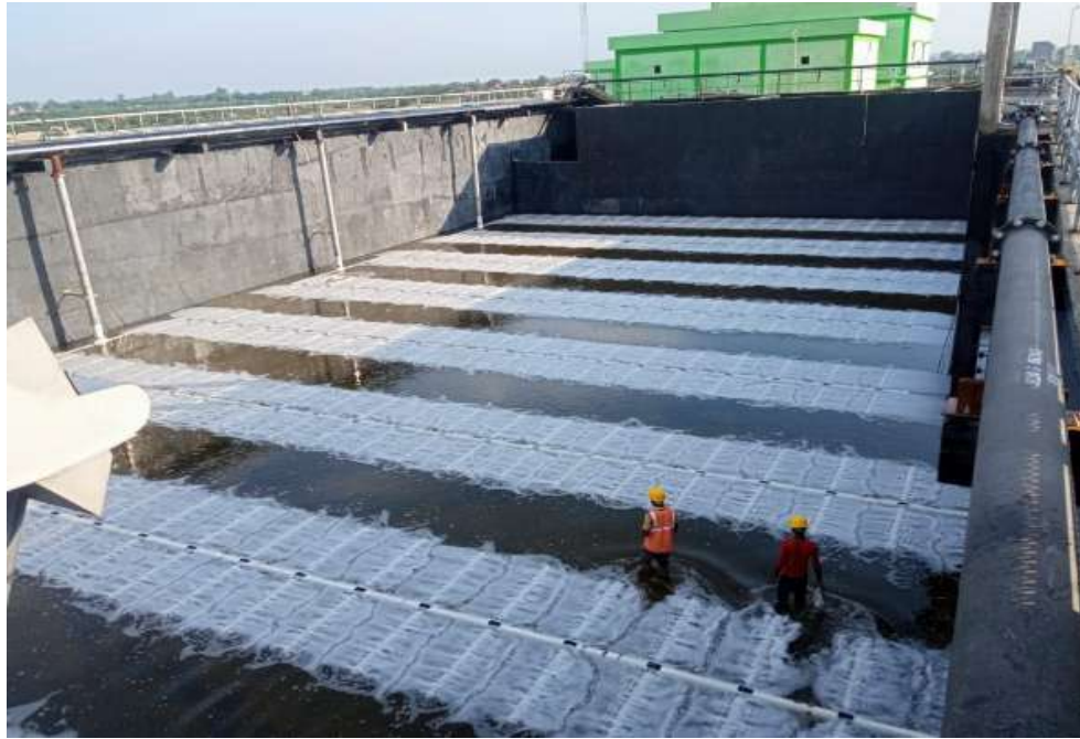
Diffuser leakage testing done
