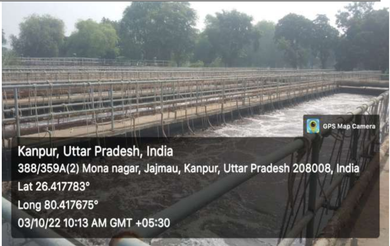
Aeration tank under operation of 43 MLD STP Jajmau
