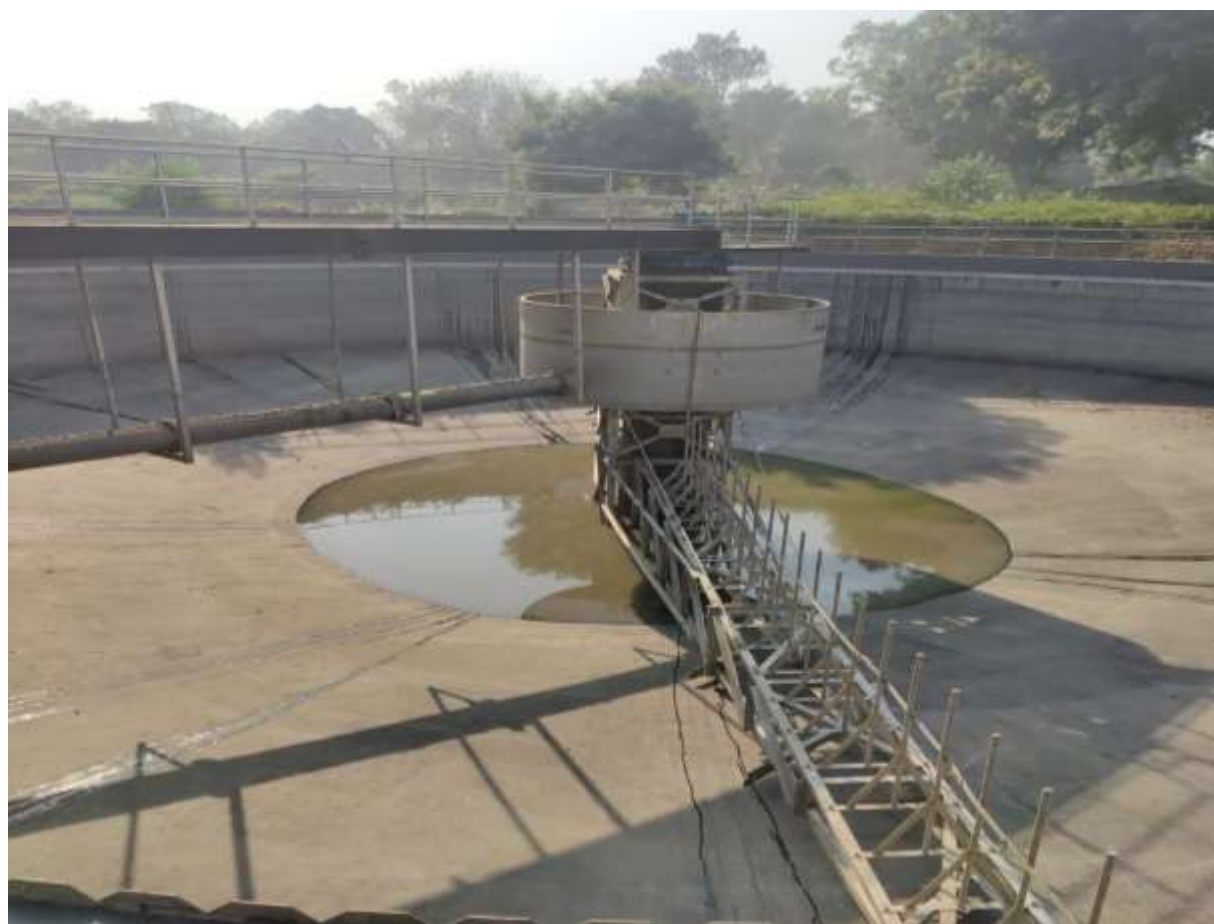
Renovation of Sludge Thickener in November 2022
