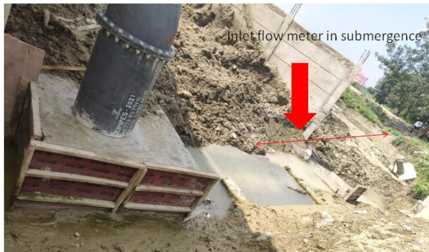
Fig 18a: Inlet Flowmeter – Submerged condition on 03.11.2022
