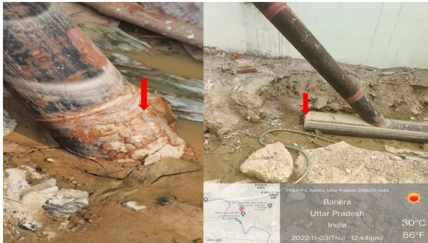
Fig 5: Heavy corrosion in the blower discharge line
