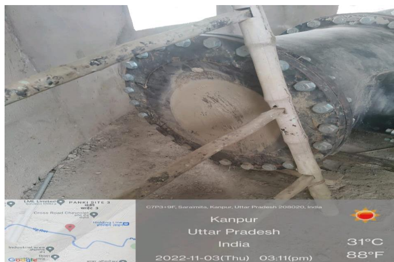
Fig 13B: Discharge pipeline Blind Flange Installed incorrectly at ICI pump house
