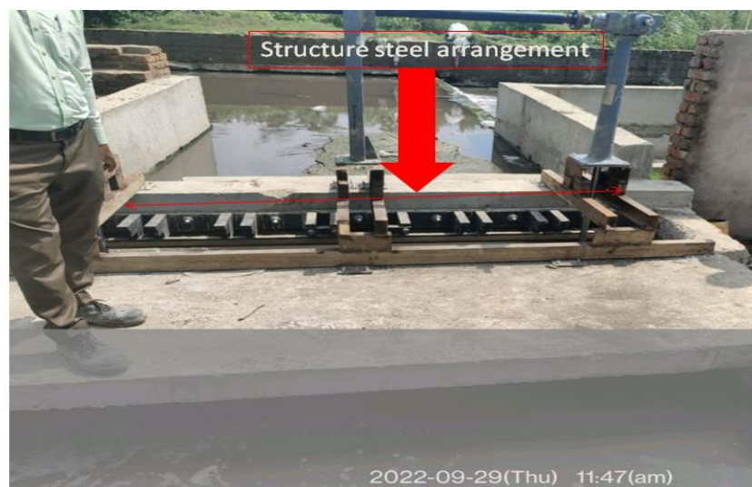
Fig 8: Weir Sluice gate (Size 3000X500mm)
