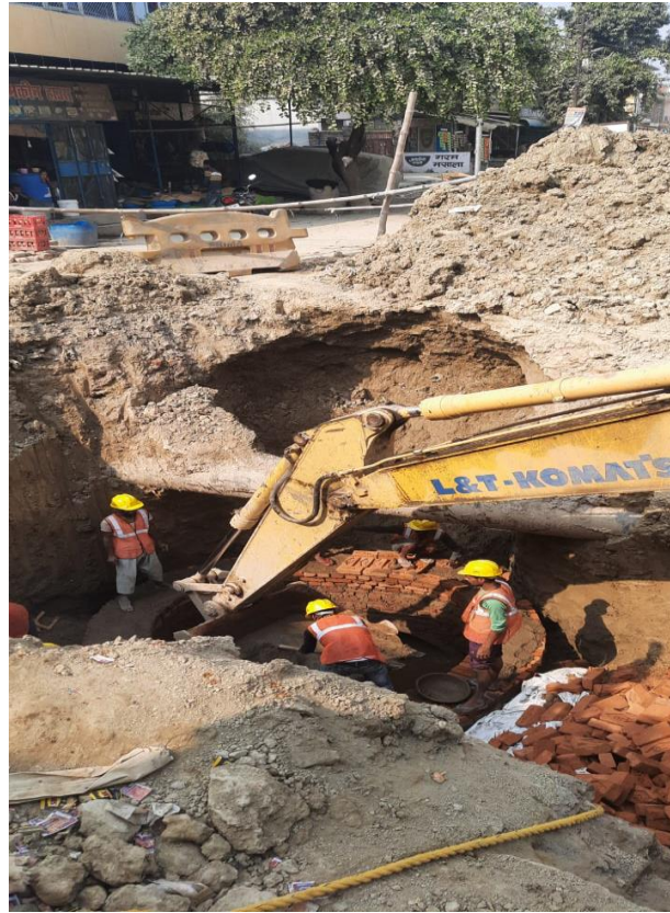
Fig 7: Manhole construction without safety arrangements (barricading, shoring, etc.) near 4 ATM Tiraha, Gangaganj, Pankhi, Kanpur
