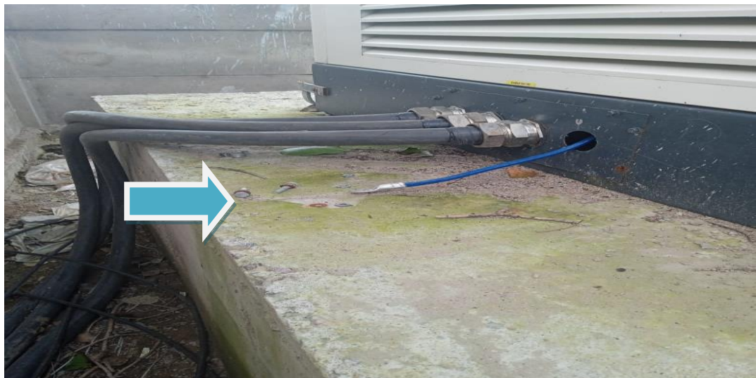
Fig 20: DG set earthing not done properly
