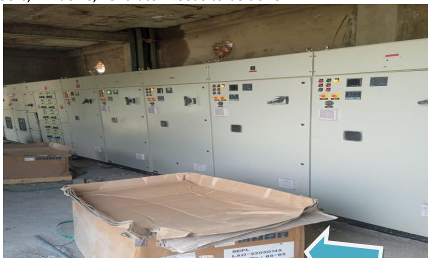
Fig 22: LT Panel charged without VFD starters and control functioning not proper
