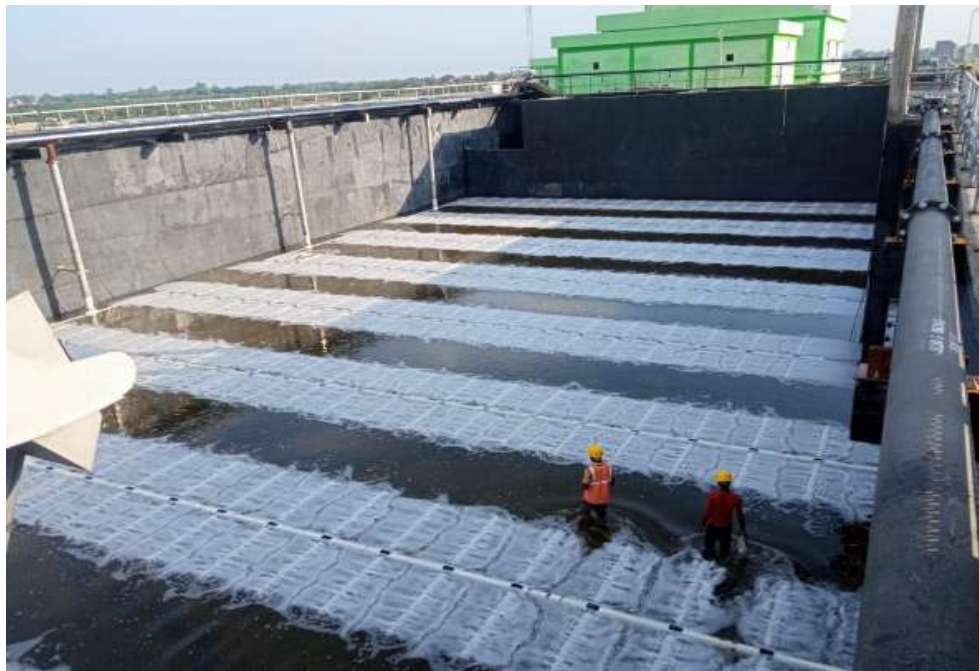
Diffuser leakage testing done
