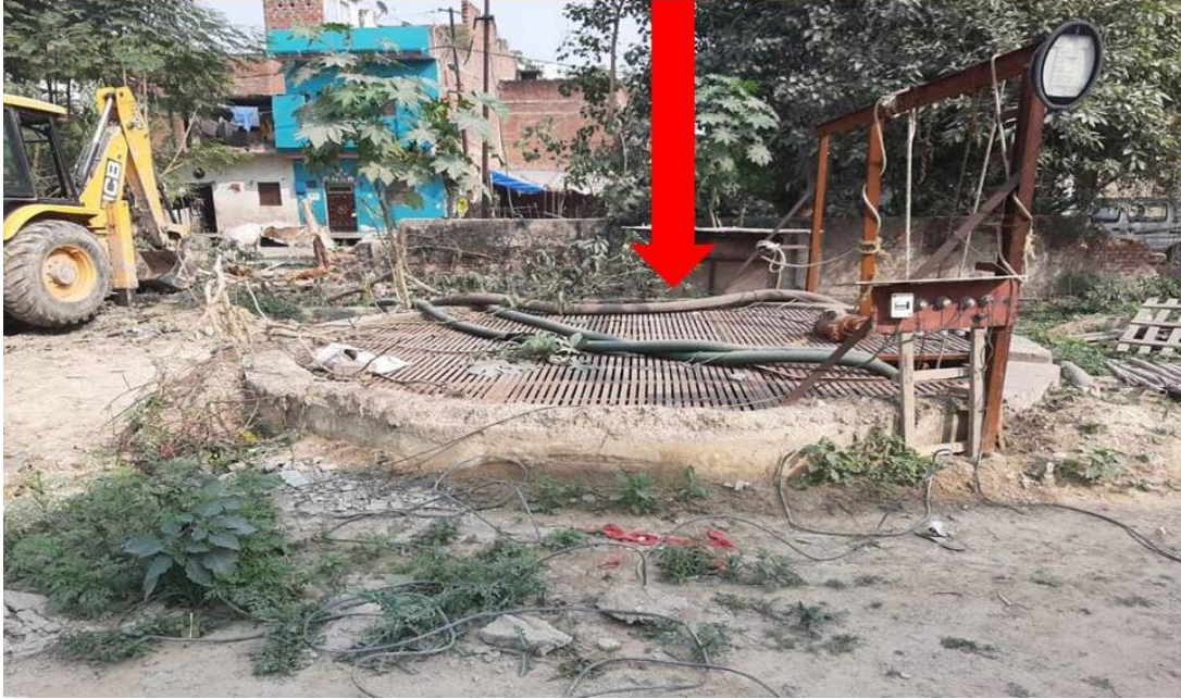
Fig 25: Existing wetwell at Sundar Nagar
