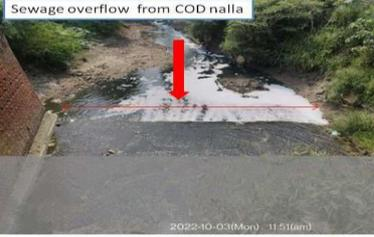
A photograph showing a concrete channel with a large amount of sewage overflowing onto the ground. A red arrow points to the overflow. The date and time '2022-10-03(Mon) 11:51(am)' are visible at the bottom of the photo. | Required nos. of pumps at MPS need to be operated to tackle the problem of overflow.                                                                                                   |                                      | 03.10.2022
