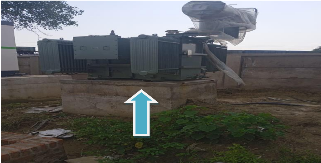
Fig 21: Transformer placement on foundation is not proper
