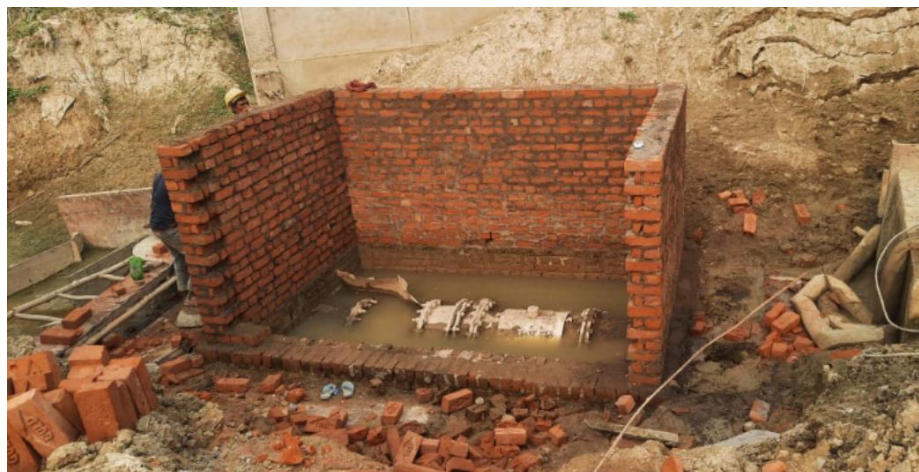
Fig 18b: Inlet Flowmeter – Submerged condition on 07.11.2022 and within unapproved brick chamber under construction
