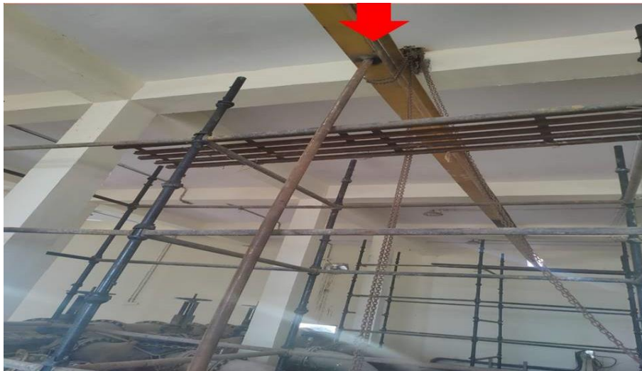
Fig 2: Monorail Installation
