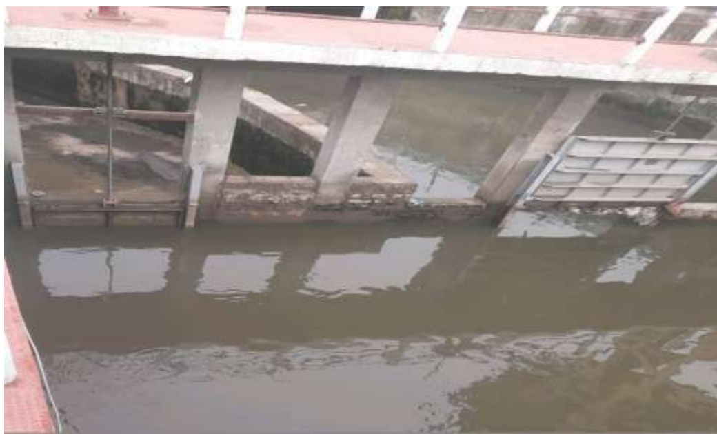
Over flow condition happens during peak hour at Shishamau IPS
