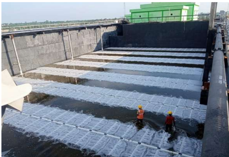
Diffuser leakage testing done
