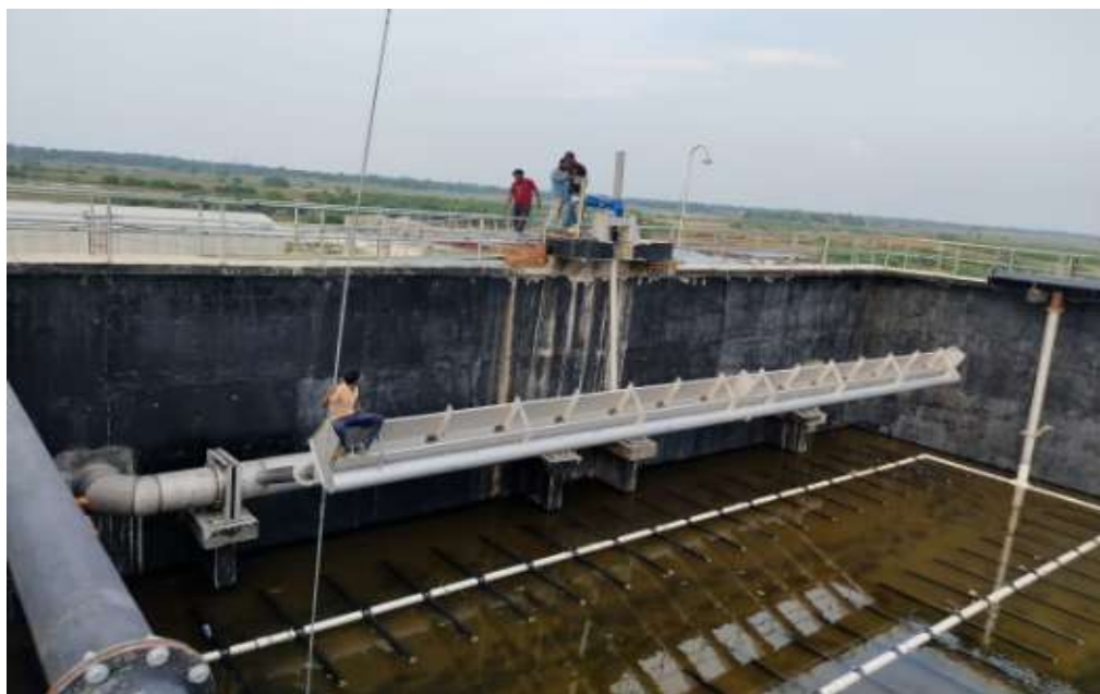
Decanter Installation & Testing
