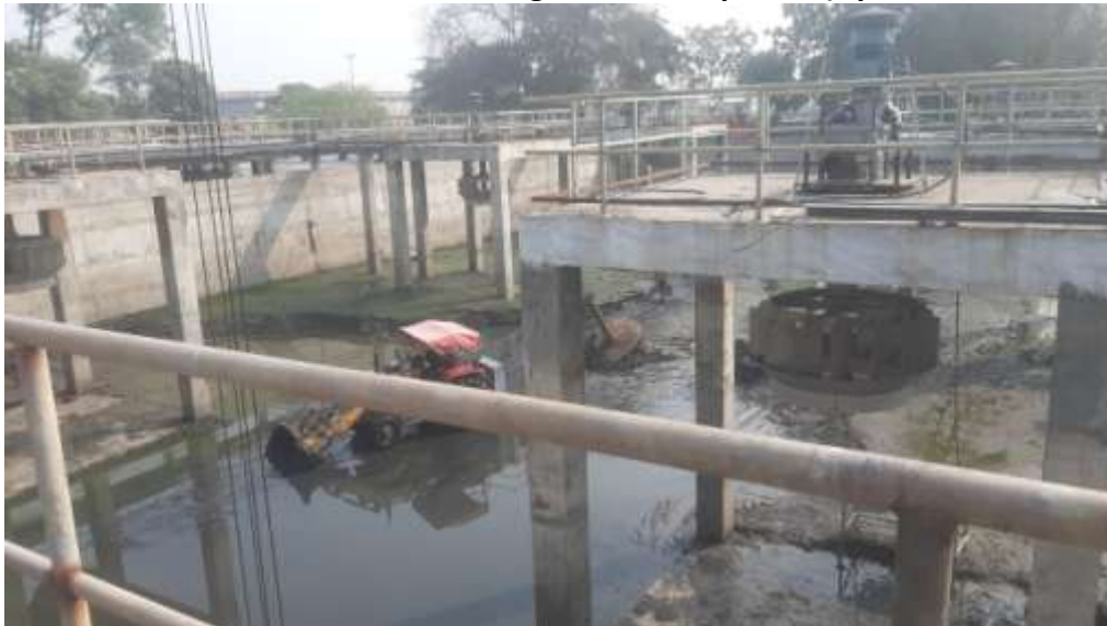
Sludge cleaning work in progress at aeration tank no.2 in January 2023
