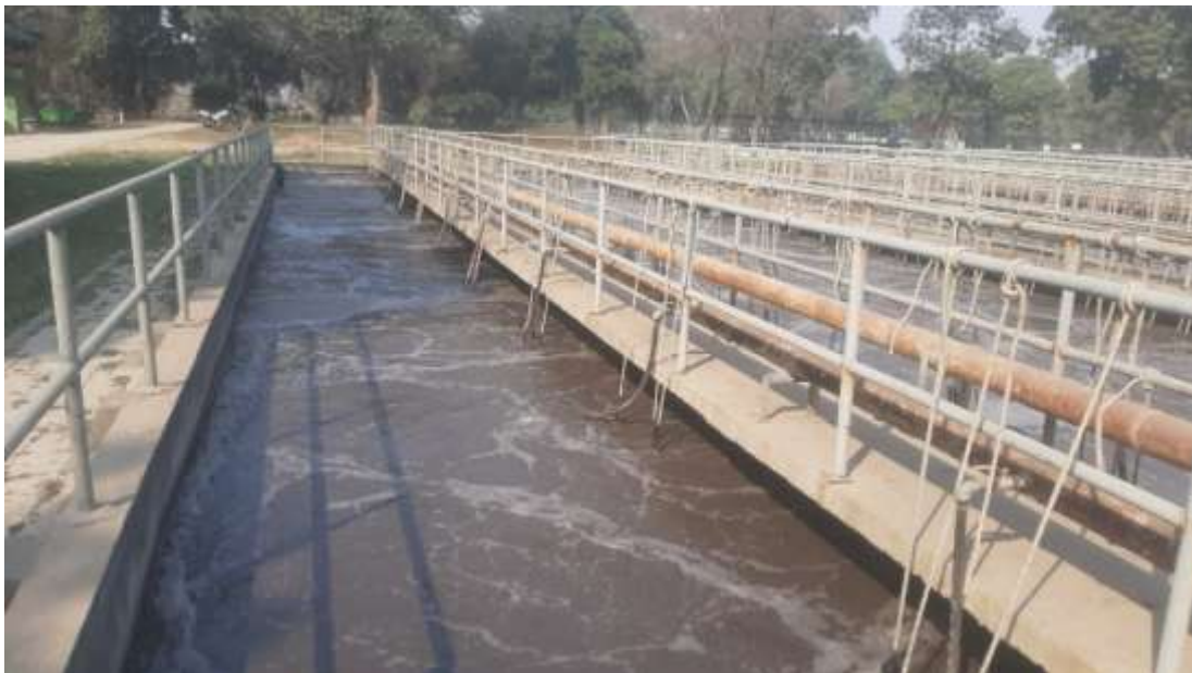
Aeration tank at 43 MLD STP Jajmau
