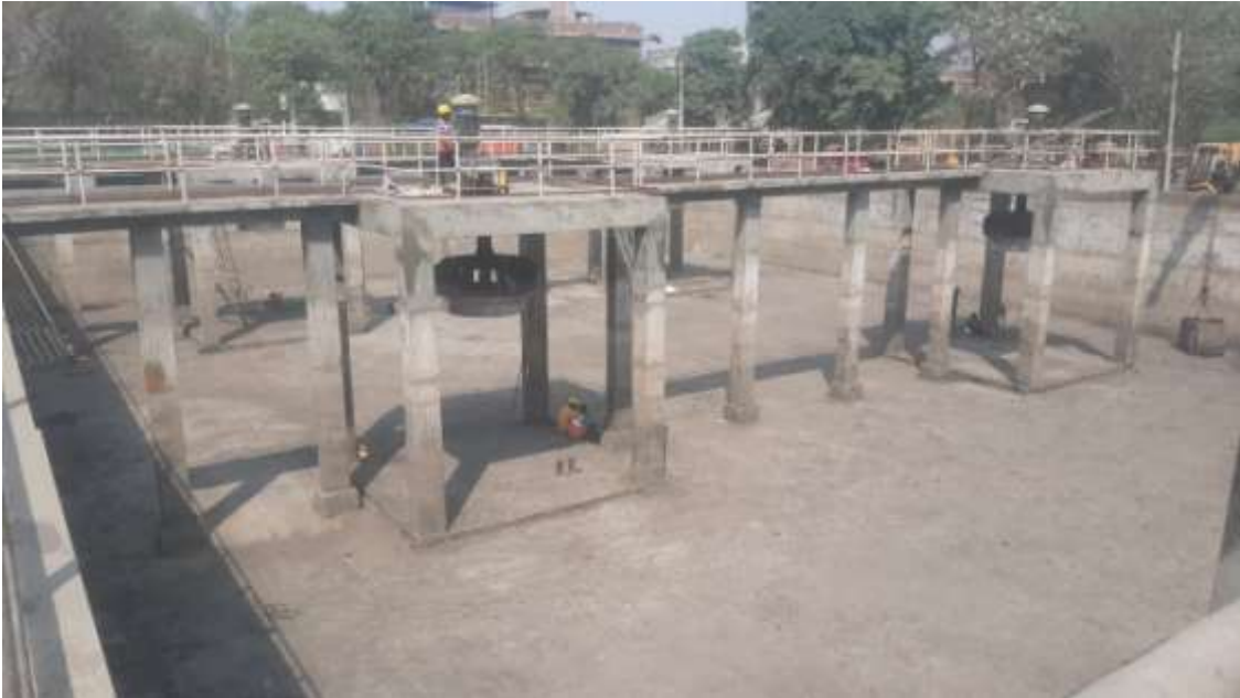
Sludge cleaning work at aeration tank no.1 in February 2023
