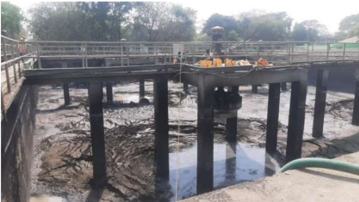
Sludge cleaning work at aeration tank no.3 in February 2023
