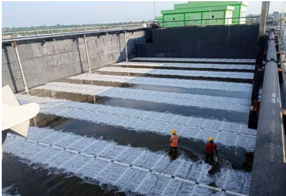
Diffuser leakage testing done
