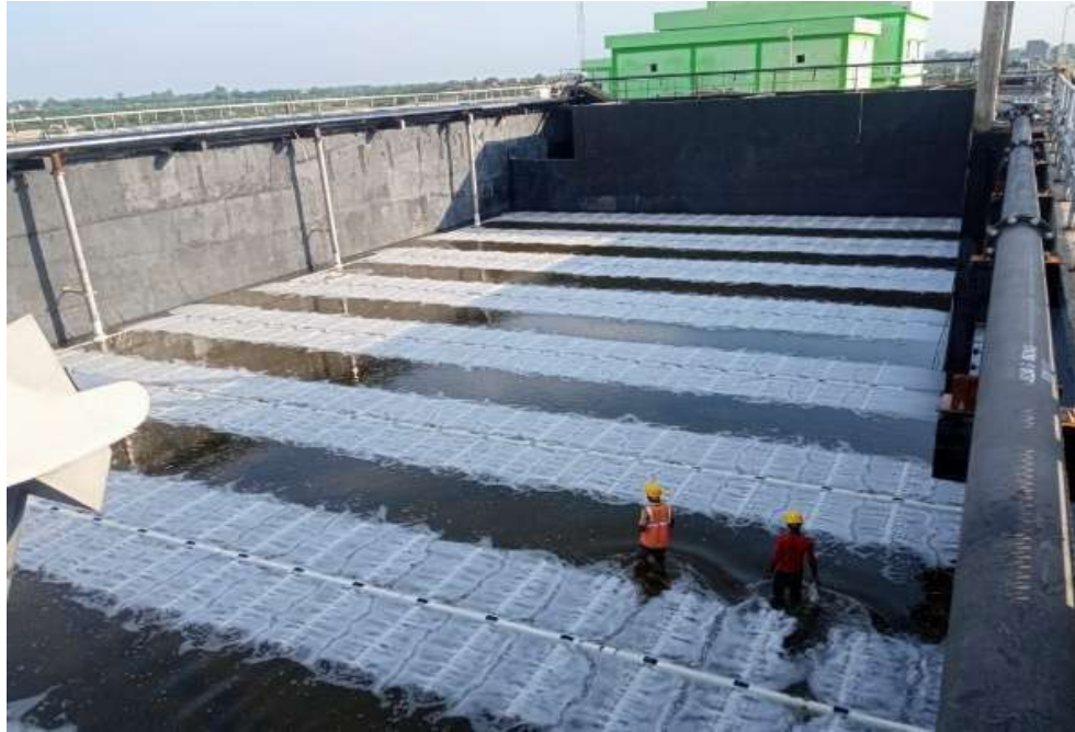
Diffuser leakage testing done
