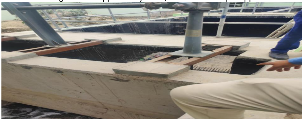
Fig: I&D Sluice Gate
