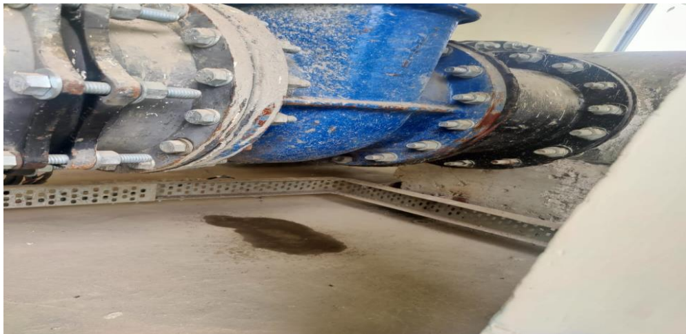
Fig: Leakage found in pipe line.
