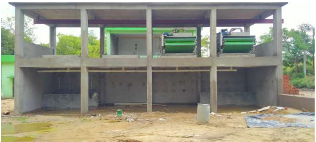
Installation of 2 nos of BFP in progress
