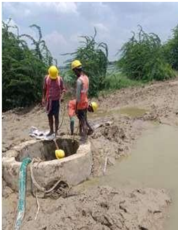
Sewer Line and Manhole Cleaning at MH 37 on 22.08.2023
