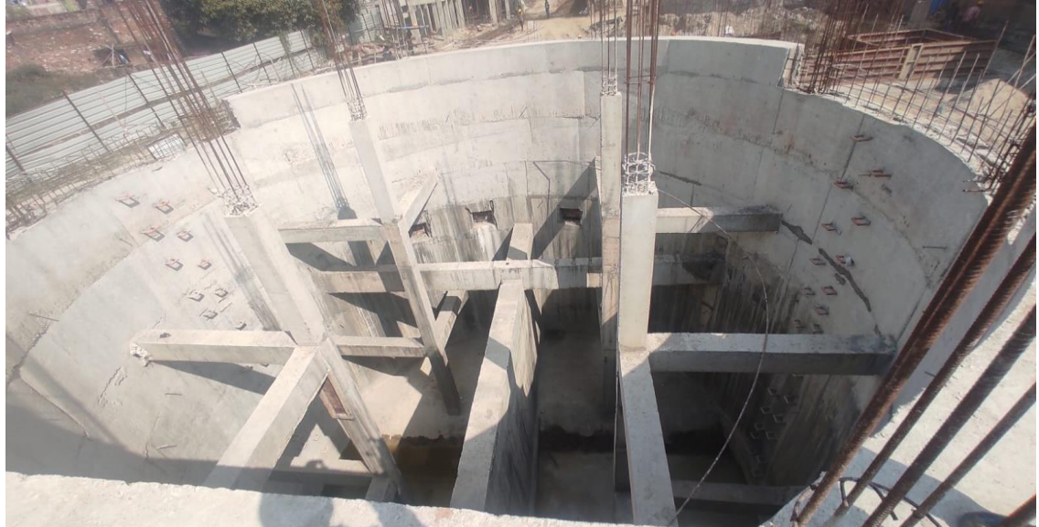
MPS wall casting work done
