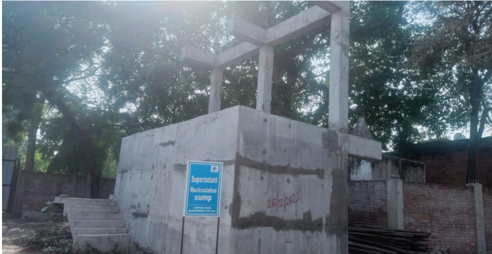
Supernatant Sump, Hydro test pending
