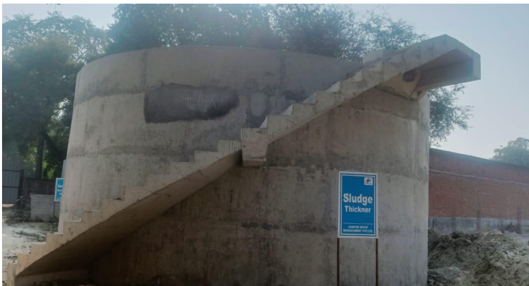
Sludge Thickener, Hydro test pending
