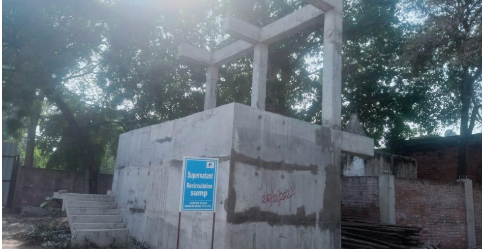
Supernatant Sump, Hydro test pending
