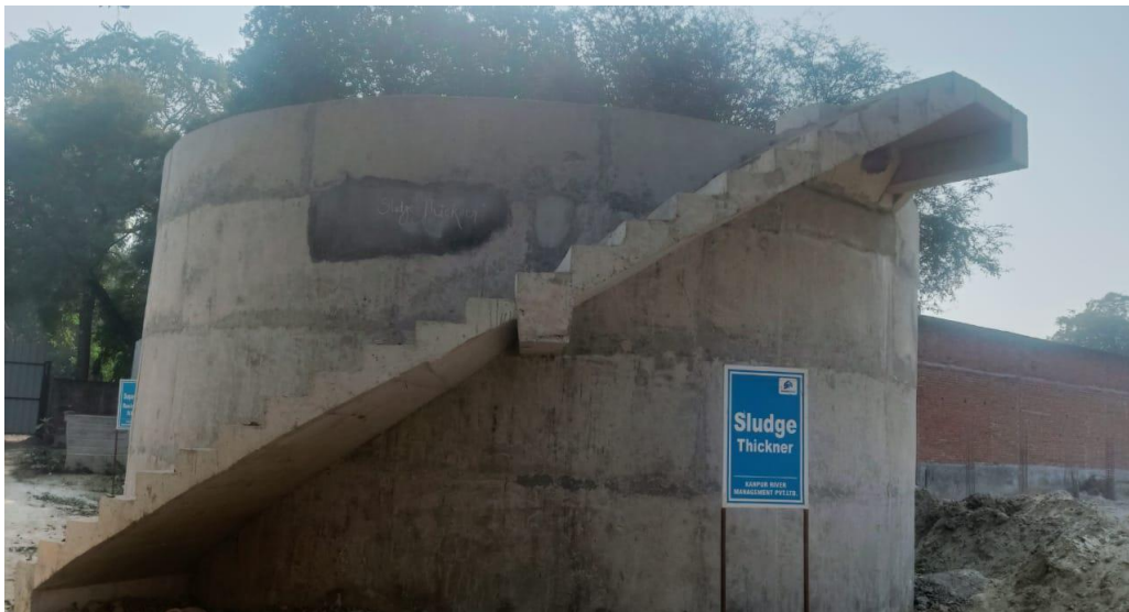
Sludge Thickener, Hydro test pending
