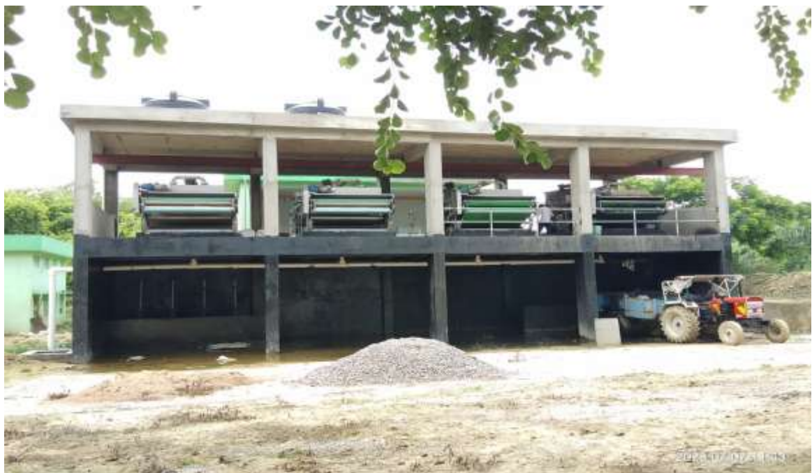
Installation of 2 nos of BFP in progress
