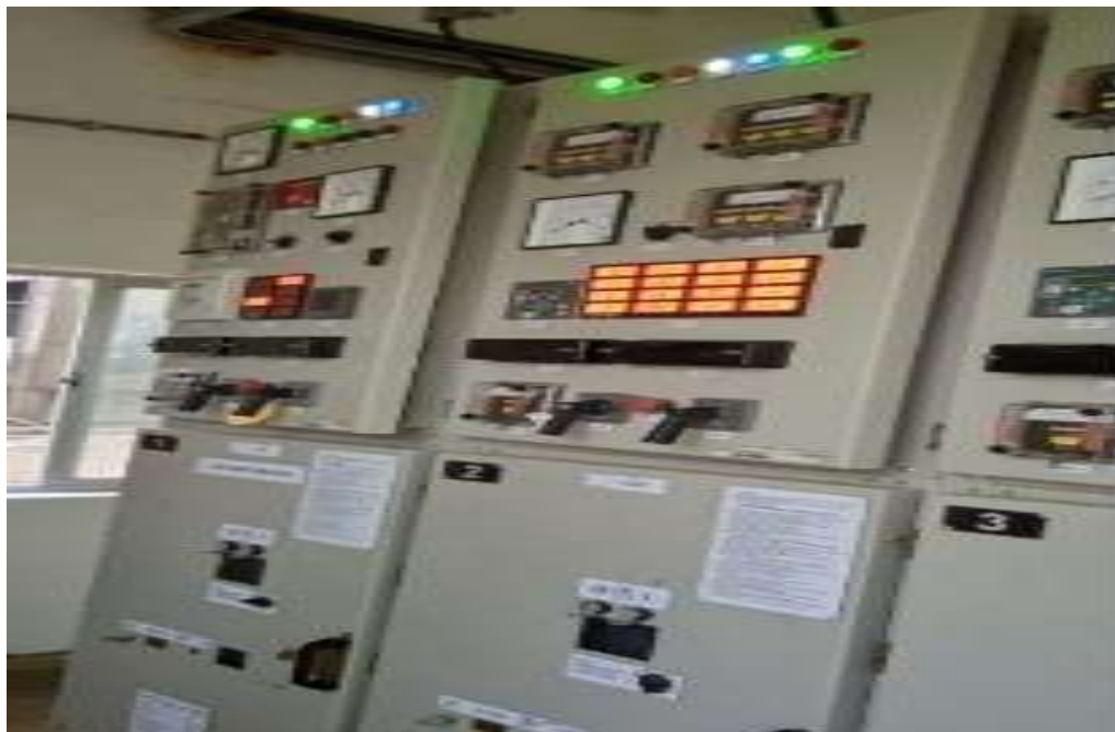
HT VCB Panel testing done
