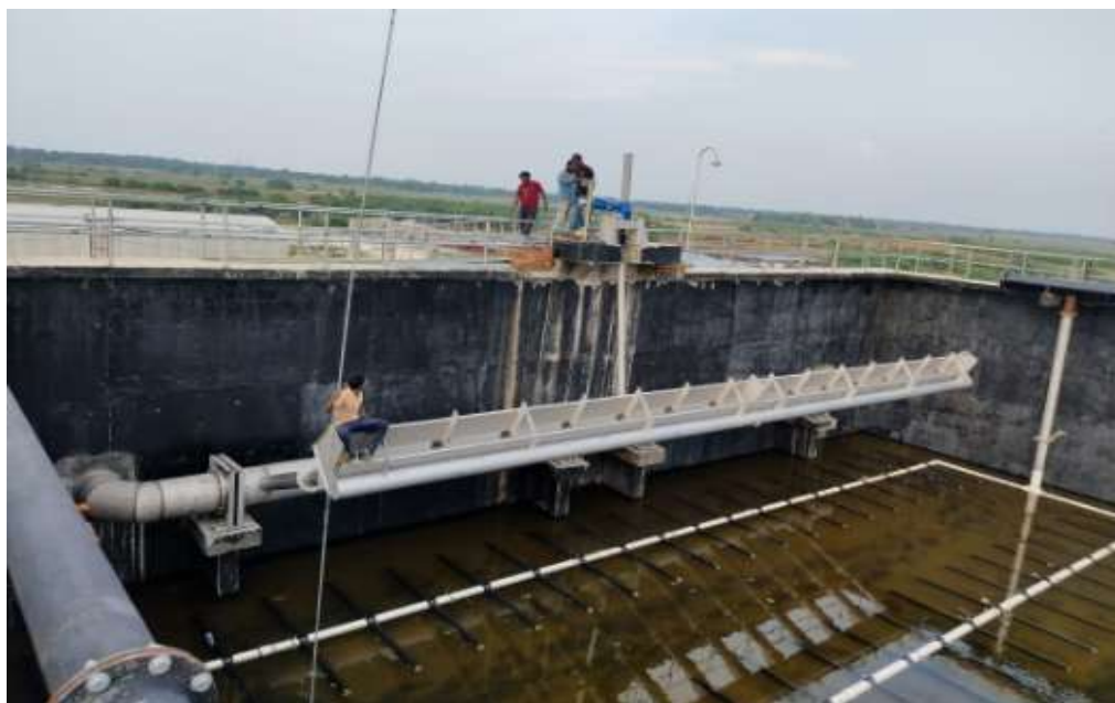
Decanter Installation & Testing
