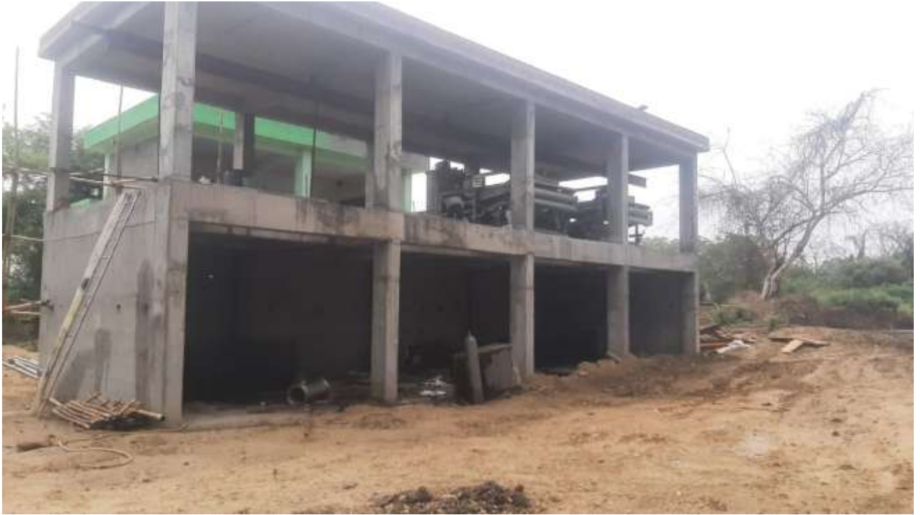
BFP building brick work and finishing work pending on 20.03.2023
