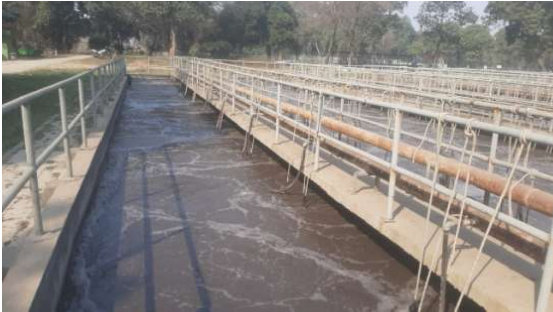
Aeration tank at 43 MLD STP Jajmau
