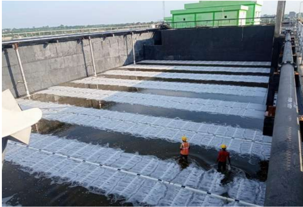
Diffuser leakage testing done
