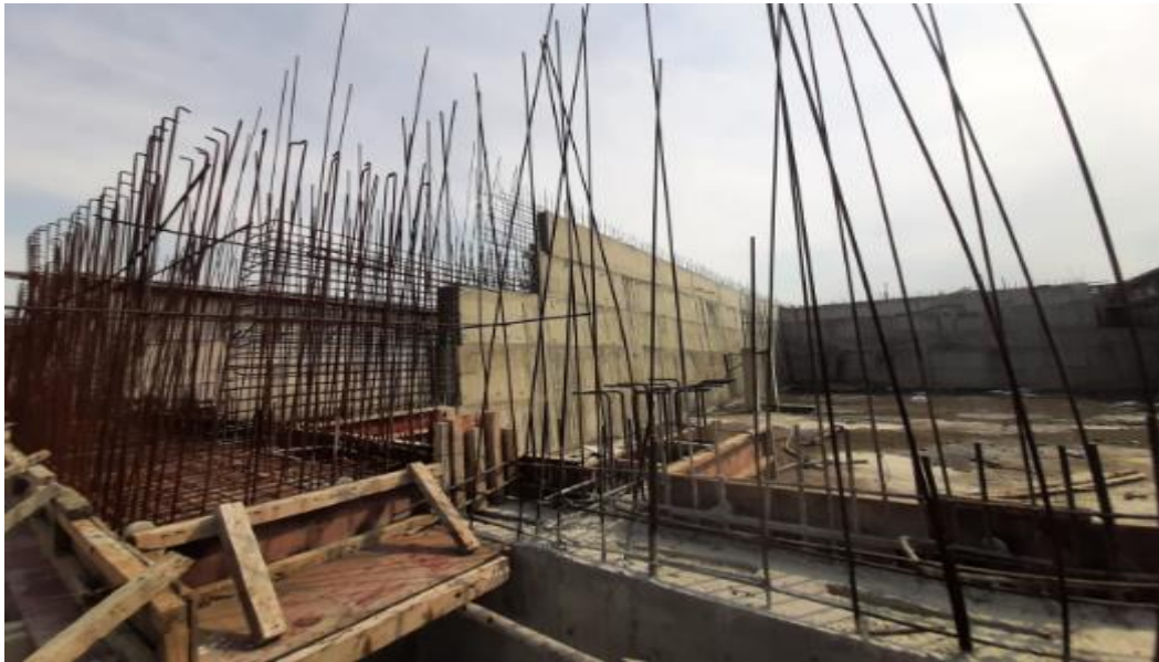
SBR - North side wall, reinforcement and shuttering work in progress
