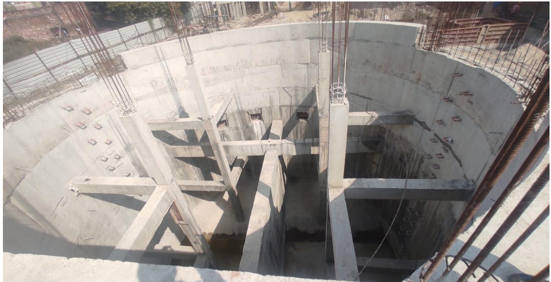
MPS wall casting work done
