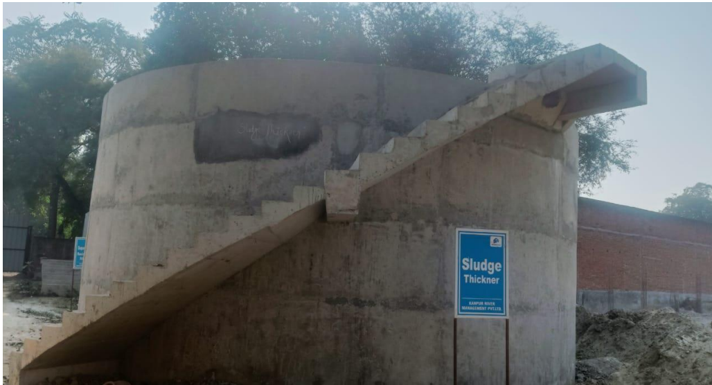
Sludge Thickener, Hydro test pending
