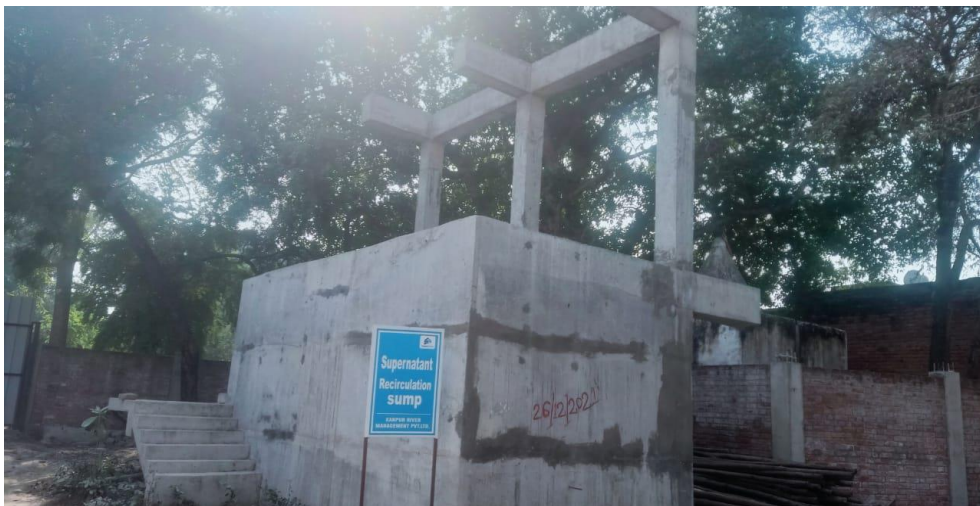
Supernatant Sump, Hydro test pending
