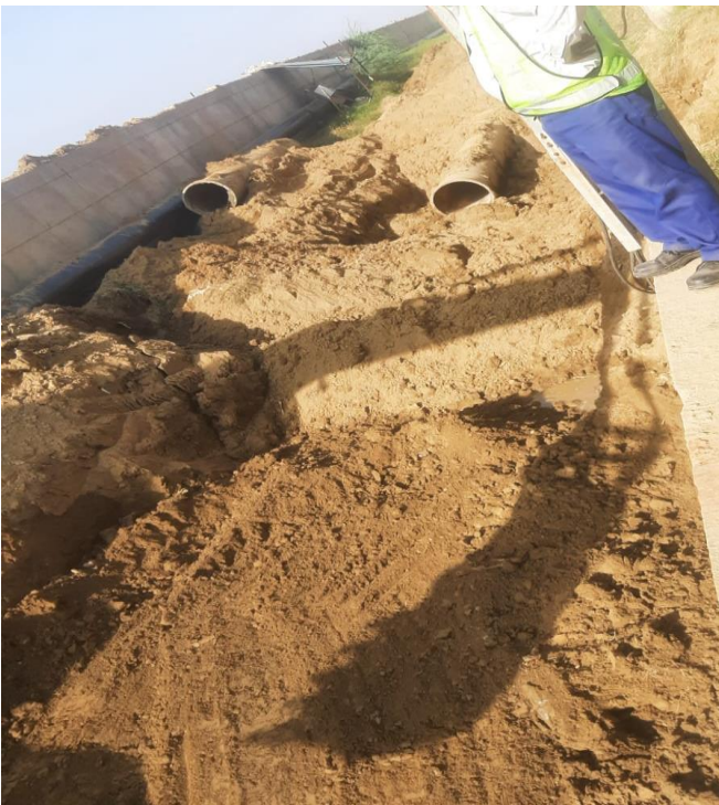
Installation of pipe 1200 mm from MPS to PTU
