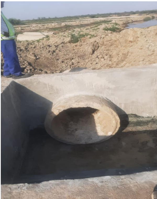
Incoming Chamber at source at City jail Naala outside and inside
