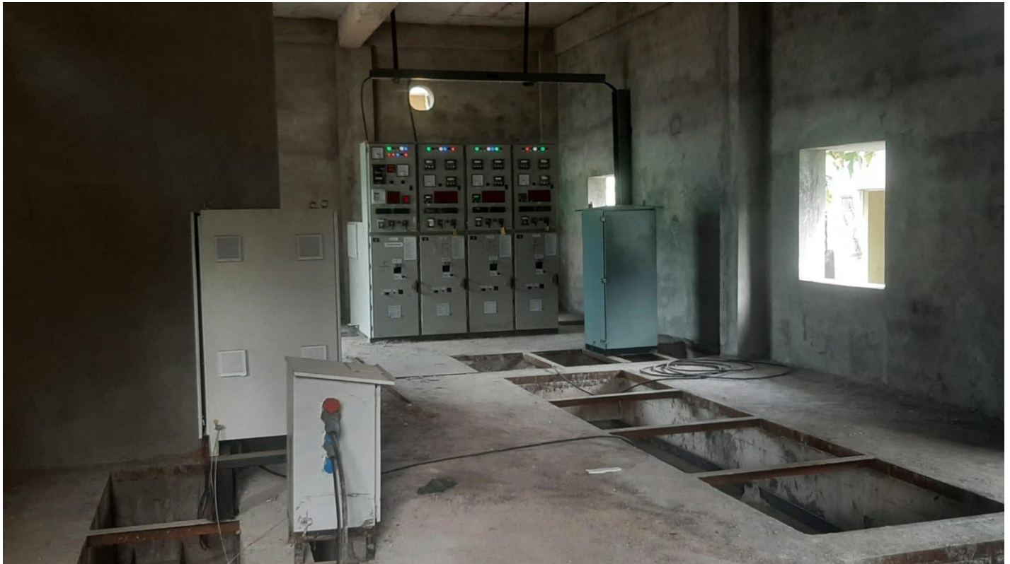
Installation of HT Panel in the panel room
