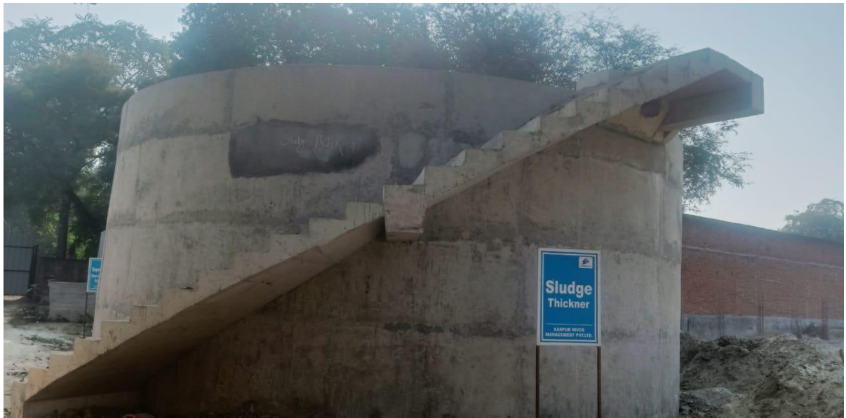
Sludge Thickener, Hydro test pending
