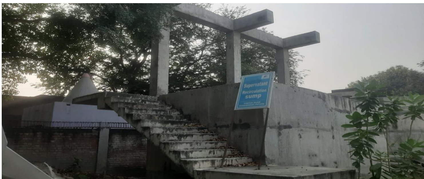
Supernatant Sump, Hydro test pending
