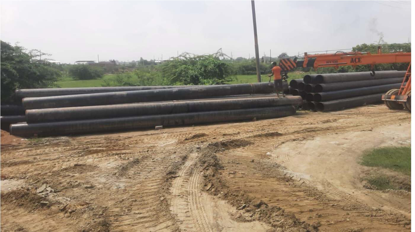
PIC-5- Stacking of 500 mm dia MS pipes for laying
