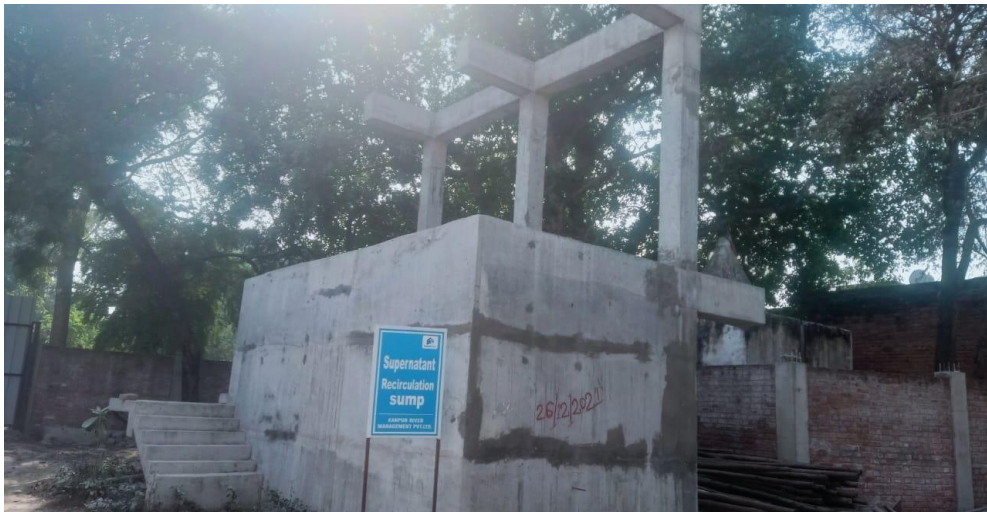
Supernatant Sump, Hydro test pending
