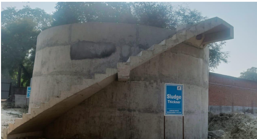
Sludge Thickener, Hydro test pending
