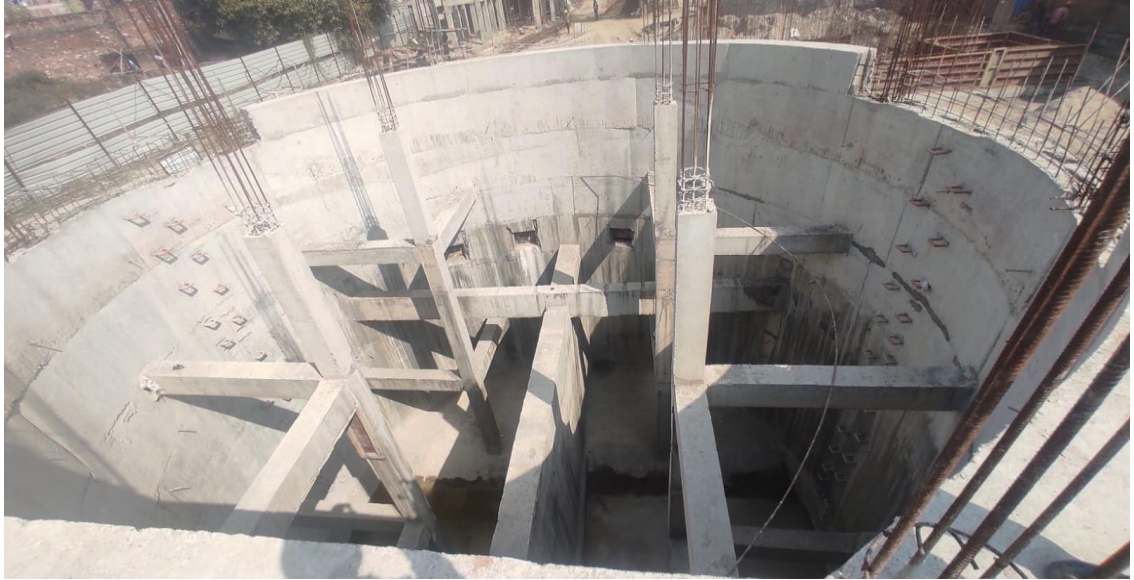
MPS wall casting work done
