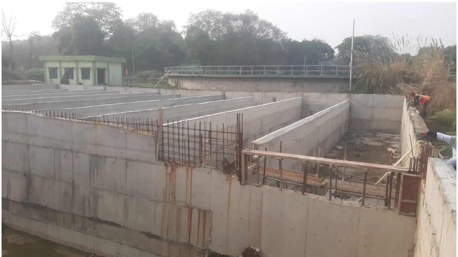
Chlorine Contact Tank
