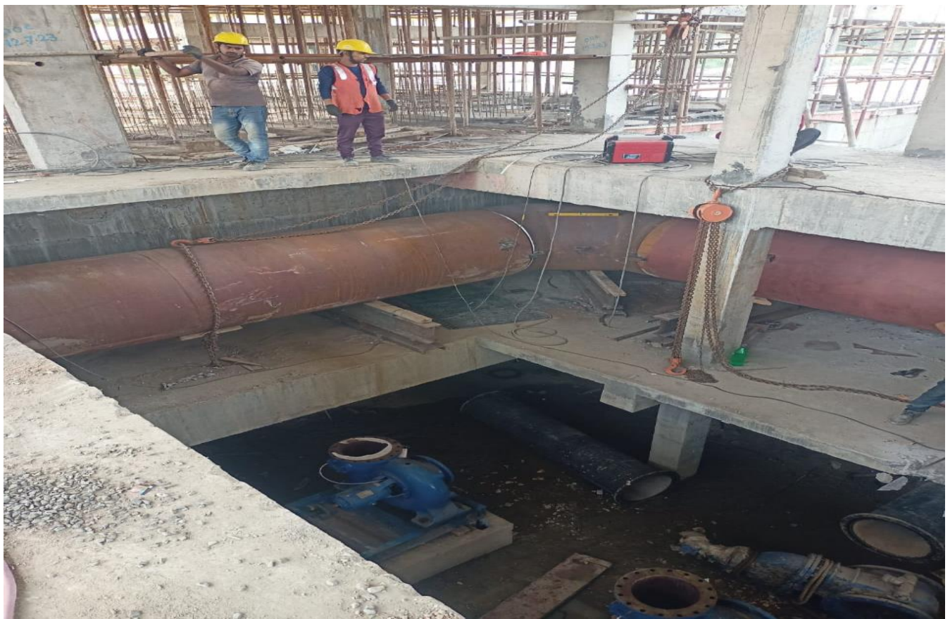
Common header connection in TEPH
