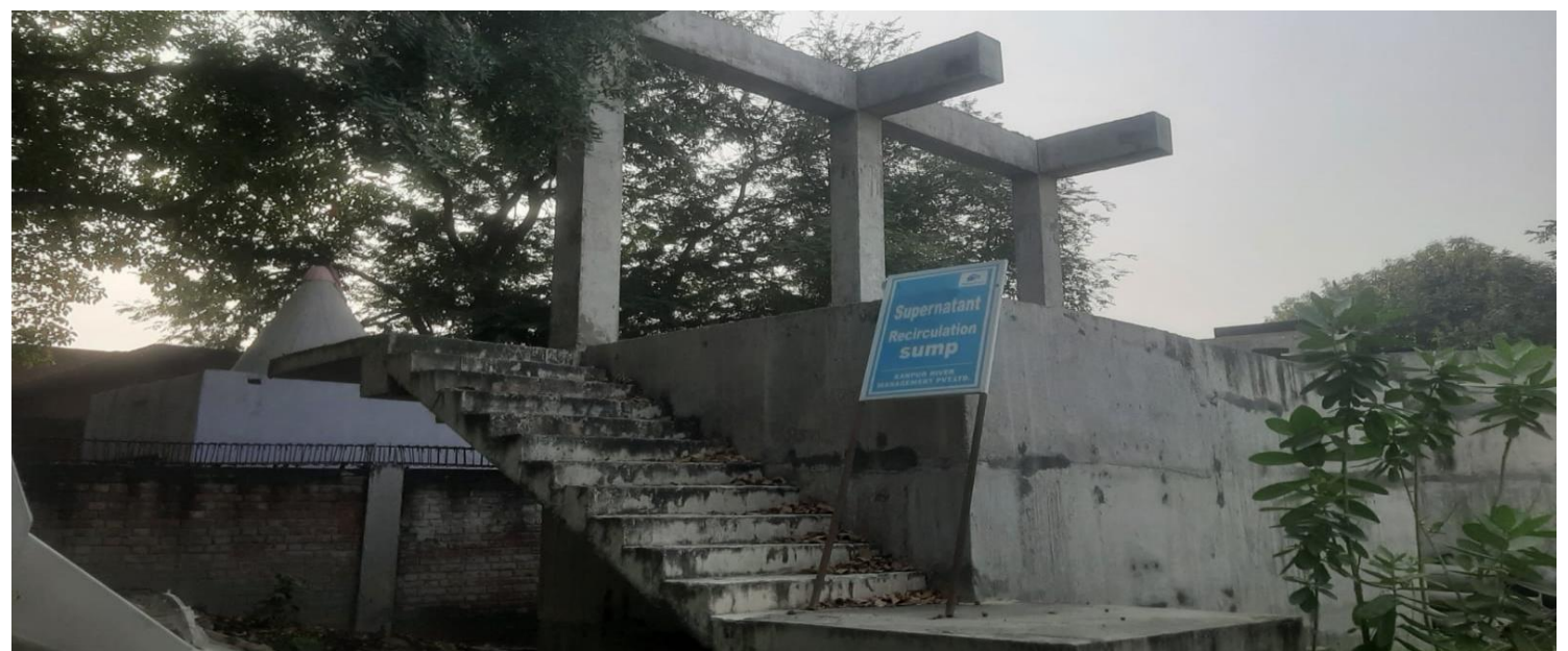
Supernatant Sump, Hydro test pending
