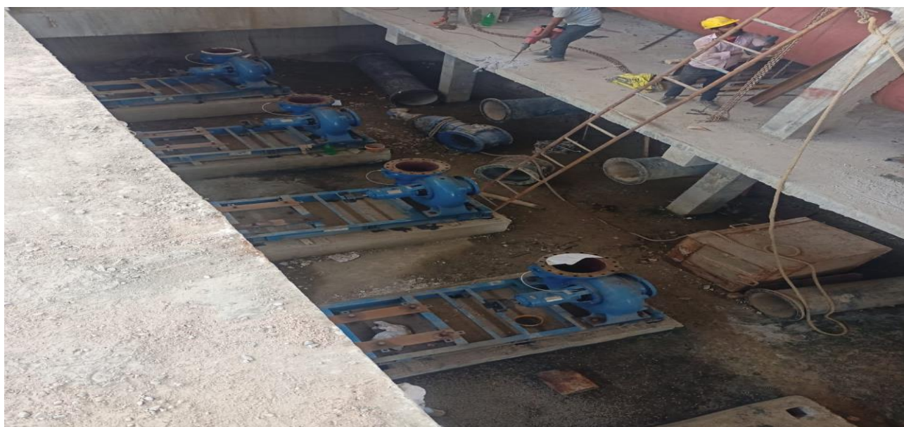
Base plate and Pump Installation at TEPH
