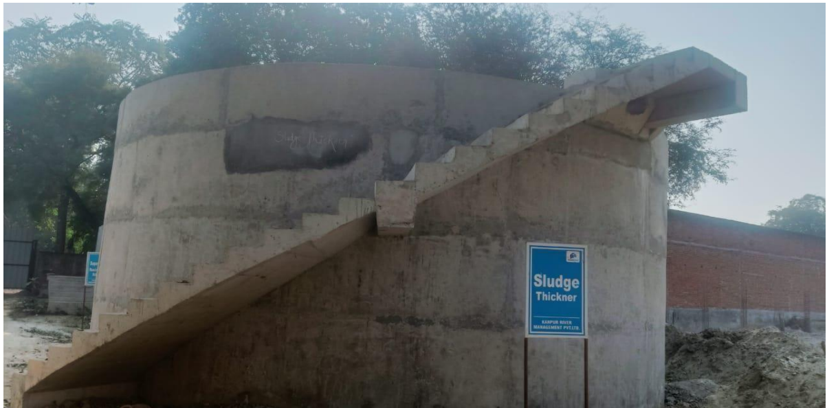
Sludge Thickener, Hydrotest pending
