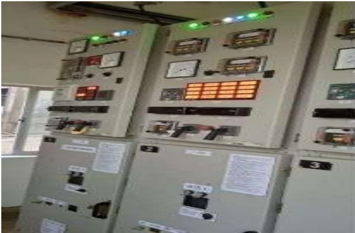
HT VCB Panel testing done
