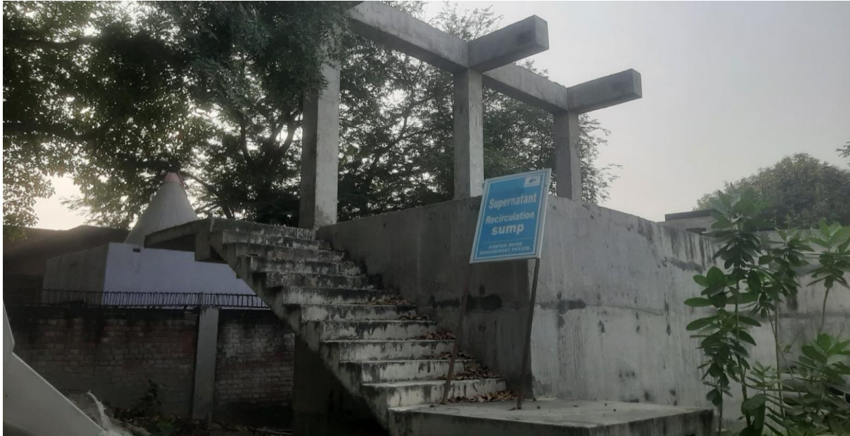
Supernatant Sump, Hydro test pending
