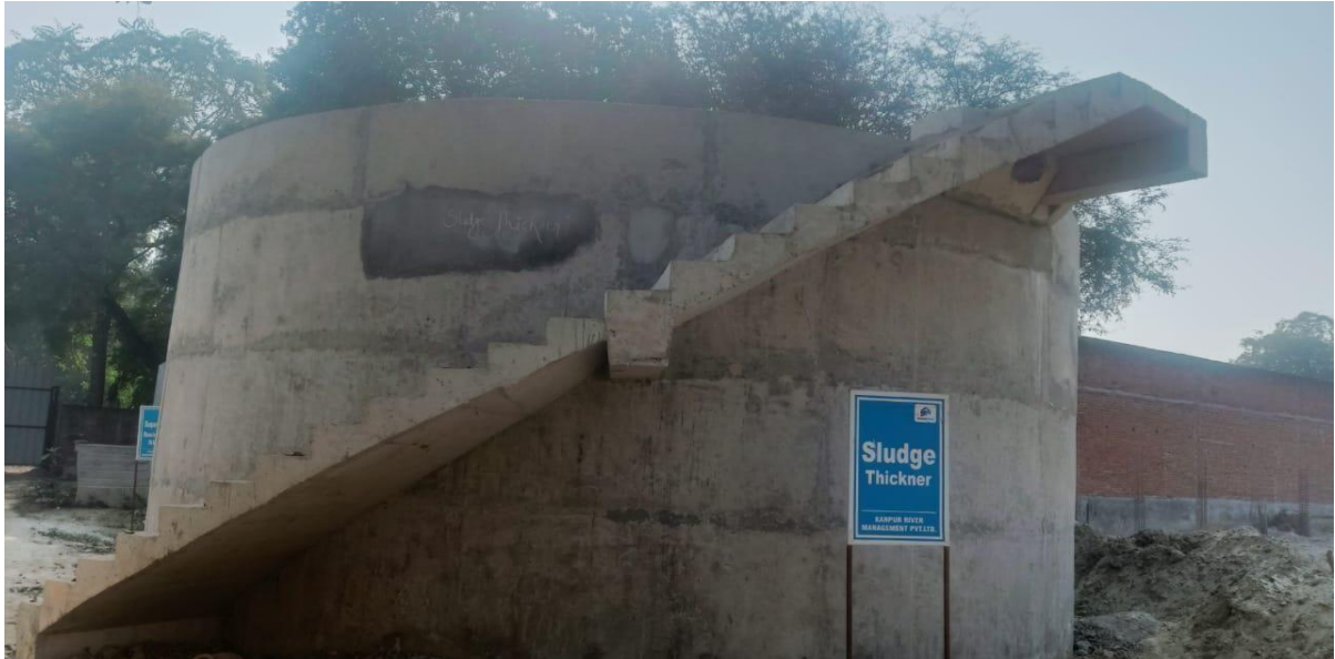
Sludge Thickener, Hydro test pending
