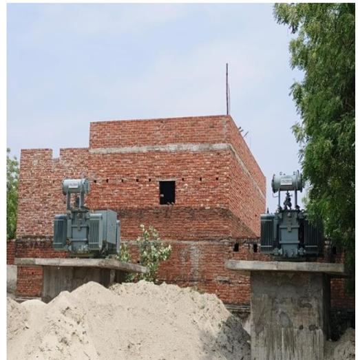
**I. CCT & Chlorination building** - In CCT outlet channel work, finishing of outlet chamber, grinding, finishing and painting works are pending. In building foundation of tonner, Electric work, plumbing, floor, finishing and painting works are pending. Booster pump and fitting pump can be install. During inspection there is no manpower on chlorination building & CCT.
