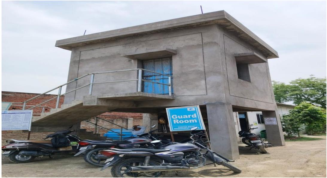
**H. Transformer & DG Yard-** Staircase, finishing, approach and painting works are pending.
