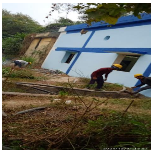
Cable route excavation
