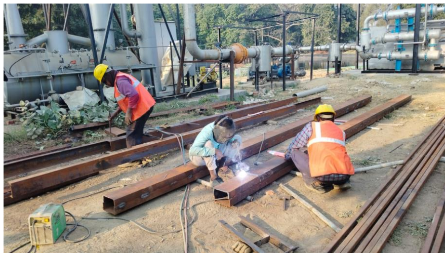
Scaffolding shade structure work
