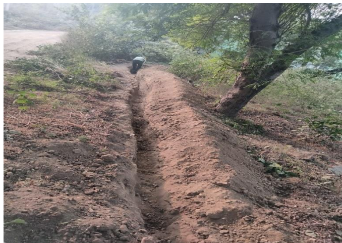
Cable route excavation
