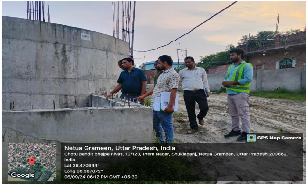
c PTU- Most of Steel found corroded. PTU, Column work completed and slab shuttering and reinforcement work is in progress. In Inlet chamber area finishing work, hydro test is pending. In Grit chamber and parshall flume RCC wall & slab, walk way, platform and hydro test pending. Stair costing done and connecting channel column on progress.
