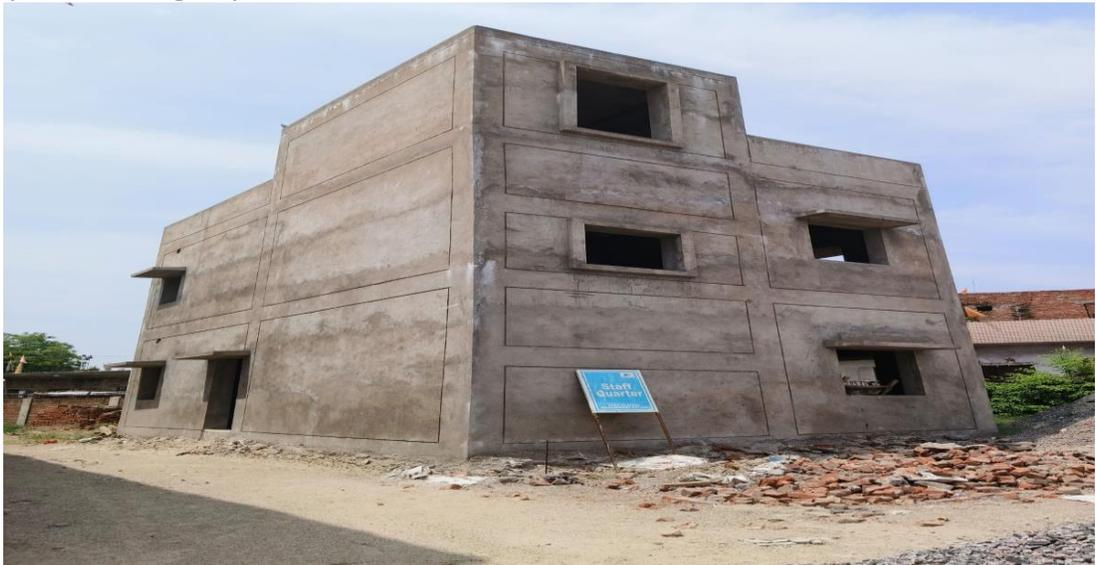
**D. Guard Room-** Electric work, plumbing, sanitary fittings, floor, roof treatment, drainage, finishing and painting works are pending. There is no manpower on staff quarter during inspection.
