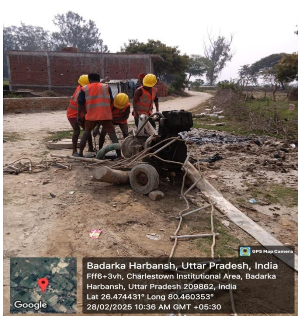
Desilting work at MH-14 & Jointing work
