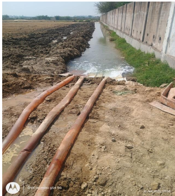
Bore well 140 is in progress and MH 38 depressing water work in progress
