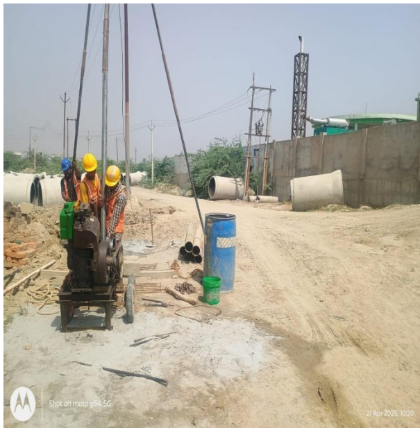
Bore well 140 is in progress and MH 38 depressing water work in progress
