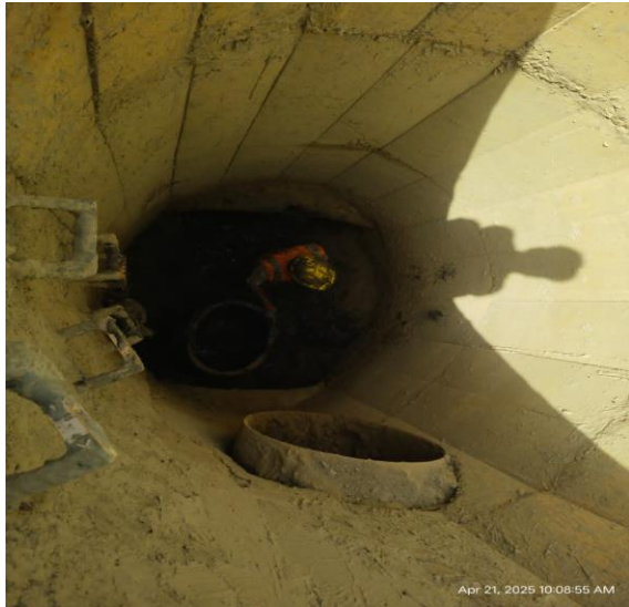
Desilting work for MH 17 to 19 and 16 to 17
