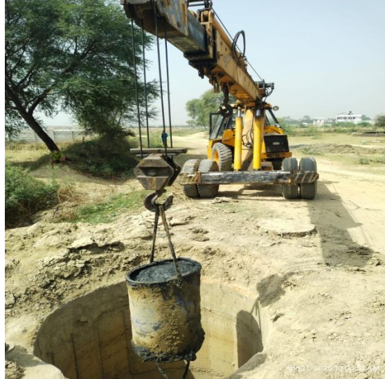
Desilting work for MH 17 to 19 and 16 to 17
