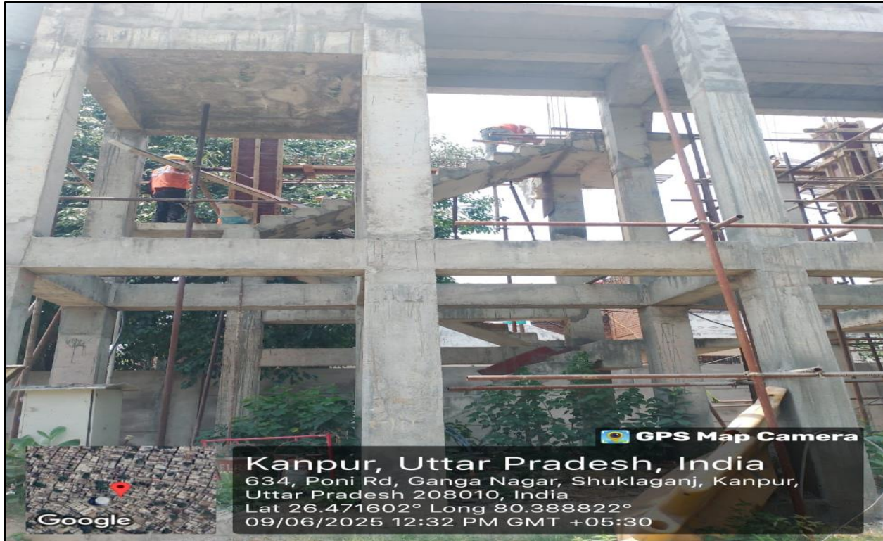
PTU Staircase & walkway reinforcement & Shuttering work.
